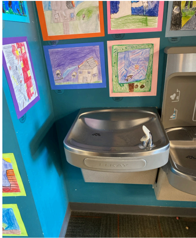
3/18/2024 - 650-1 - Epic Elementary - 001868- Hallway by North Office-Left
