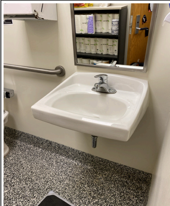
3/18/2024 - 650-35 - Epic Elementary - 001882- Room 302-Restroom
