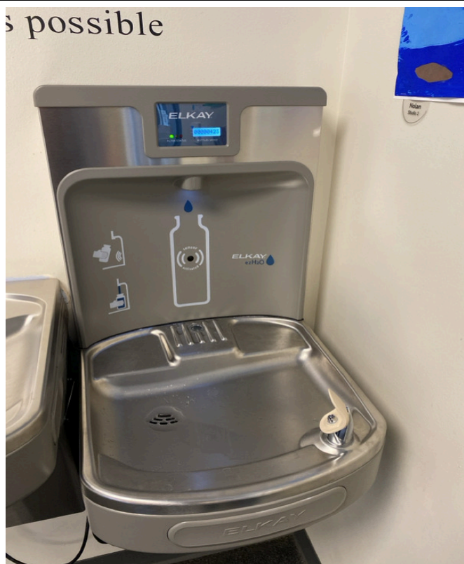
3/18/2024 - 650-21 - Epic Elementary - 001869F- South Entrance
