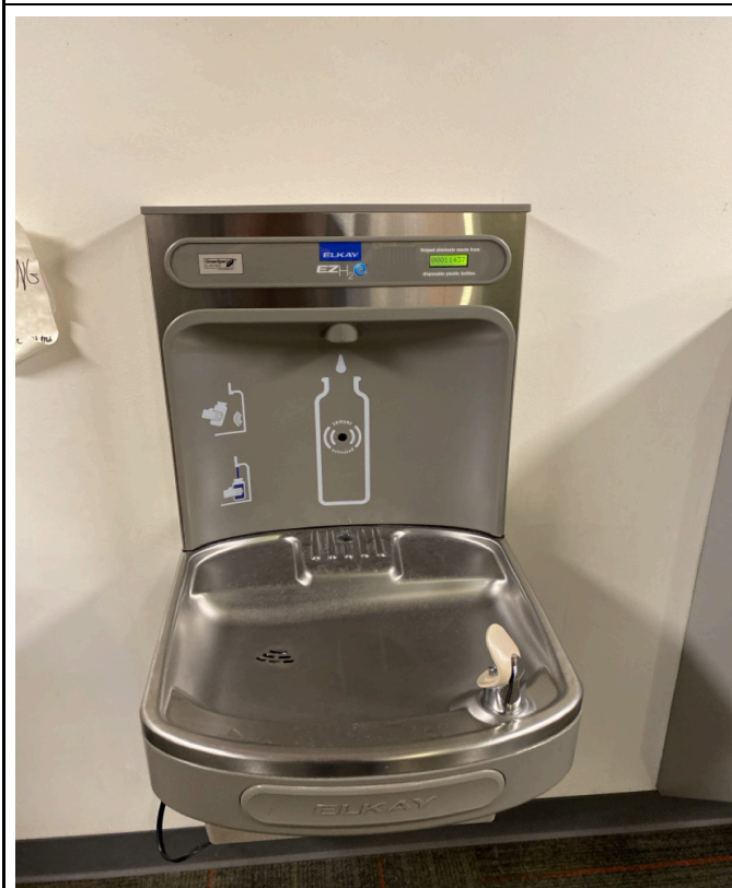
3/18/2024 - 650-31 - Epic Elementary - 001878F- Hallway by 304
