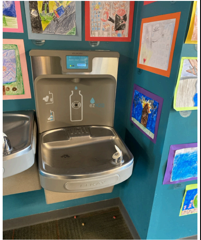
3/18/2024 - 650-2 - Epic Elementary - 001868- Hallway by North Office-Right
