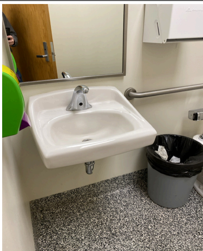
3/18/2024 - 650-36 - Epic Elementary - 001883- Room 300-Restroom
