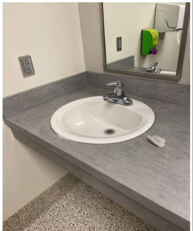
3/18/2024 - 650-16 - Epic Elementary - 001894-By 202-Girl's Restroom-Left
