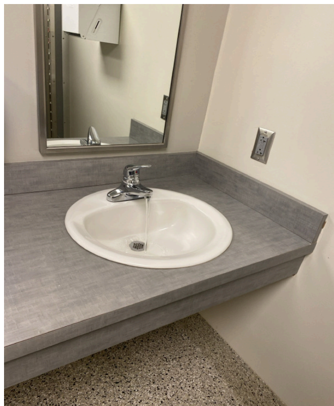
3/18/2024 - 650-15 - Epic Elementary - 001893-By 202-Boy's Restroom-Right
