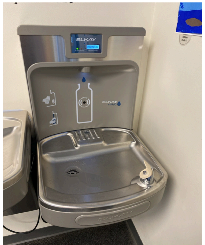
3/18/2024 - 650-20 - Epic Elementary - 001869B- South Entrance-Right
