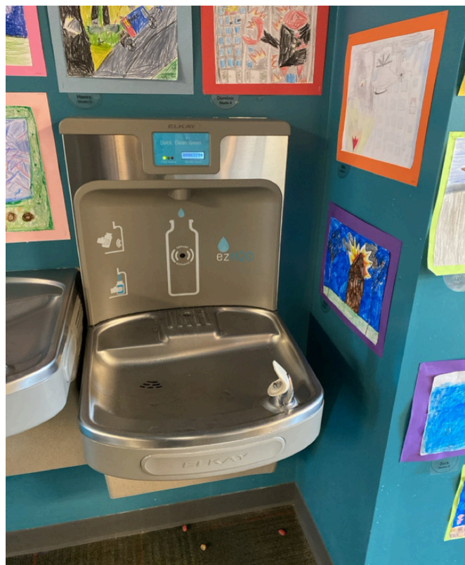
3/18/2024 - 650-3 - Epic Elementary - 001868F- Hallway by North Office
