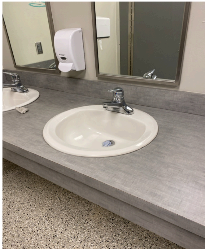
3/18/2024 - 650-17 - Epic Elementary - 001895-By 202-Girl's Restroom-Middle
