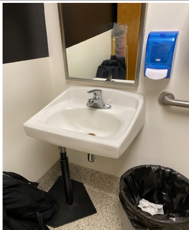
3/18/2024 - 650-22 - Epic Elementary - 001870- Staff Restroom by Custodial Office-Left
