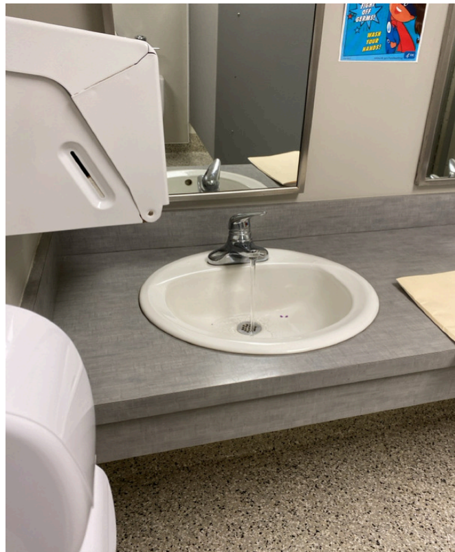
3/18/2024 - 650-13 - Epic Elementary - 001891-By 202-Boy's Restroom-Left
