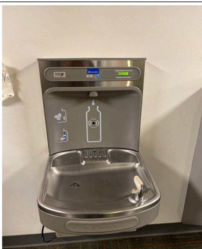
3/18/2024 - 650-30 - Epic Elementary - 001878B- Hallway by 304
