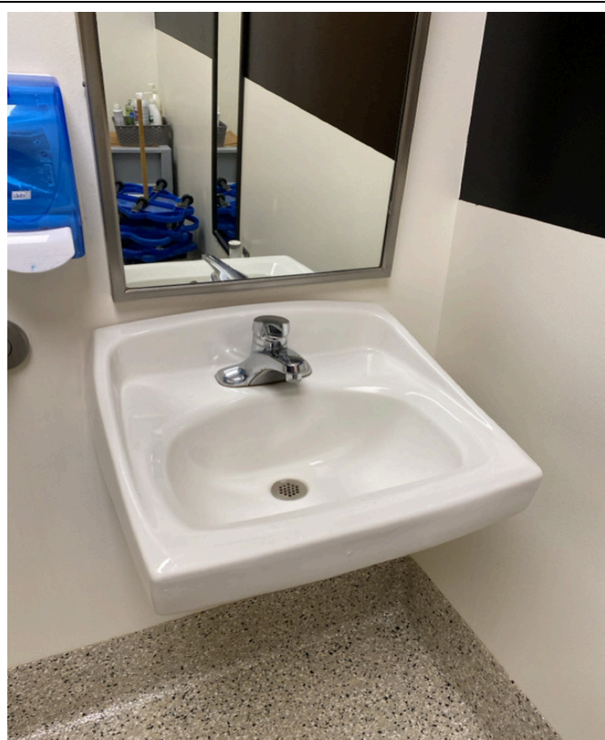
3/18/2024 - 650-23 - Epic Elementary - 001871- Staff Restroom by Custodial Office-Right
