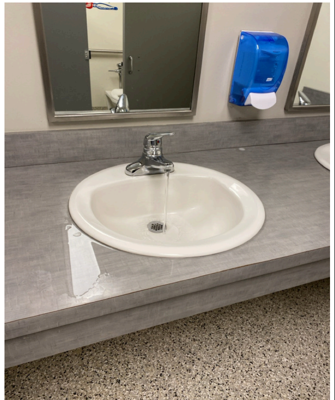
3/18/2024 - 650-14 - Epic Elementary - 001892-By 202-Boy's Restroom-Middle
