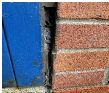
Electrical Room Door Caulking
