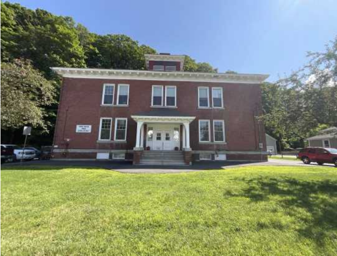
1 - OVERVIEW OF FRONT ELEVATION
