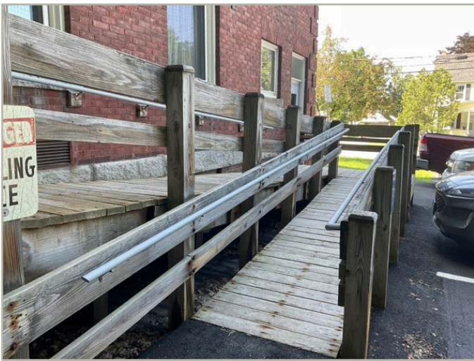
3 - EXT RAMP or PRIMARY PATH OF TRAVEL
