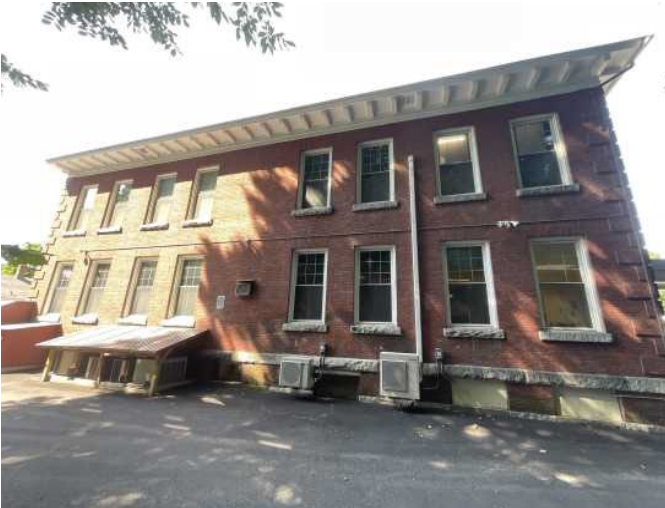
3 - OVERVIEW OF REAR ELEVATION
