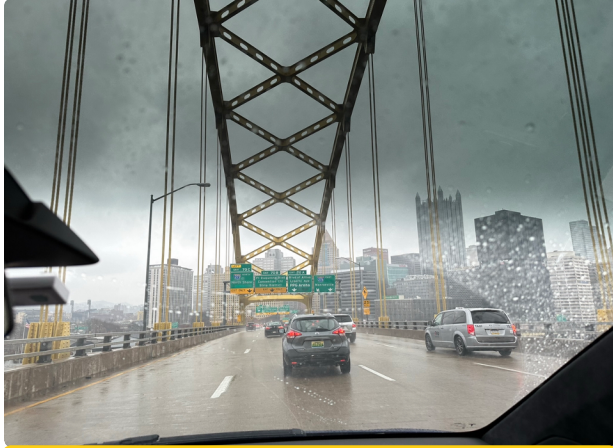
Fort Pitt Bridge
