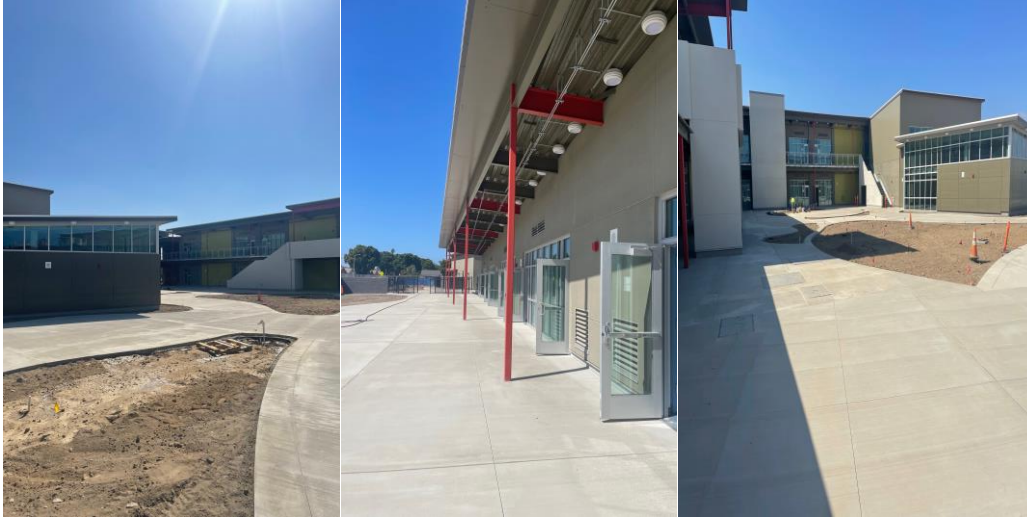
Rose Avenue Elementary School Construction Progress
