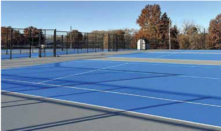
A total of eight tennis courts on the southwest corner of Liberty High School were completed in November 2023. These courts will not only serve the boys and girls tennis teams at LHS, but also provide additional court opportunities for our community.
