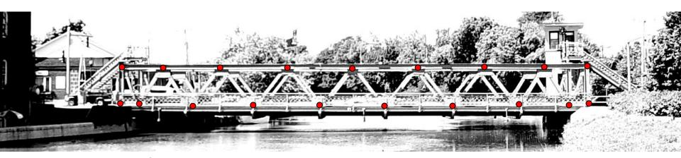
Each side of the main street bridge in Brockport, NY has 19 joints, 35 members, and three reaction forces (pin and roller), making it a statically determinate truss.
