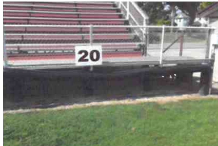
Exposed bleacher structure
