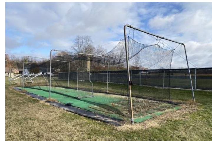
Heavily worn and damaged batting cages
