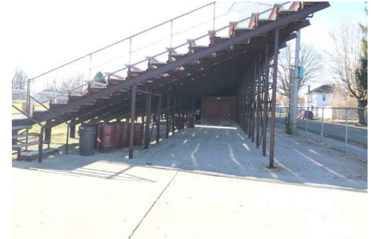
Home side bleacher underside
