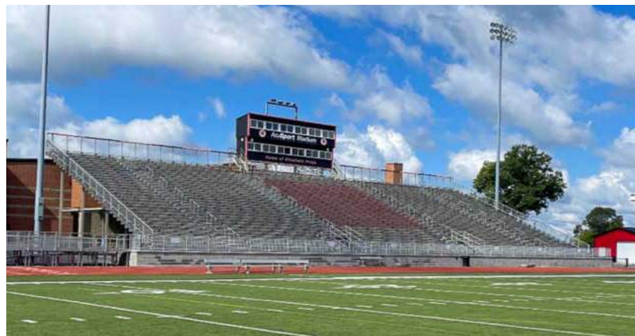
Home Bleachers - South End
