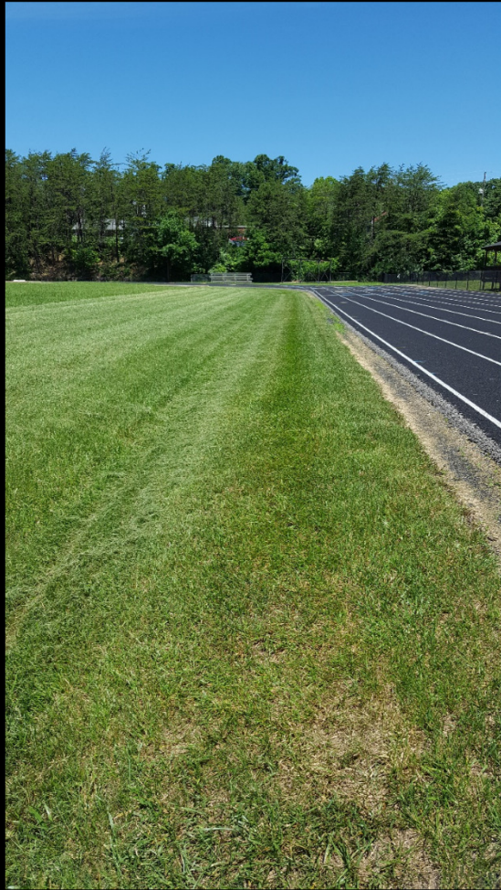
01. Large Drainage Ditch
