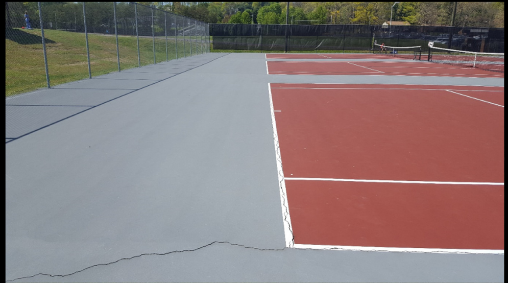
02. Surface Cracks
