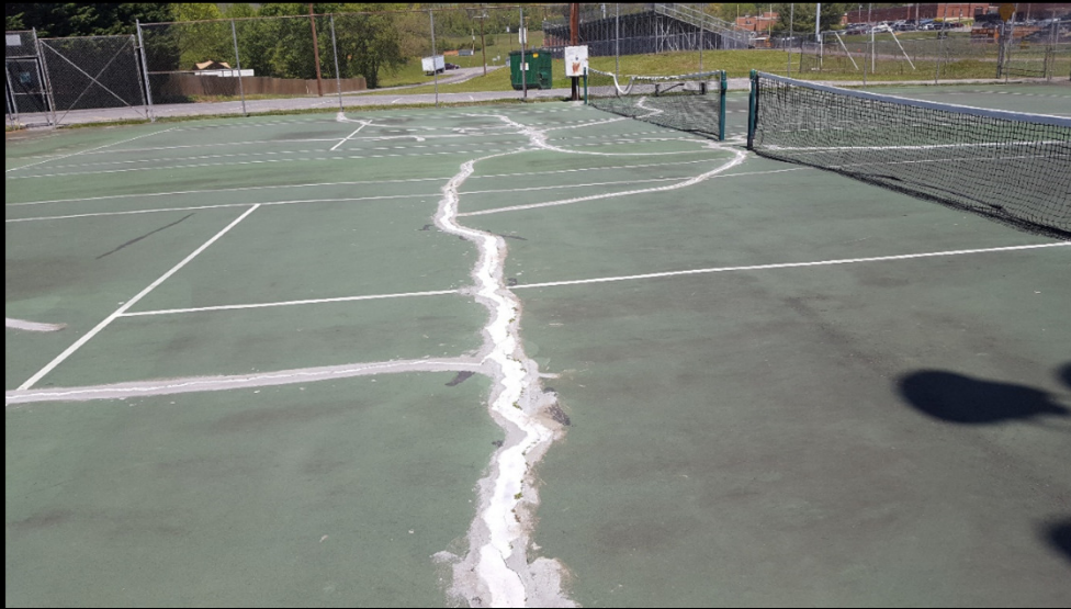
03. Cracks and Nets
