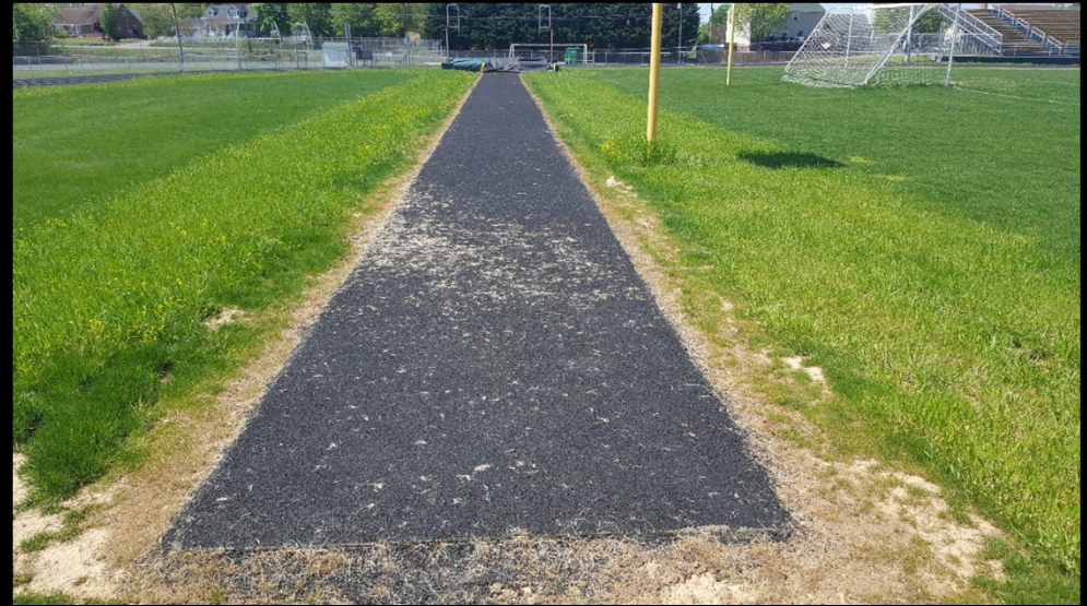
02. Debris on Surface
