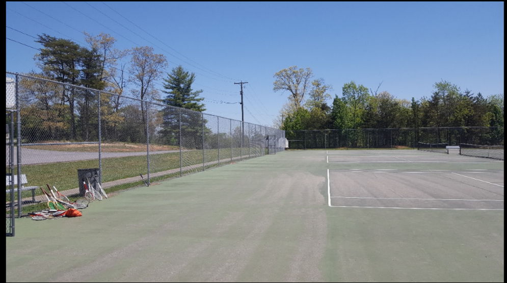
04. Fence in Good Condition
