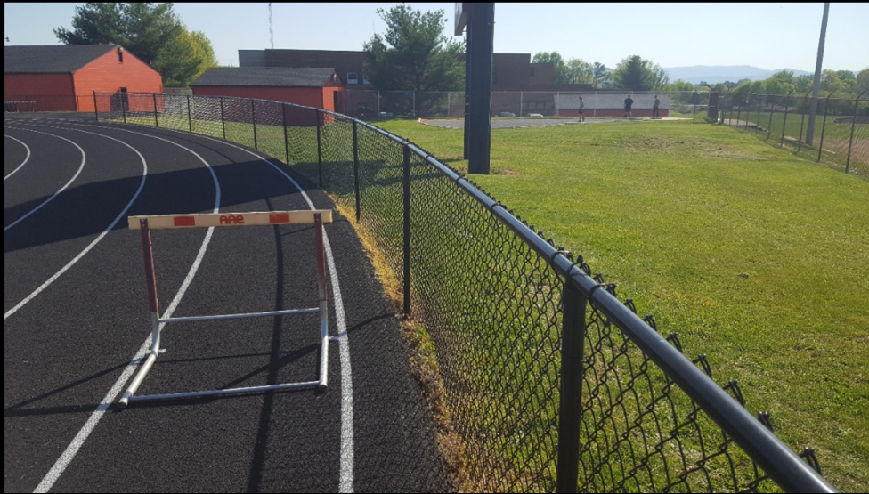
01. Fence Too Close to Track
