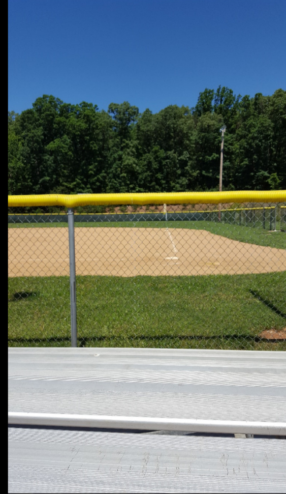
02. Install Taller Fence in Front of Bleachers
