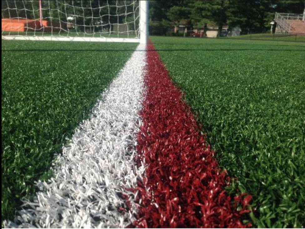
01. Fibers Standing Up in Good Condition
