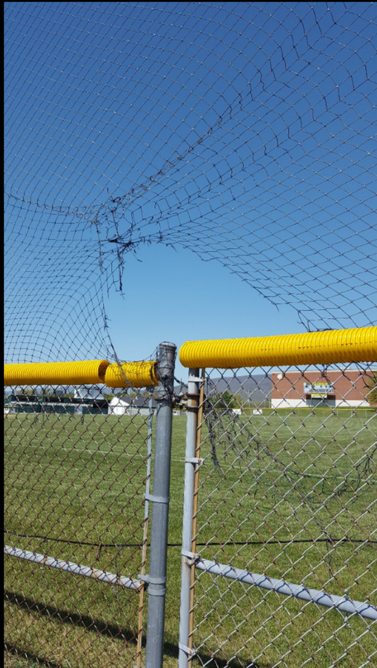
01. Safety Netting Along Right Field
