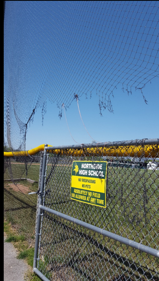
02. Safety Netting Along Right Field
