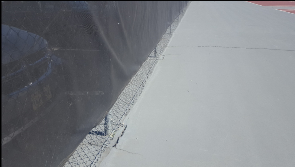
05. Perimeter Fence Foundation
