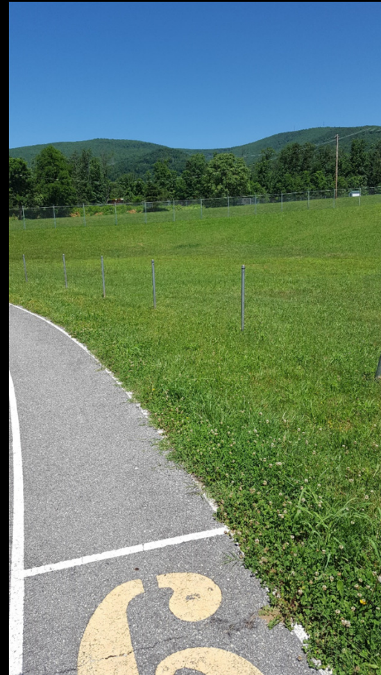
06. No Fabric on Perimeter Fence
