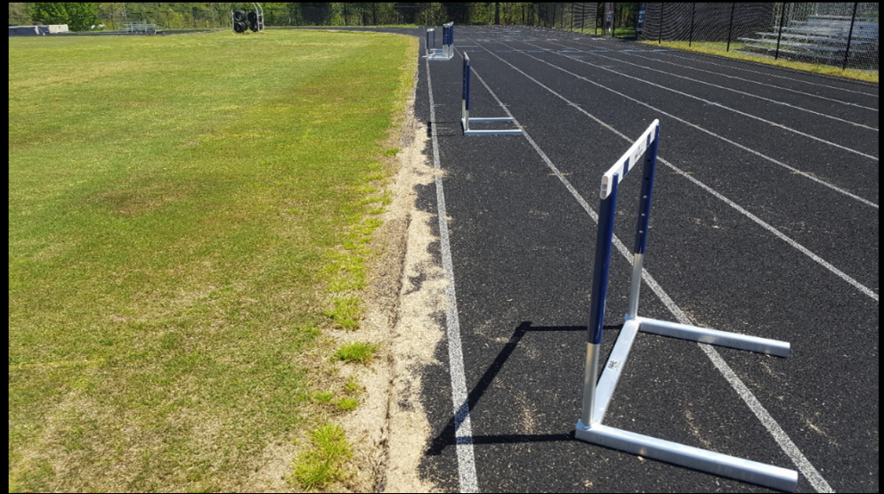
04. Inside Edge No Curb or Trench Drain
