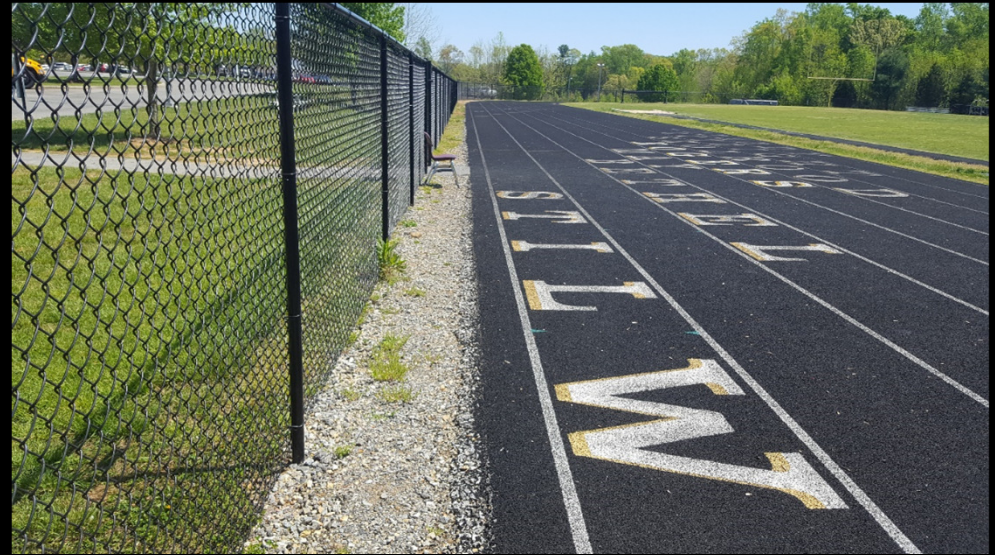
02. No Outside Curbing
