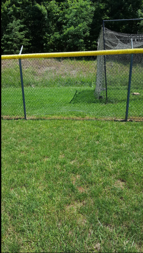
01. Outfield Fence Needing Repair
