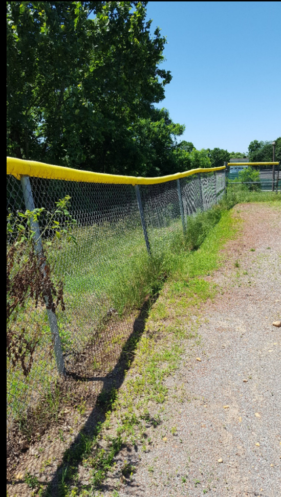
02. Fence Repair Along Left Field Line
