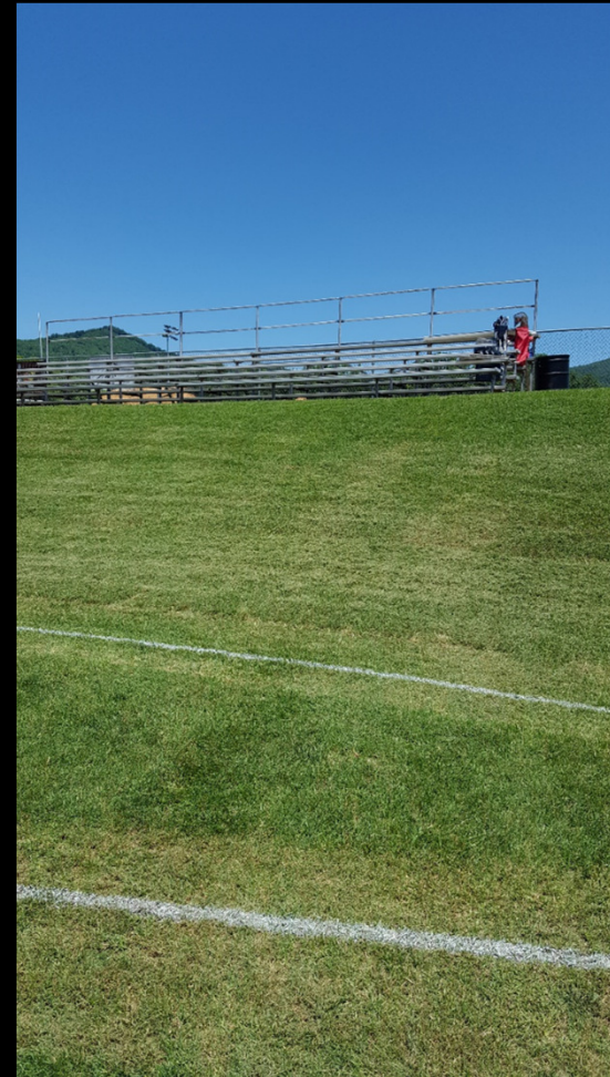
04. Extend Retaining Wall Down Left Field Line
