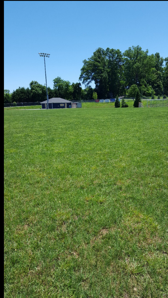
02. No Drop Inlets Around Perimeter
