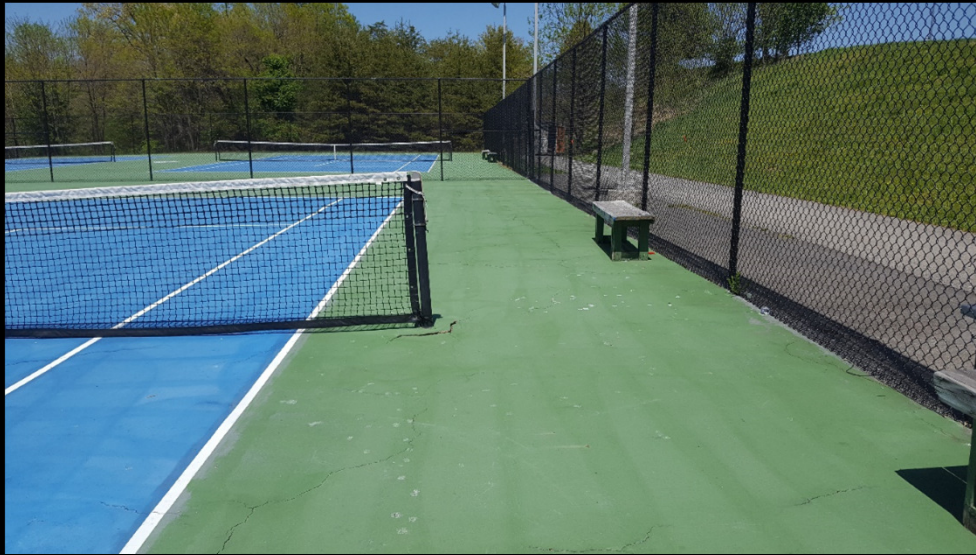
01. Streaks and Surface Delamination
