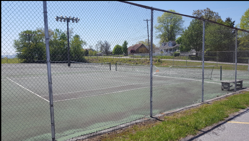
01. Perimeter Fence Condition
