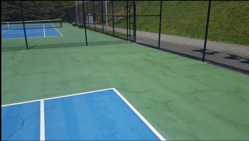
03. Multiple Cracks
