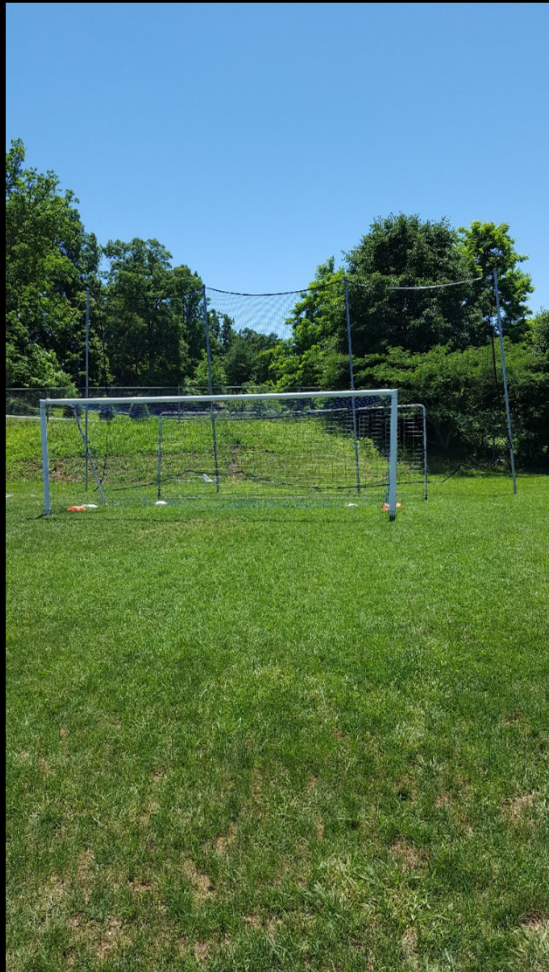
03. End Netting Needing Repair
