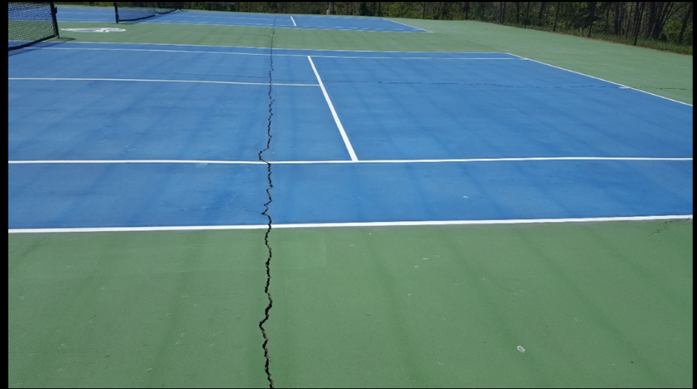
02. Large Crack
