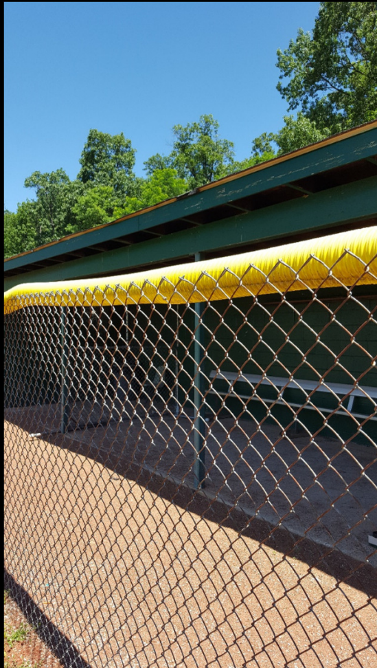
01. Fence Repair in Front of Dugout
