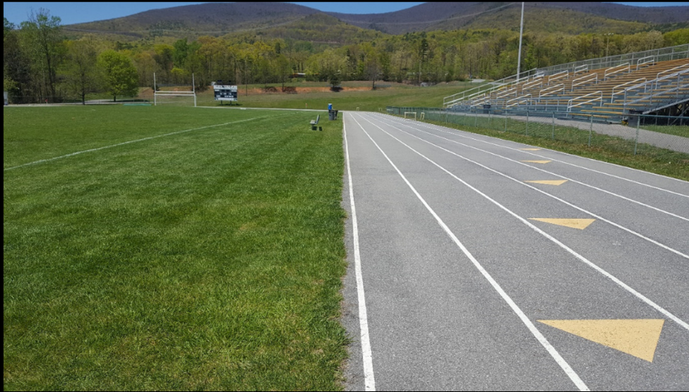
03. No Curb or Trench Drain Along Edge
