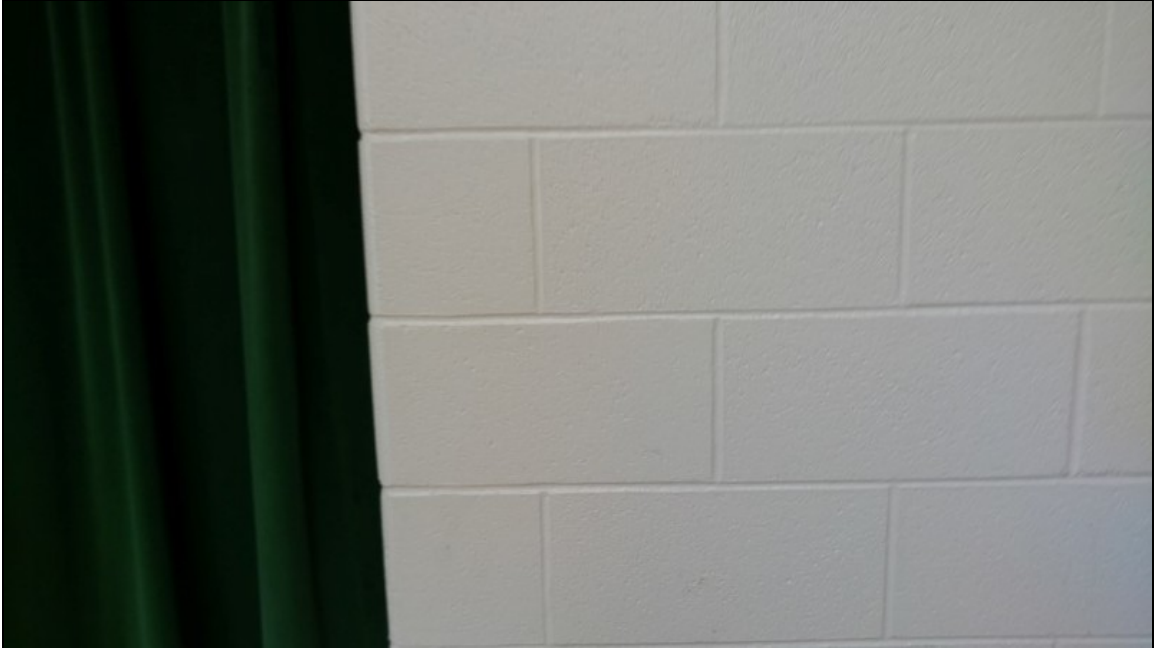
1 - View of typical CMU wall coating, homogenous group 1
