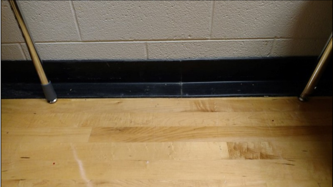
5 - View of typical black 90 degree vinyl cove baseboard, homogeneous group 5
