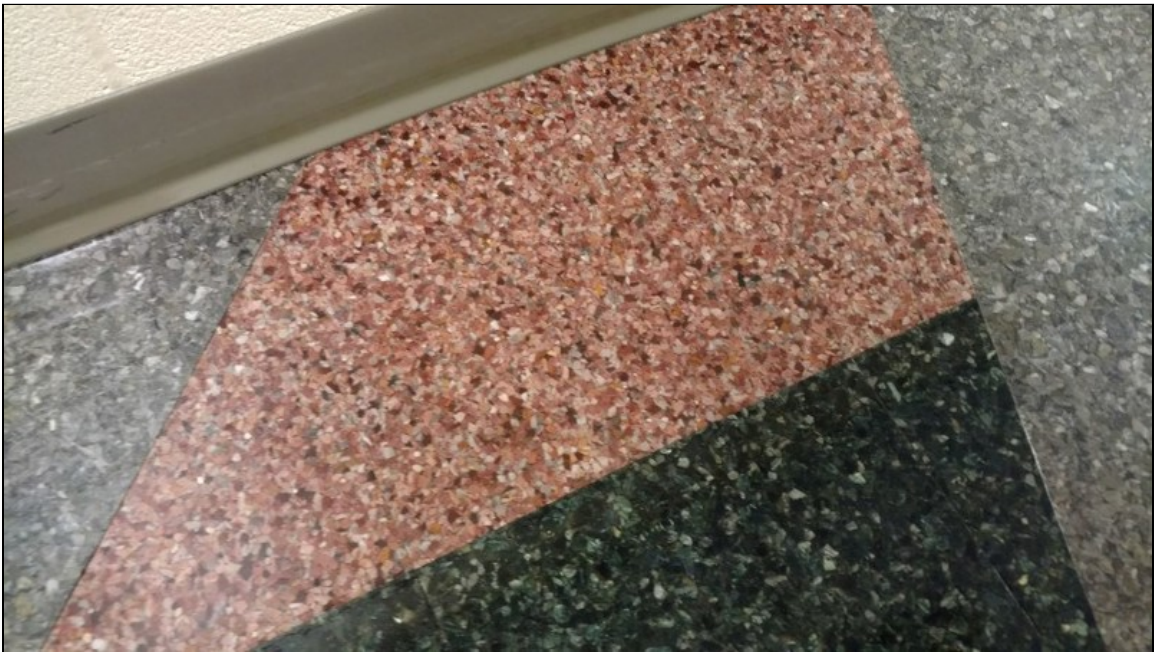
16 - View of typical red aggregate 12"x12" floor tile, homogeneous group 16
