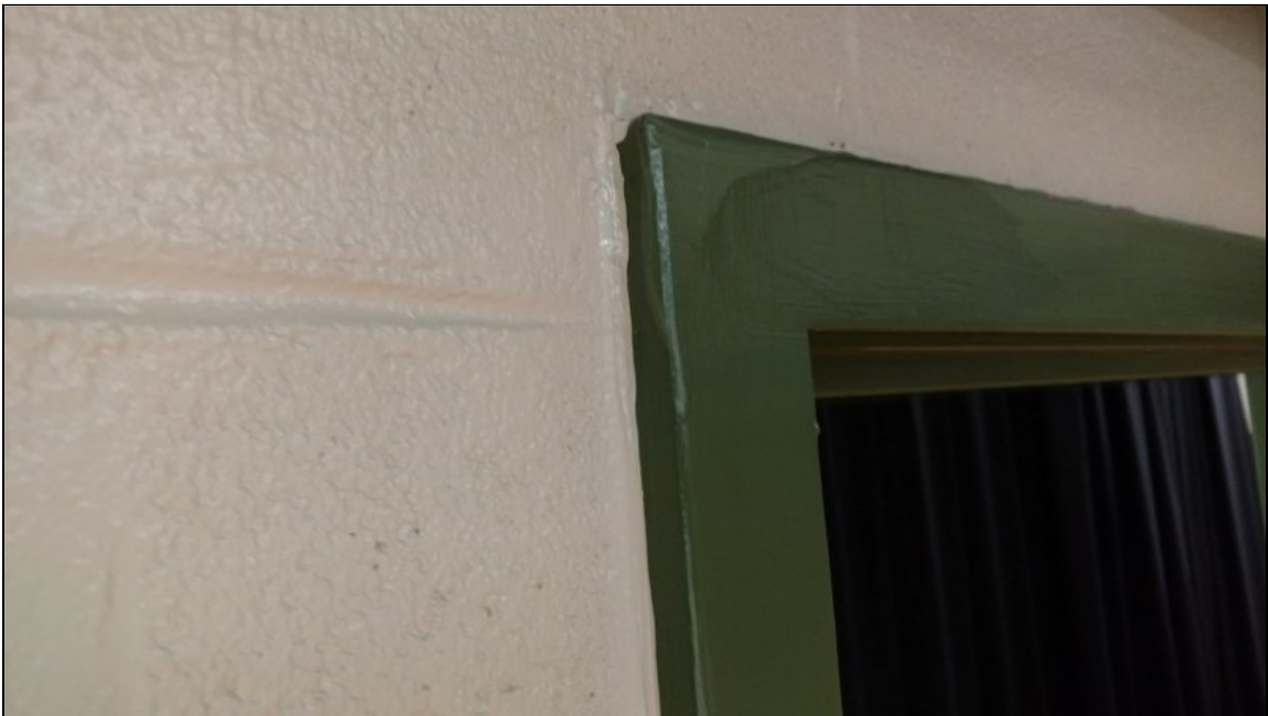
6 - View of typical interior metal door frame caulk, homogeneous group 6
