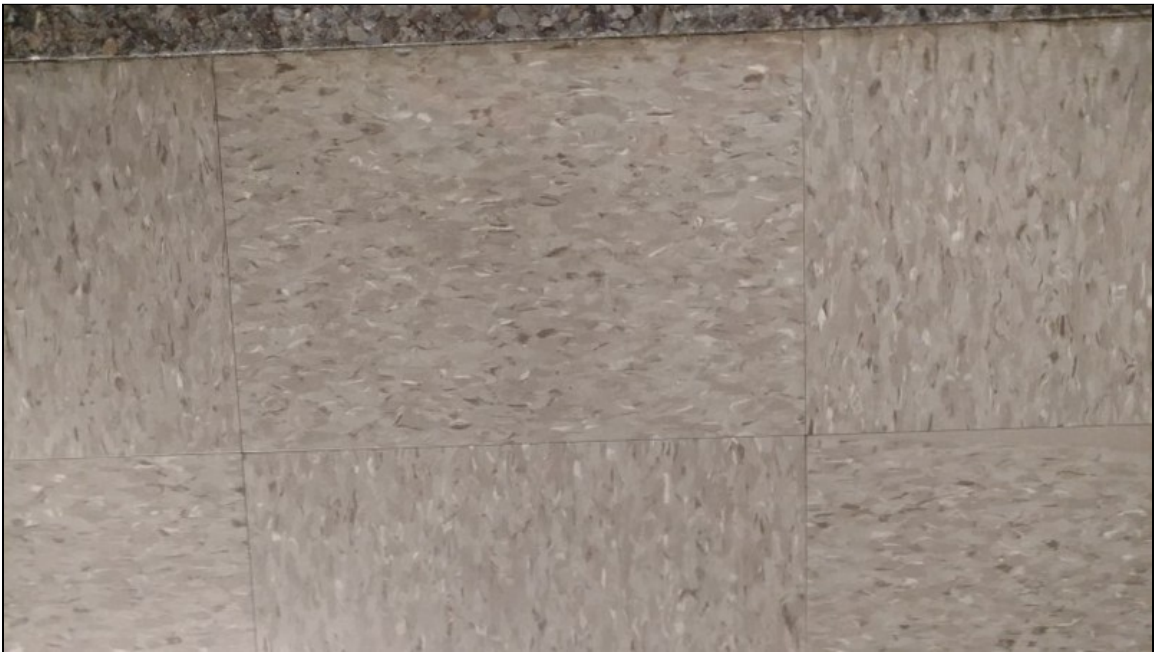
18 - View of typical grey mottled 12"x12" floor tile, homogeneous group 18
