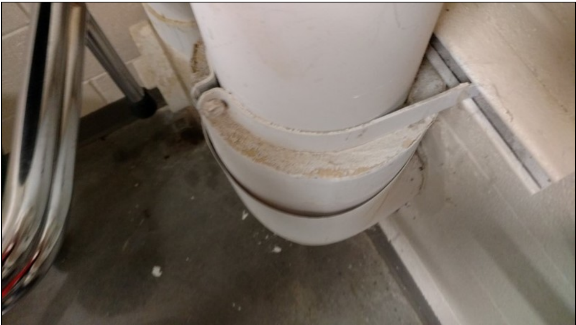
4 - View of typical white mastic on fiberglass pipe insulation, homogeneous group 4
