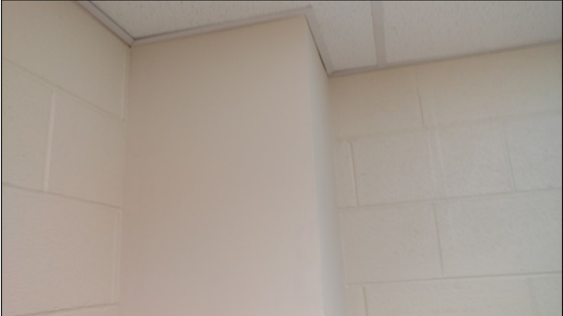
9 - View of typical drywall and joint compound wall, homogeneous group 9
