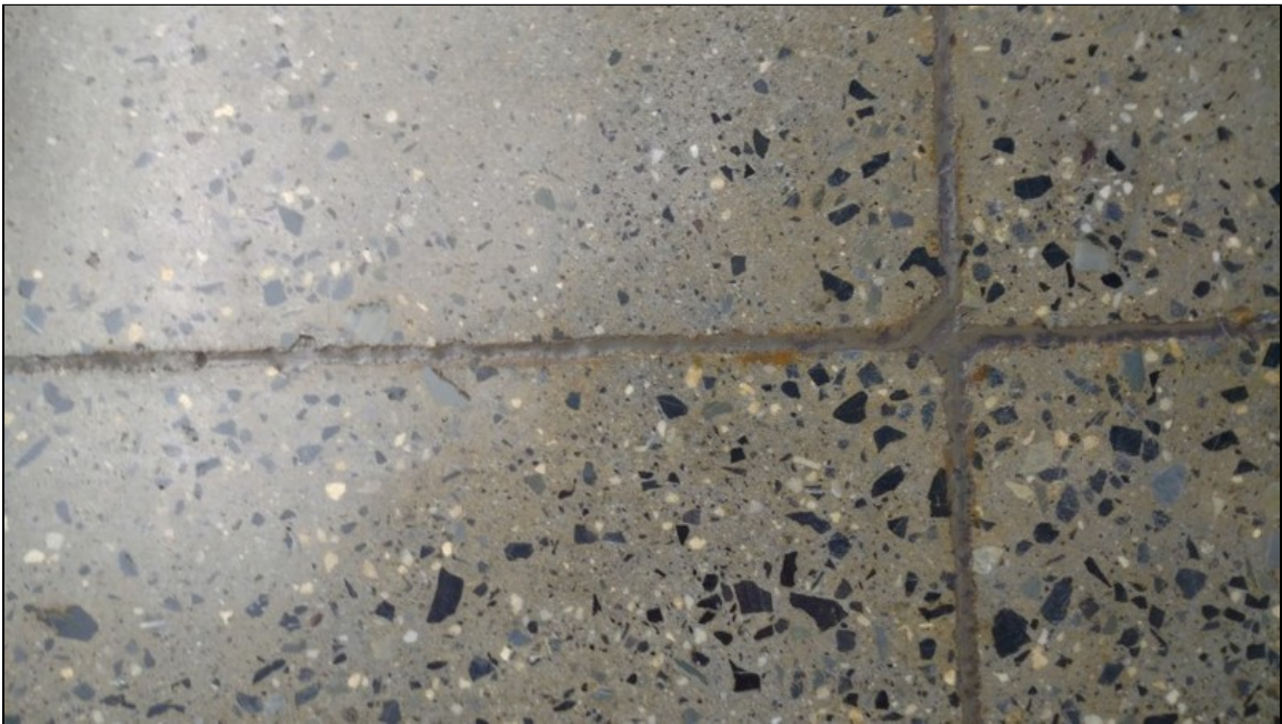
2 - View of typical concrete floor seam caulk, homogeneous group 2
