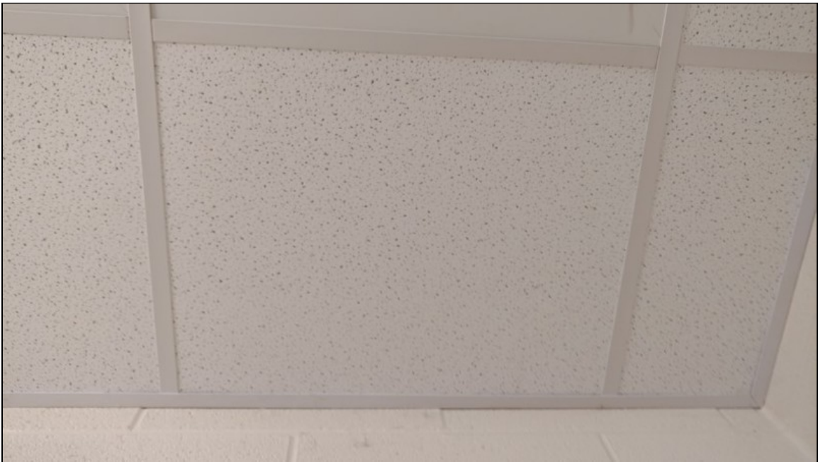
8 - View of typical pinhole/divot ceiling tile, homogeneous group 8
