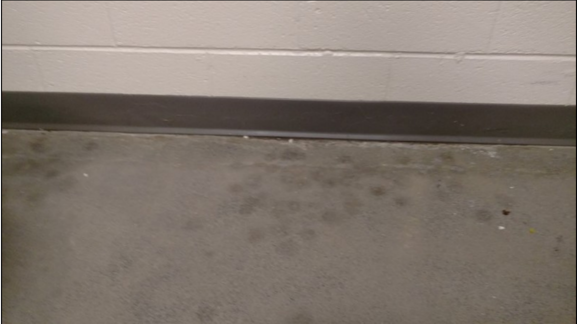
3 - View of typical 4" vinyl cove baseboard, homogeneous group 3
