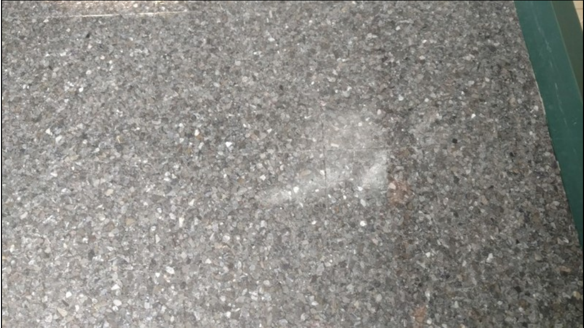
13 - View of typical grey aggregate 12"x12" floor tile, homogeneous group 13
