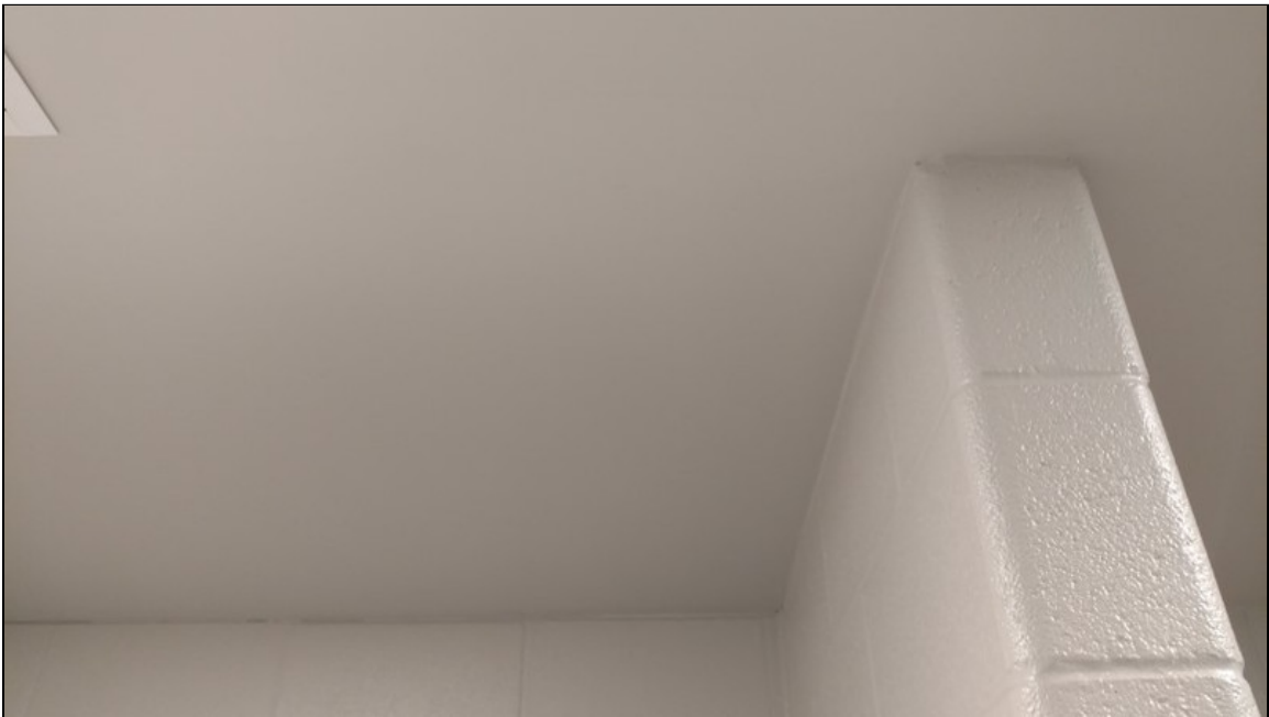
12 - view of typical drywall ceiling
