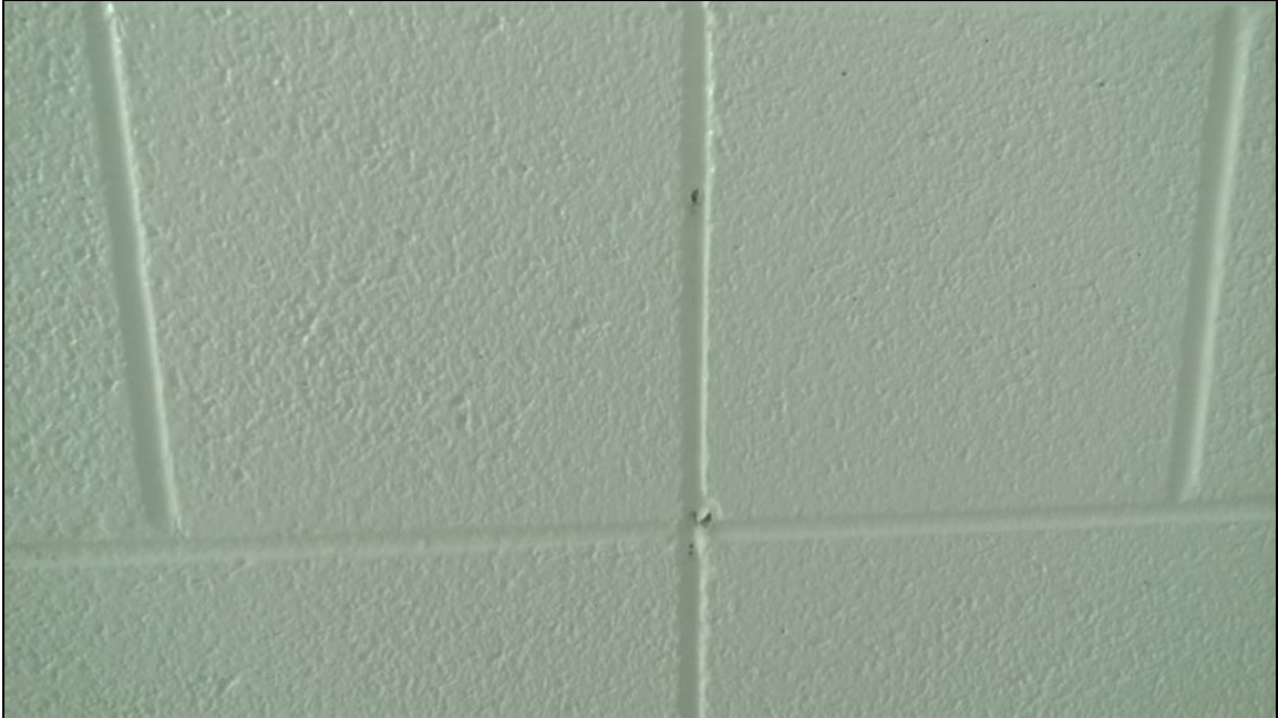
21 - View of typical interior wall expansion caulk
