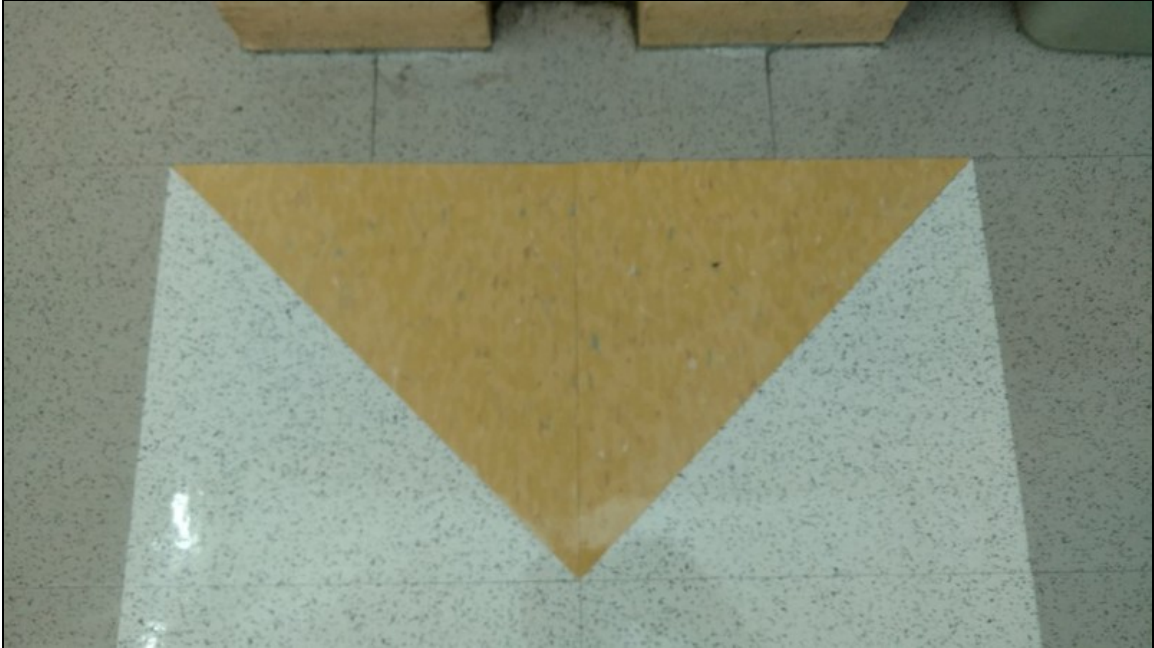
5 - View of typical yellow mottled floor tile
