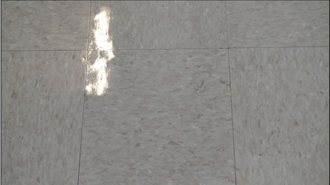
9 - View of typical grey mottled 12"x12" floor tile
