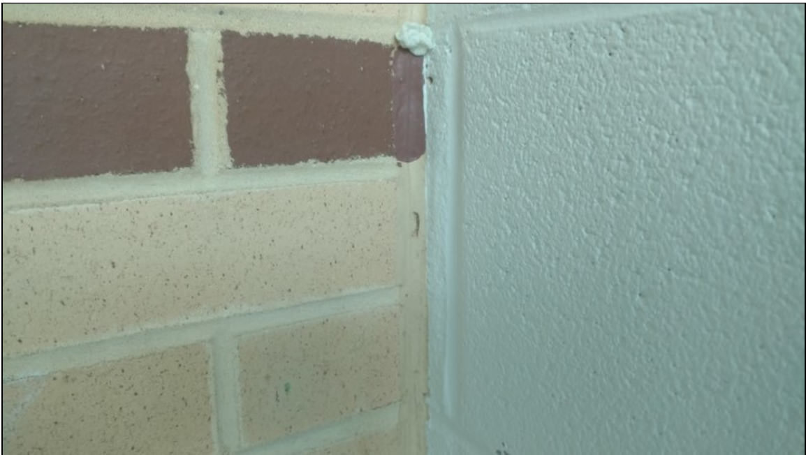
20 - View of typical interior column caulk
