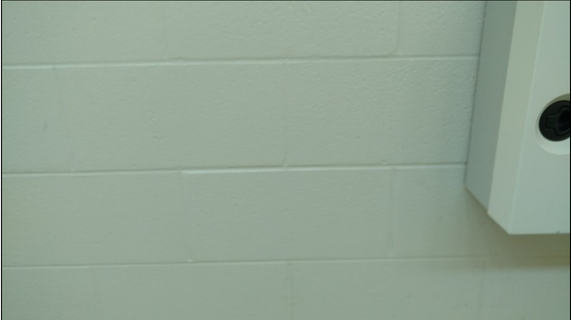
1 - View of typical CMU wall coating
