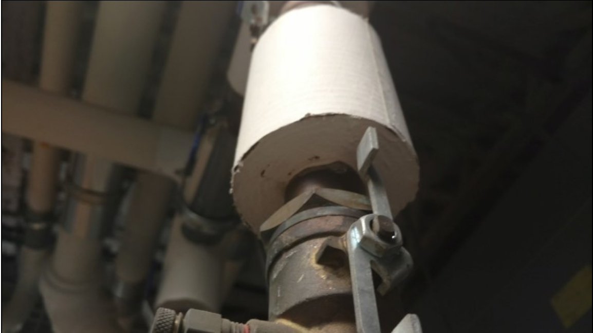
17 - View of typical white fiberglass pipe insulation mastic
