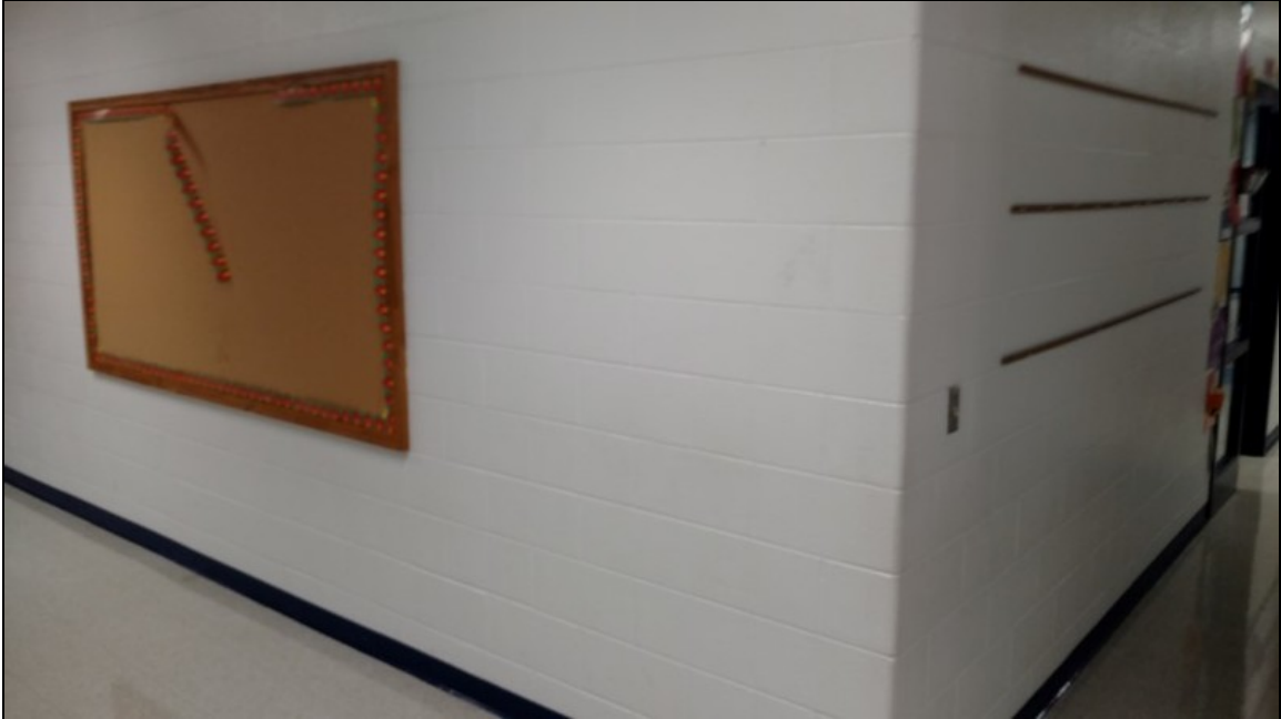
1 - View of typical CMU wall coating
