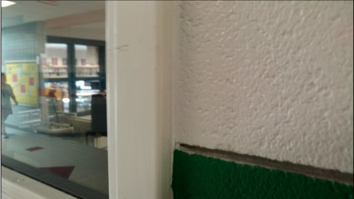
11 - View of typical interior metal window frame caulk
