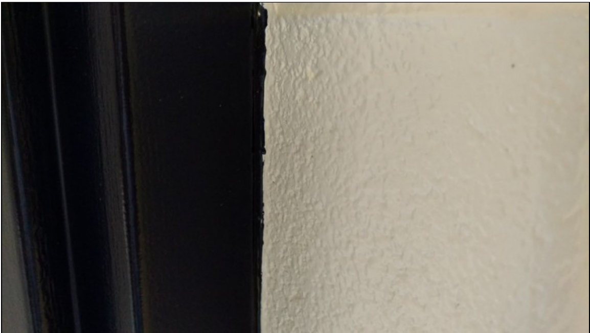
10 - View of typical perimeter door frame caulk
