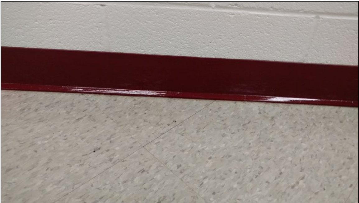
12 - View of typical 4" red vinyl cove baseboard
