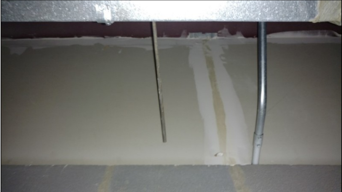
15 - View of typical drywall and joint compound wall
