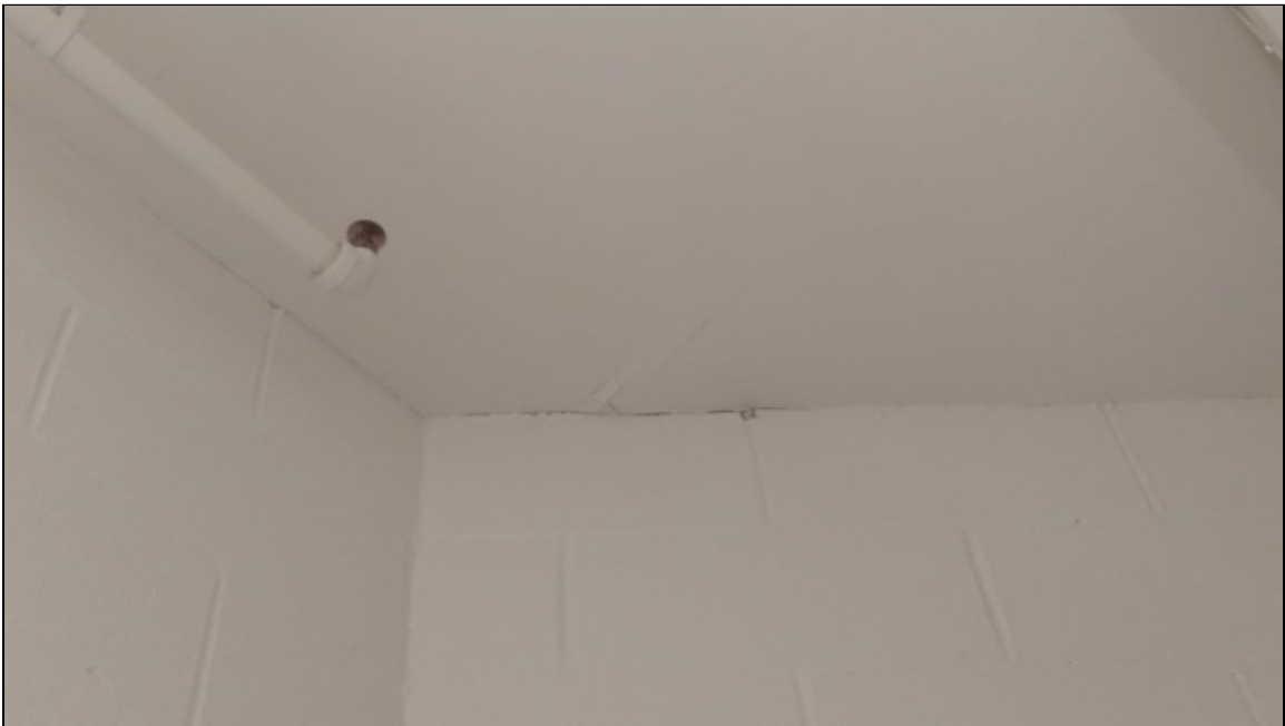
8 - View of typical drywall and joint compound ceiling
