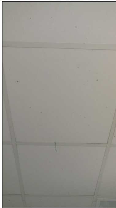
16 - View of typical gypsum ceiling tile
