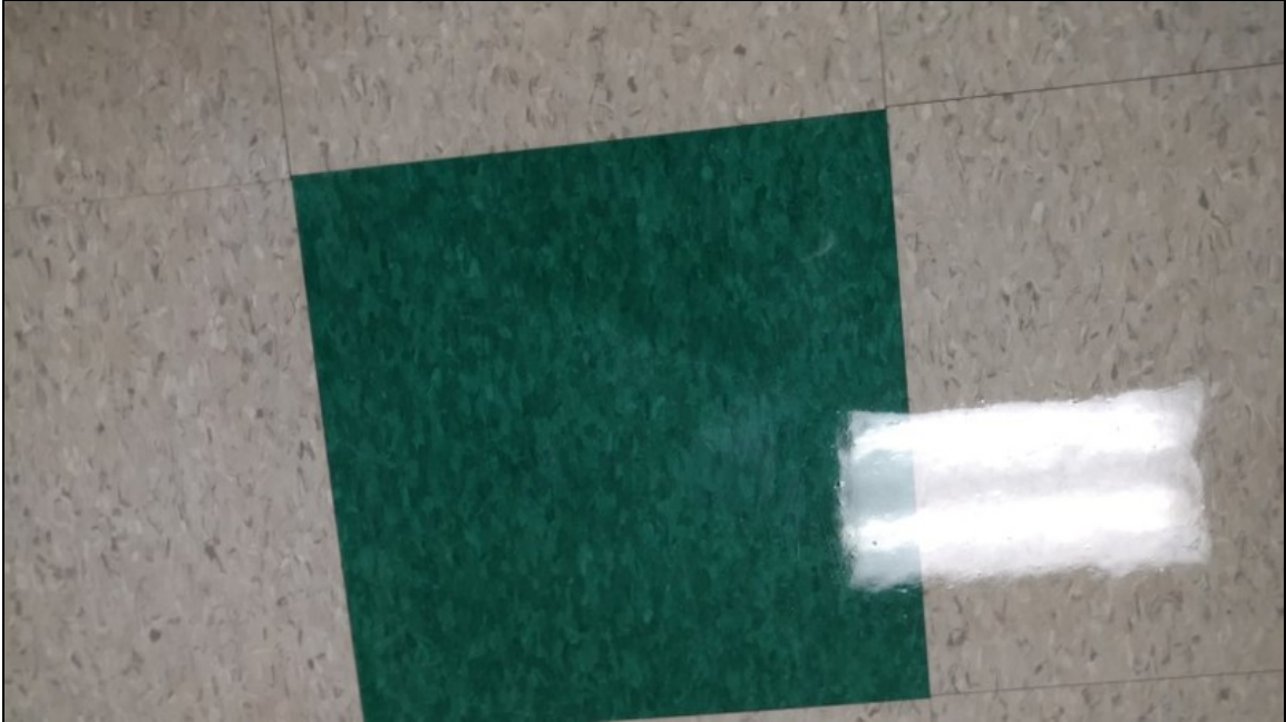
5 - View of typical green mottled 12"x12" floor tile
