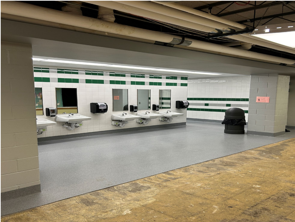
Unit B Bathroom Progress
