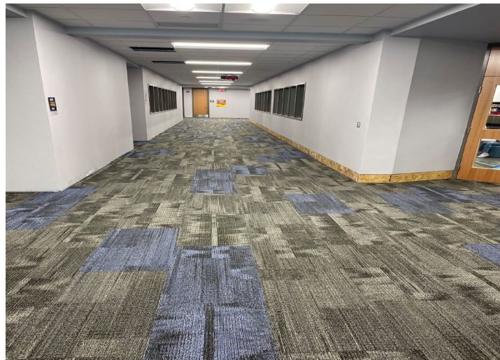
New Carpet Installation
