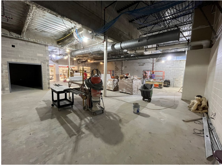
PLTW Lab Progress
