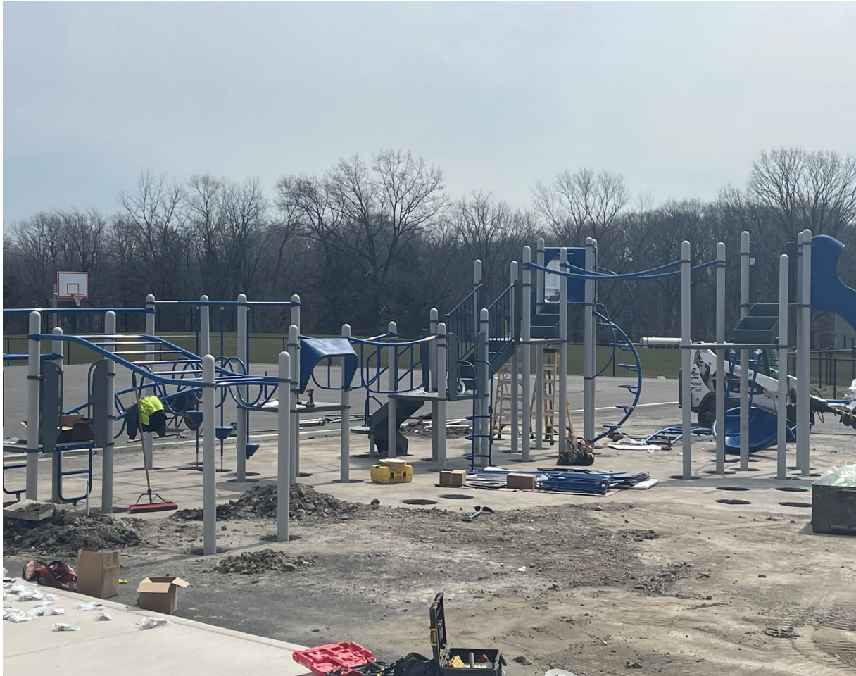
New Playground Equipment
