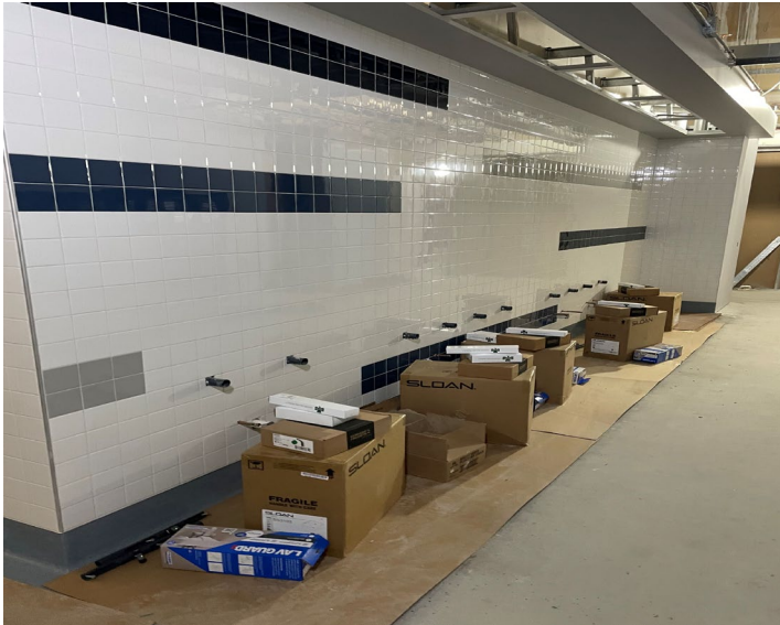
Wall Tile in New Bathrooms
