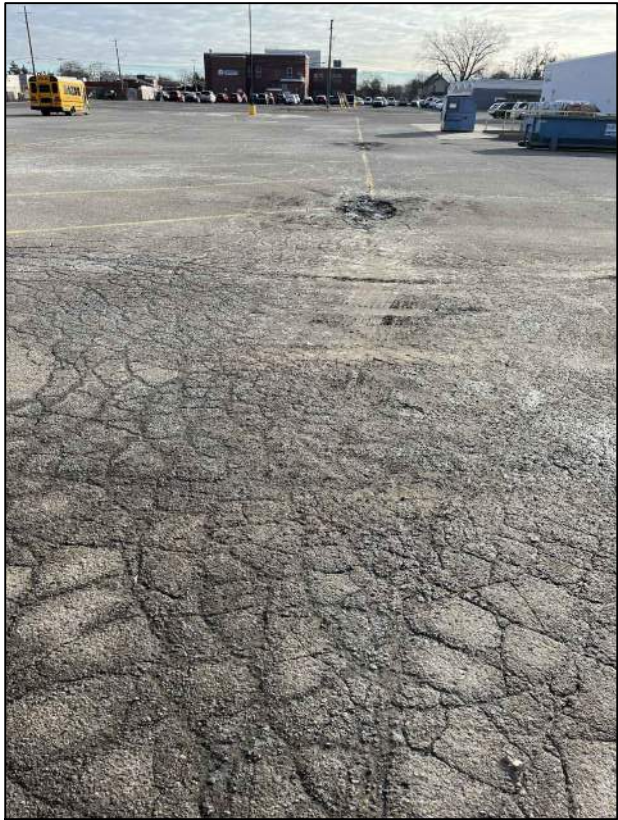
1 Severe Alligator Cracking - Potholes NTS
