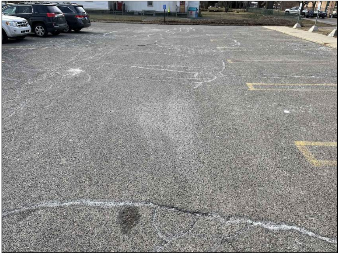
Block Cracking - Salt Buildup
