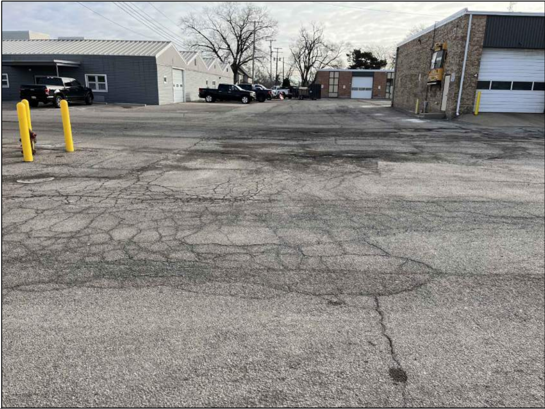
Block Cracking - Alligator Cracking - Potholes
