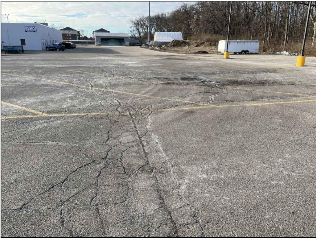
3 Edge Cracking - Potholes - Alligator Cracking
