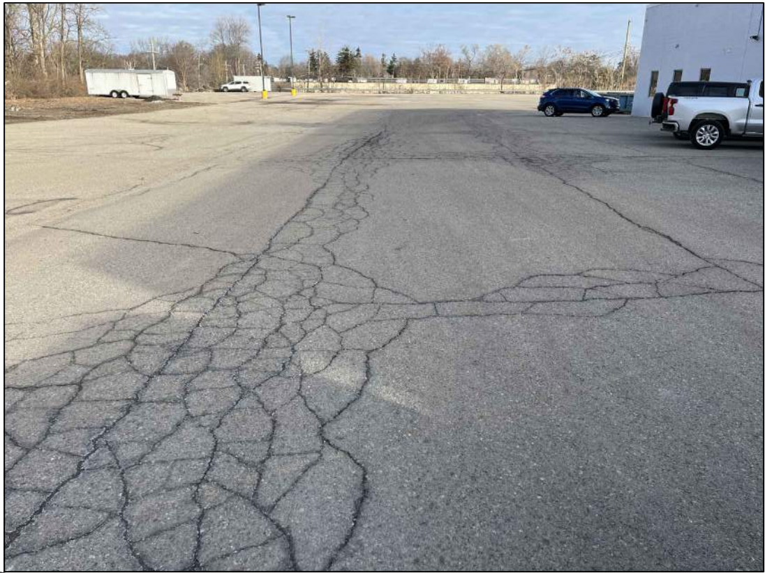
2 Joint Cracking - Alligator Cracking NTS
