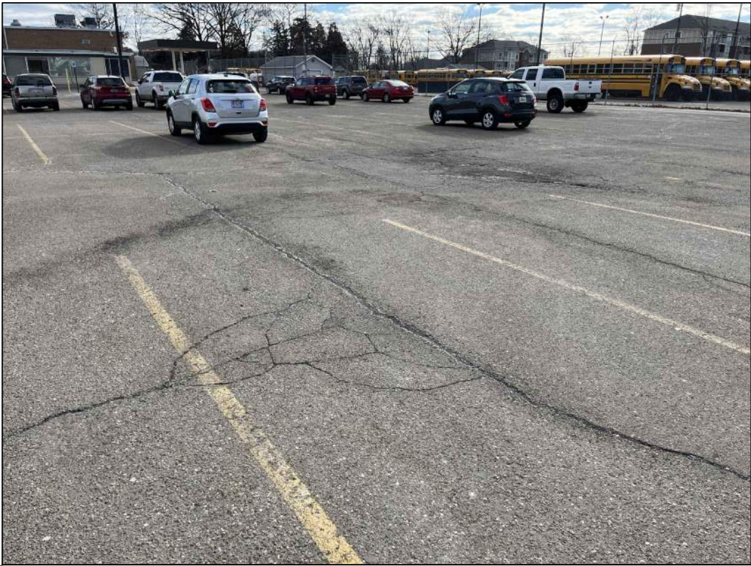
3 Block Cracking - Alligator Cracking - Potholes NTS
