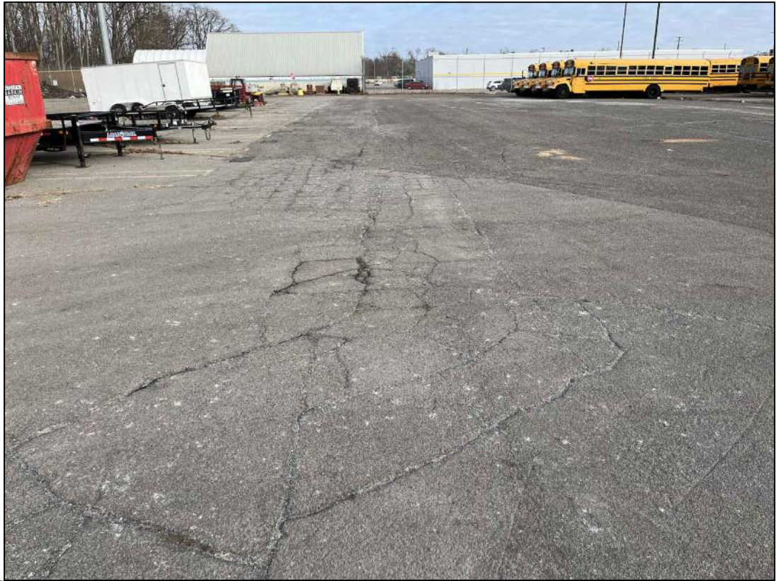
1 Alligator Cracking NTS
