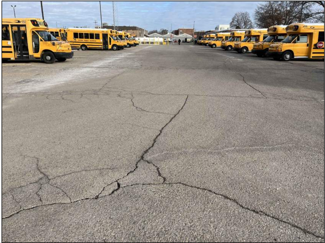
1 Block Cracking NTS
