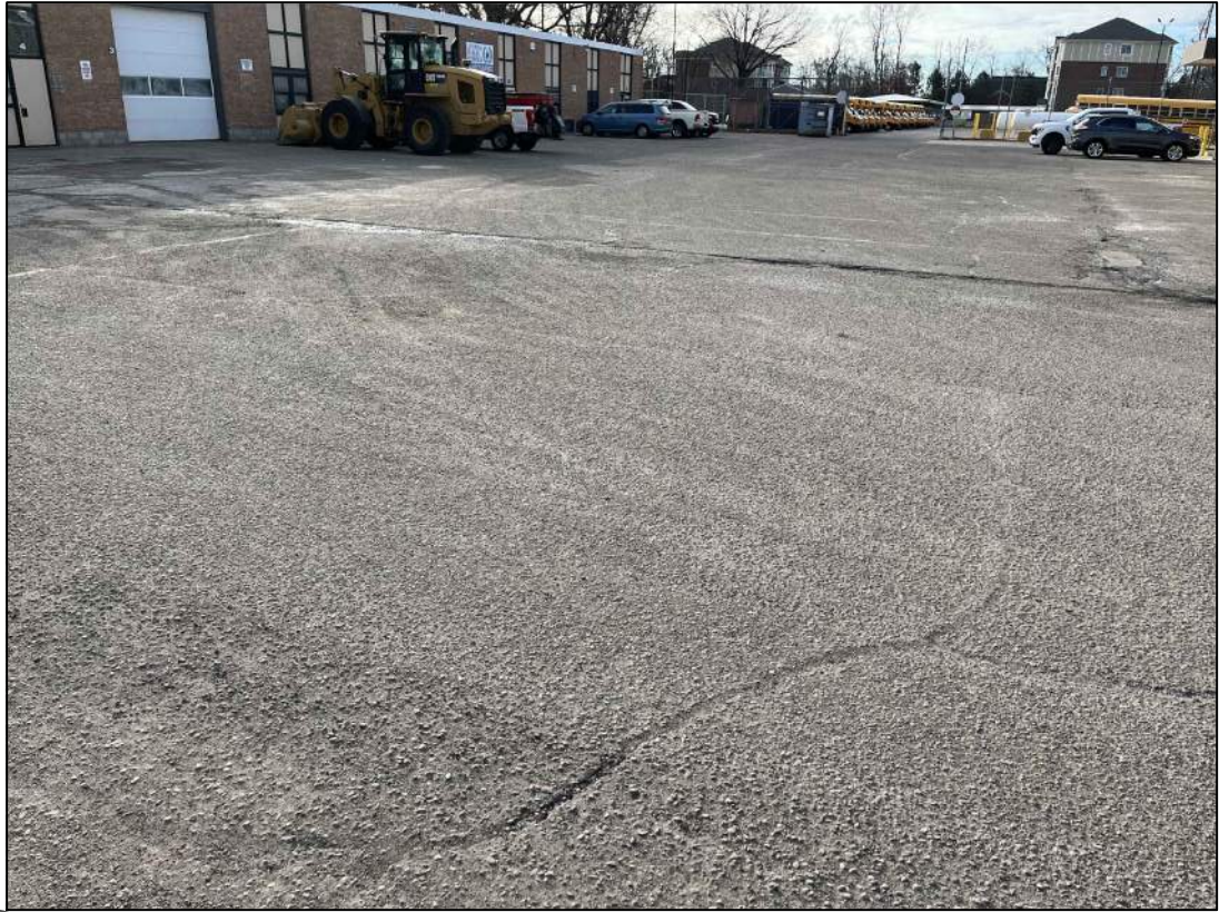
Block Cracking - Potholes
