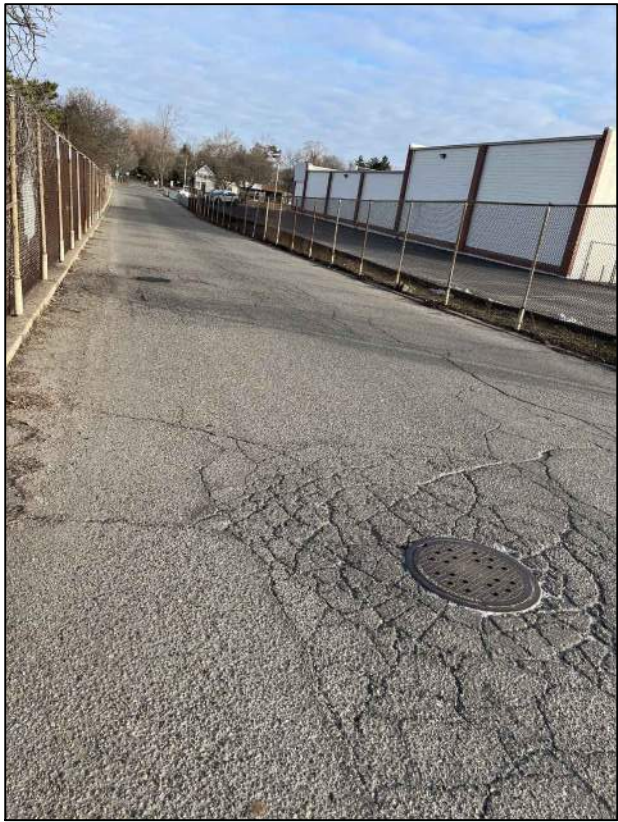
2 Alligator Cracking Surrounding Manhole
