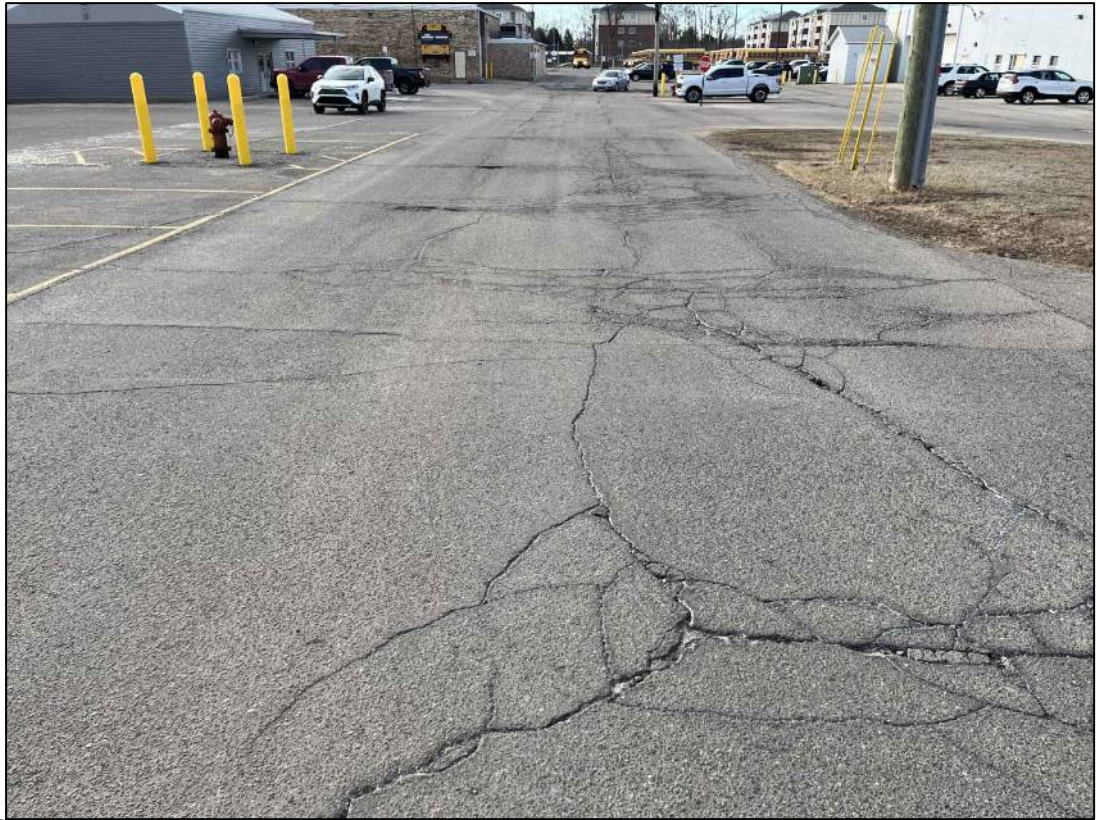
1 Block Cracking - Alligator Cracking NTS
