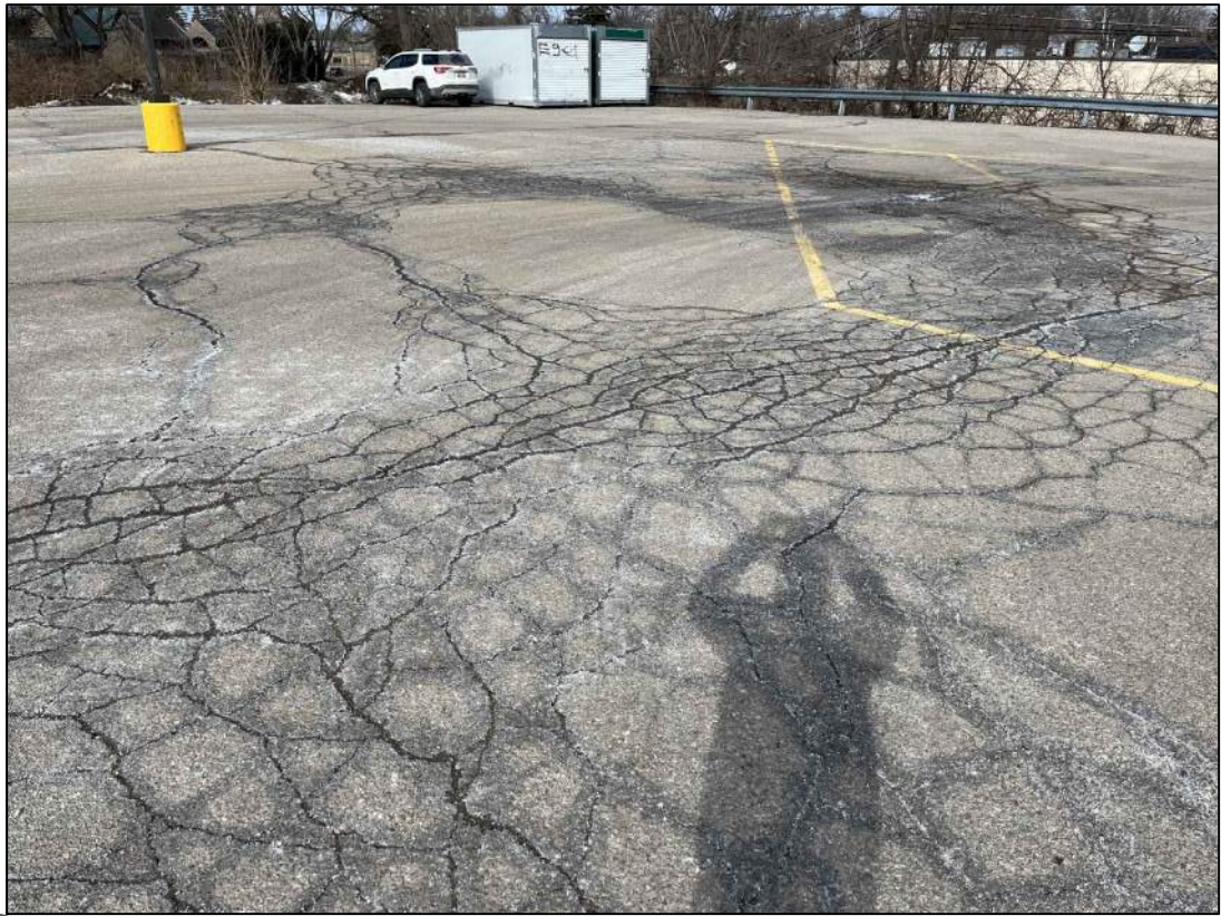
2 Block Cracking - Alligator Cracking NTS
