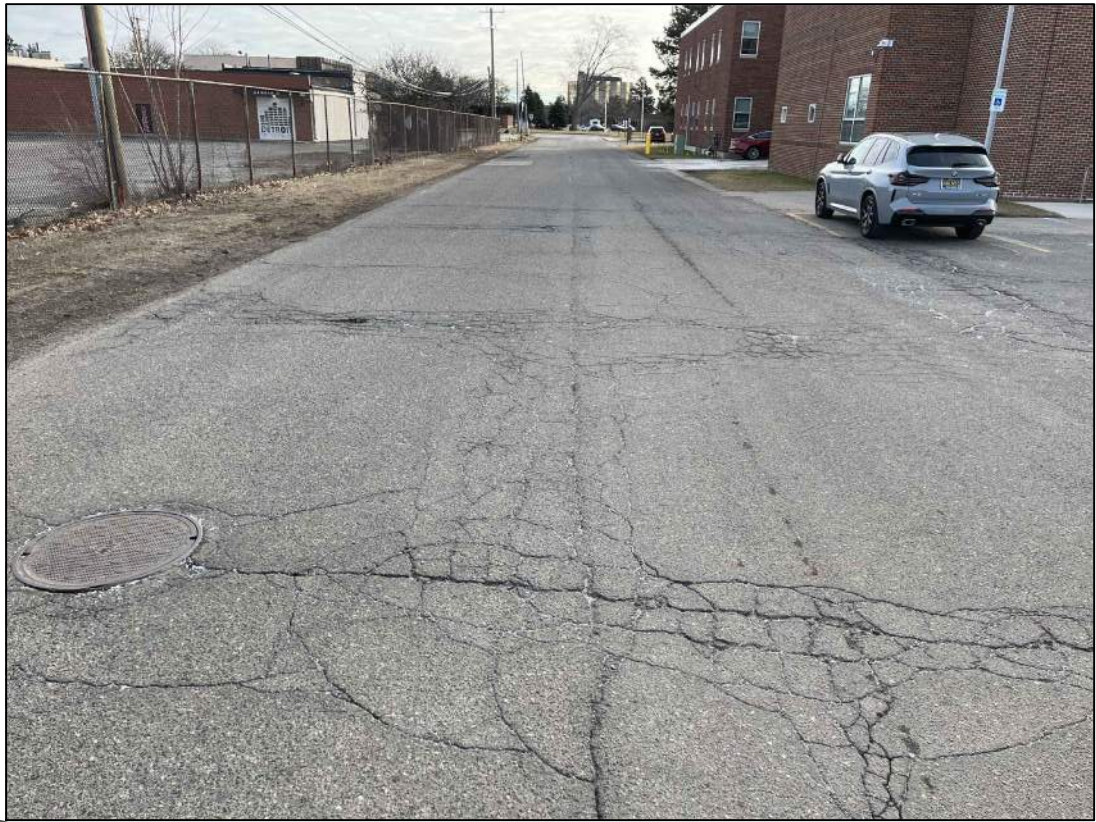
2 Block Cracking - Alligator Cracking NTS
