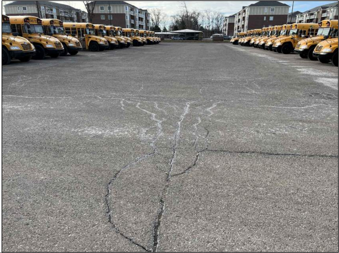
2 Block Cracking NTS
