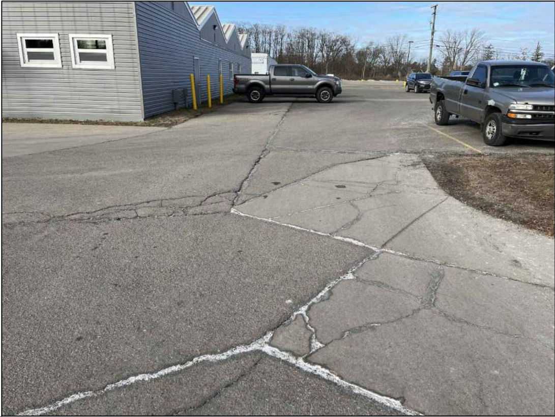
Alligator Cracking - Salt Buildup
