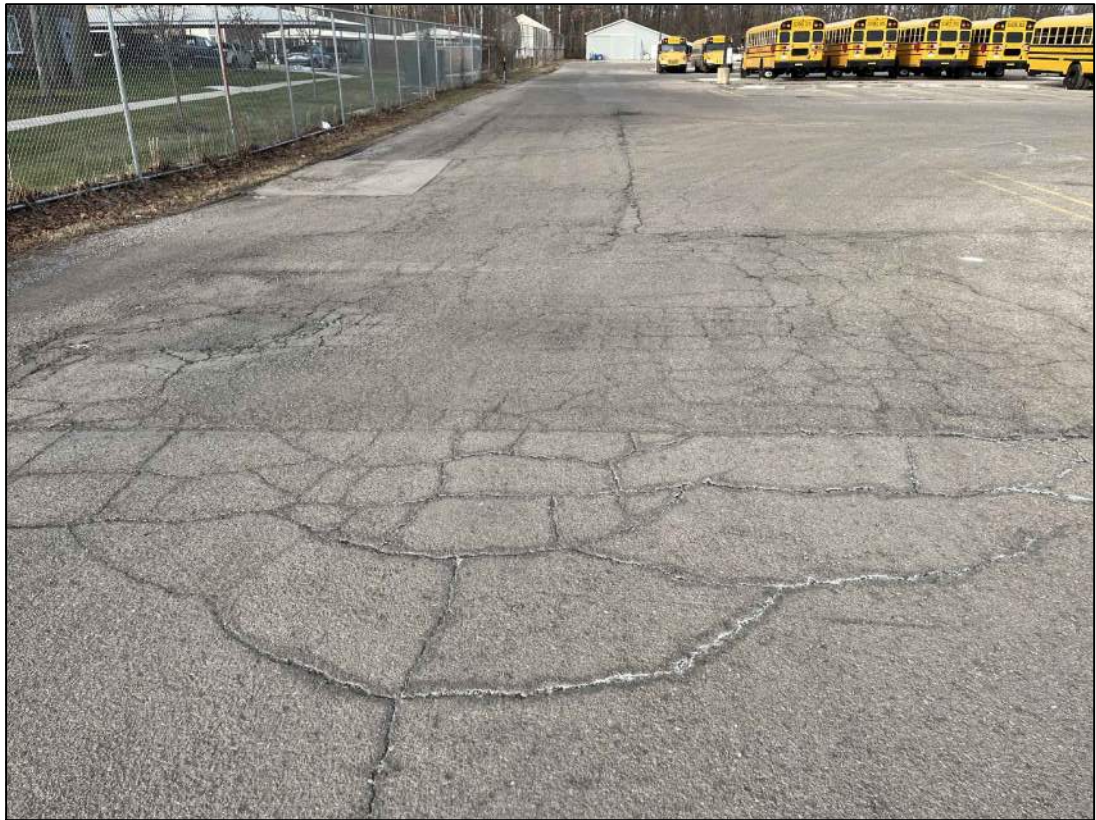
2 Alligator Cracking NTS
