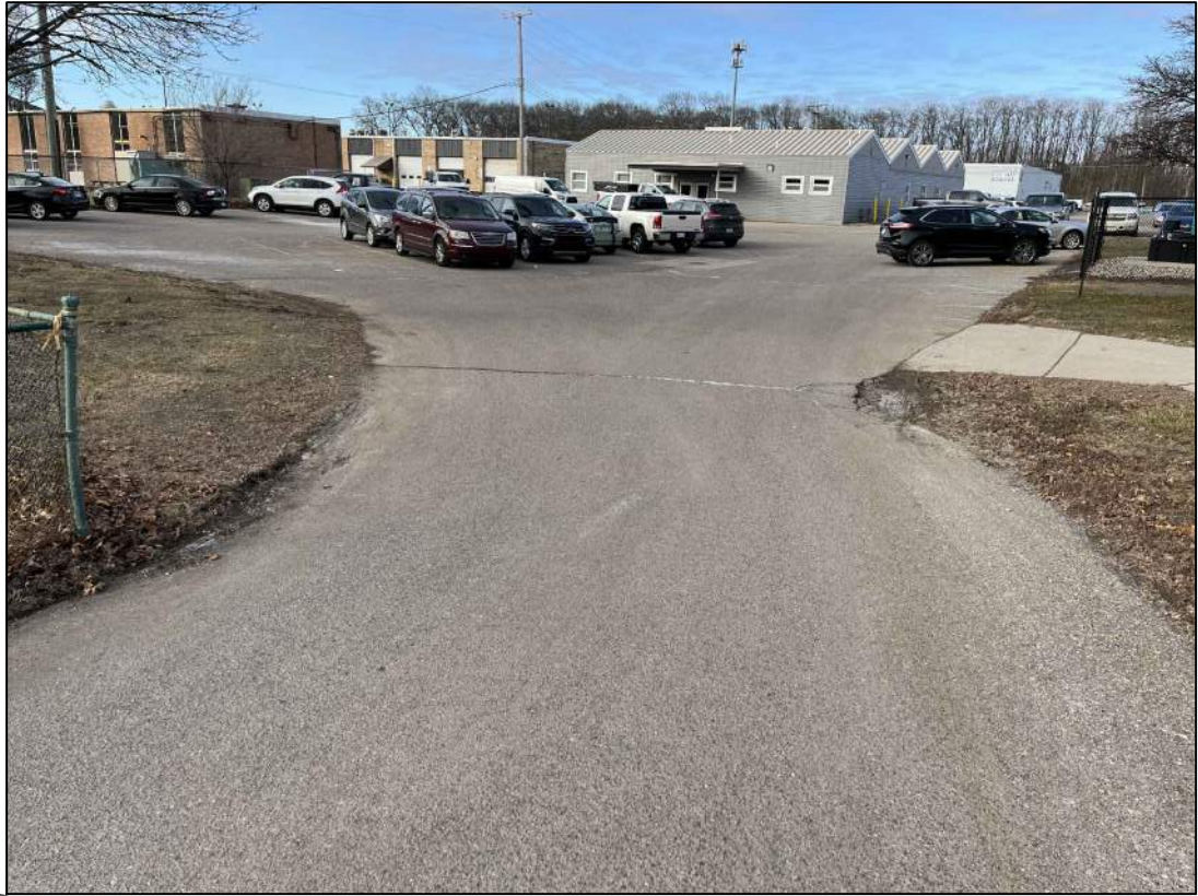
Transverse or Joint Cracking
