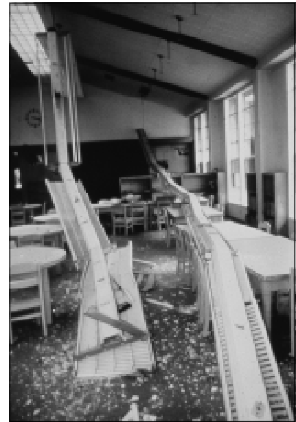
Light fixtures were dislodged in Coalinga's schools during a 1983 earthquake.
