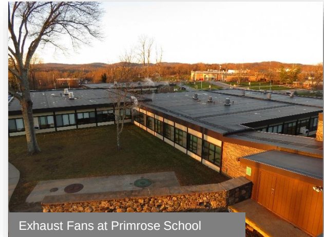
BMS Panel at High School
