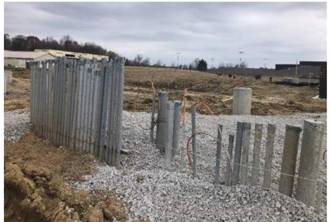
04.09.24 - Underground Conduit for Main Distribution Panel
