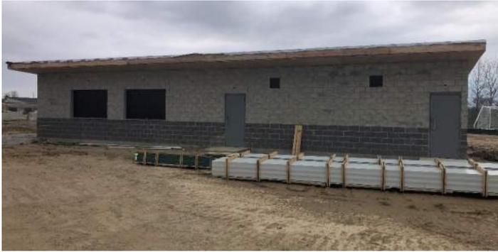
4.09.24 - Concessions Building - Rollup Doors & Hollow Metal Doors installed
