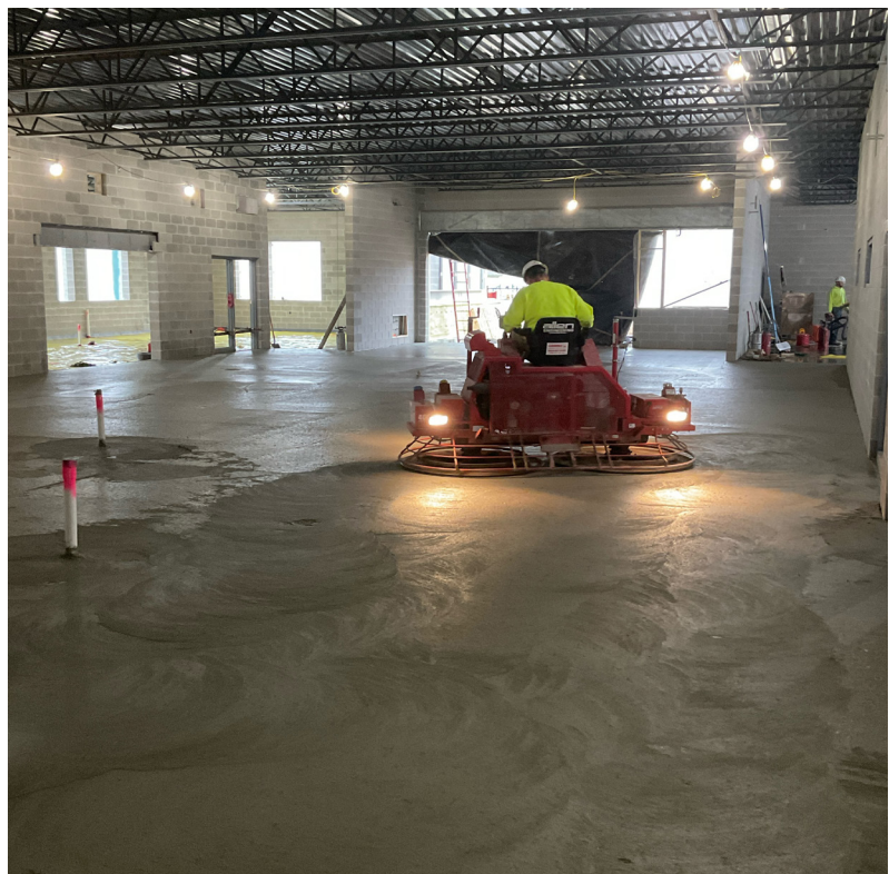
KINDERGARTEN AREA | CONCRETE FLOOR LEVELING
