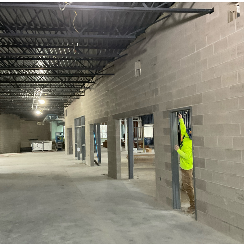
MEDIA CENTER | MASONRY WALL
