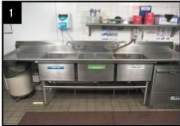
Clean and sanitize pot washing area.
