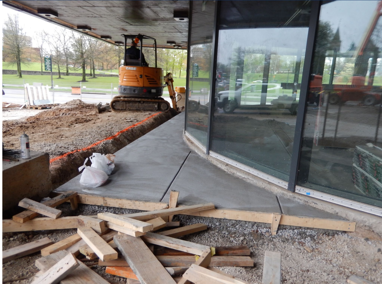
Exterior concrete slab work
