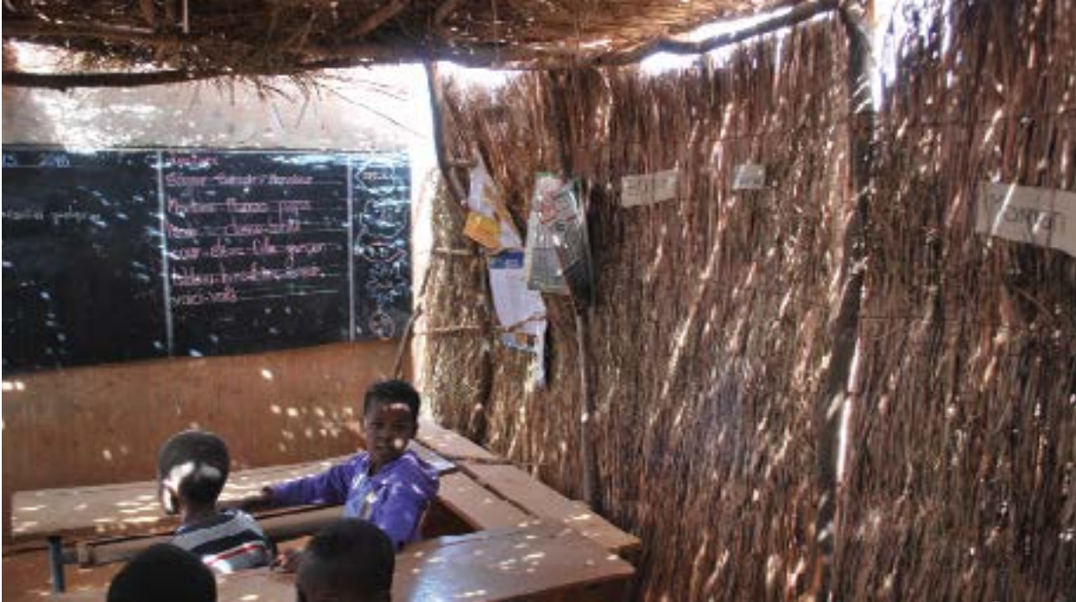
Old classroom made of straw and branches and a blackboard secured to the outer wall of another classroom.
