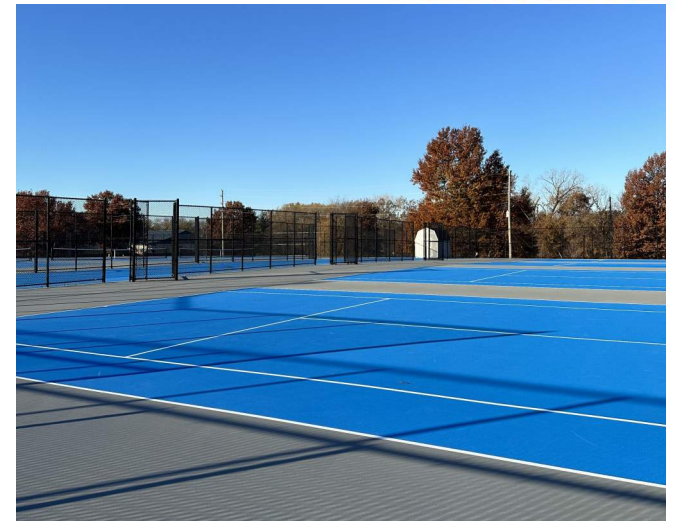
North Courts Looking Southwest
