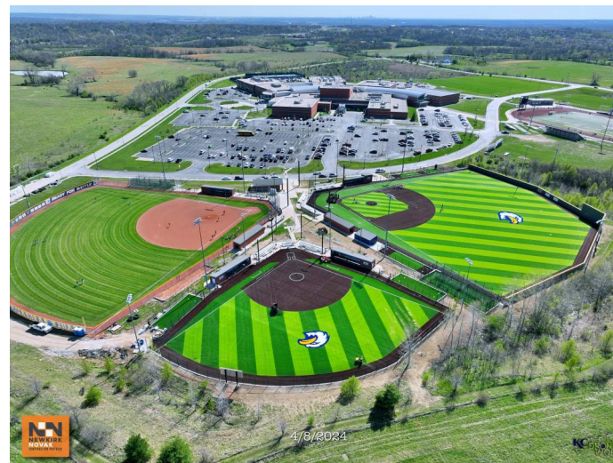
LNHS - Overall Site
