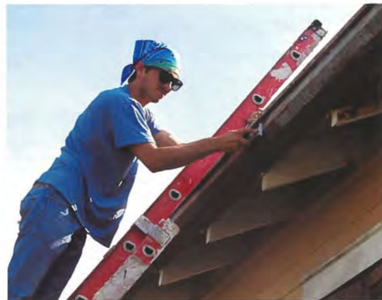
Above: Climbing high, Senior Ryan Bibby scrapes the paint off the top of a building.
