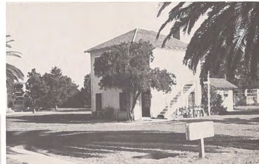
Side view of the boiler room and shop building.
