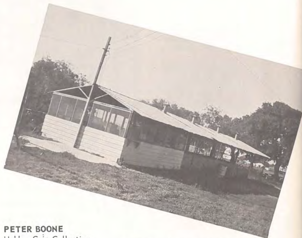
A side view of the barbecue pit on the school's campus.
