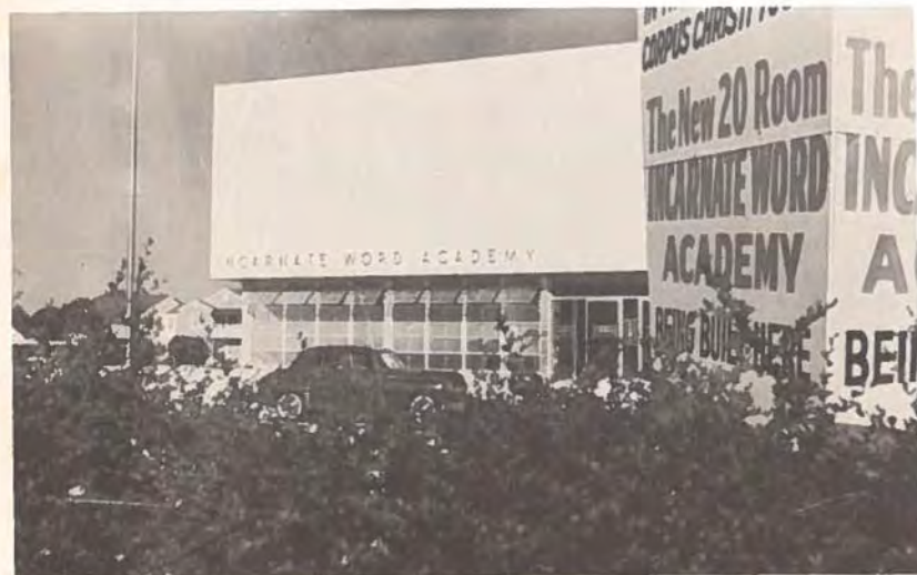
By December our new building looked nearly completed to our inexperienced eyes. We felt ready to move right in when they put the name on the front of the building.
