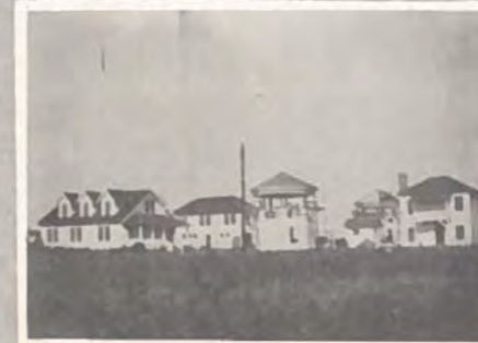
December 20, 1927--- danger threatens the completion of the school here, by the destruction of the Abbey by fire.
