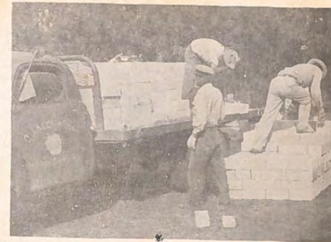
First load of tile --- May '51
