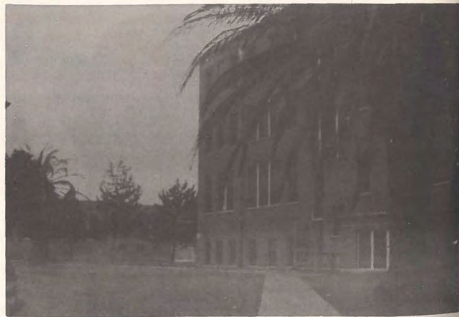
MAIN BUILDING - SOUTH SIDE
