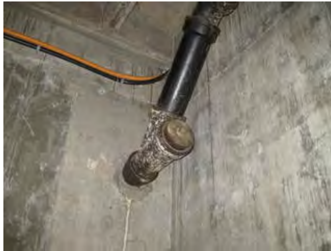
Cast-iron sanitary piping
