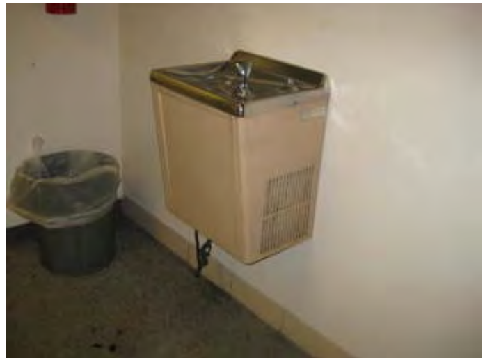
Non-compliant electric water cooler
