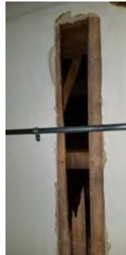
Wood roof structure at 1905 original construction
