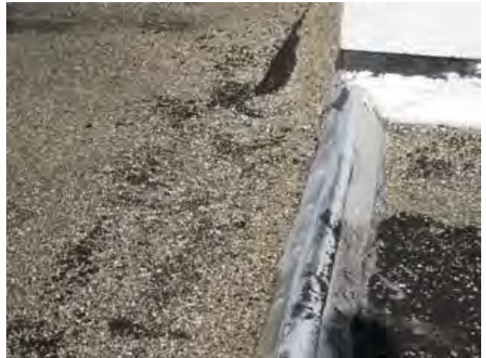
Roofing expansion joint
