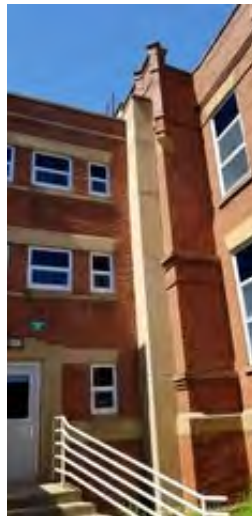
Brick veneer at 1905 original construction
