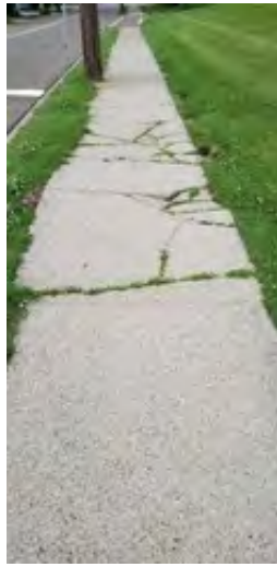
Damaged concrete sidewalks
