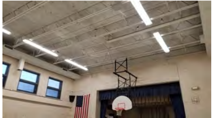
Exposed bar joist and insulated panel
