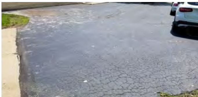
Asphalt pavement in poor condition
