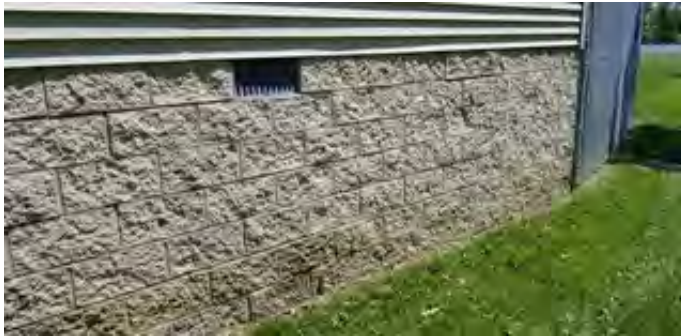
Masonry foundation wall at 2002 addition
