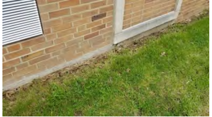
Masonry block foundation
