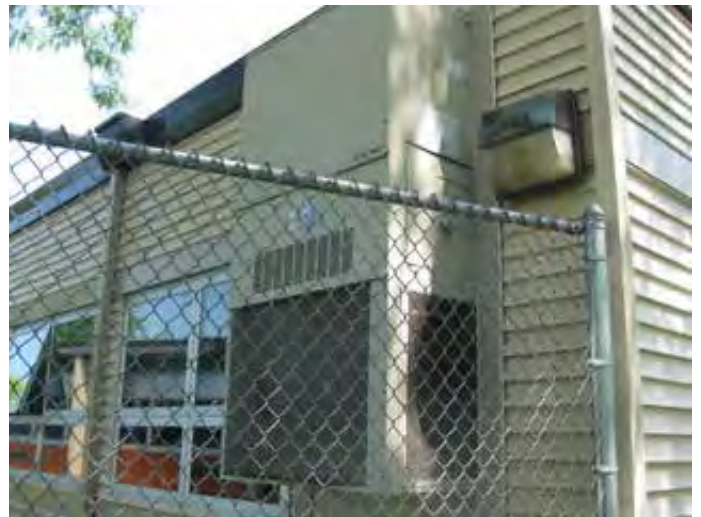
2002 addition packaged HVAC unit
