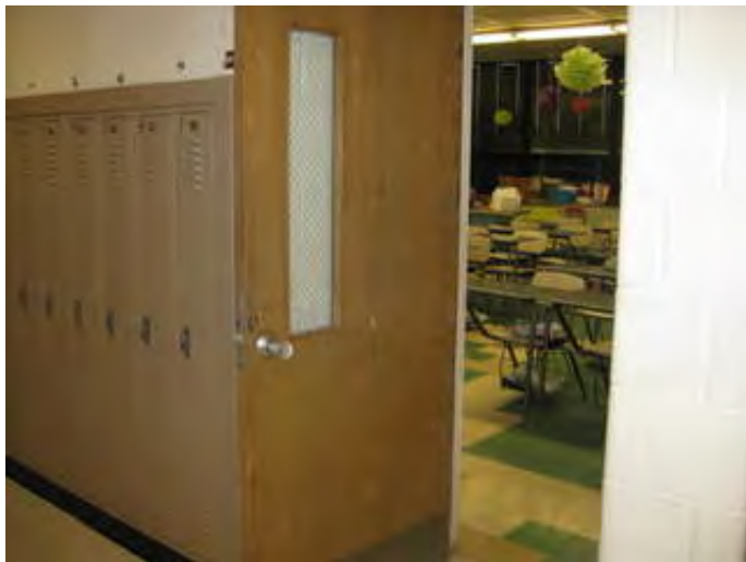
Non-compliant door hardware and clear space
