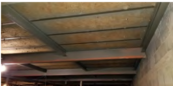
Steel frame roof with insulated panel at stage
