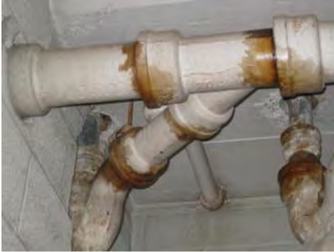
Cast-iron sanitary sewer piping
