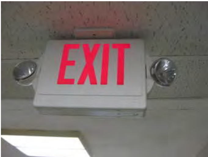
Combination exit and emergency lighting fixture in 1962 original building
