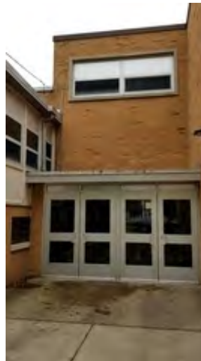
Typical exterior brick veneer
