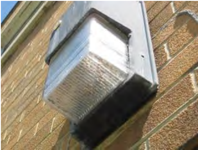
Wall mounted exterior lighting fixture
