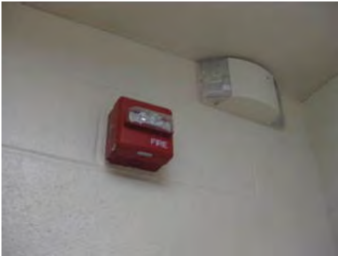
Fire alarm horn strobe device
