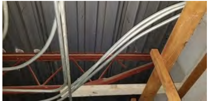
Metal deck on steel bar joist at 1965 addition
