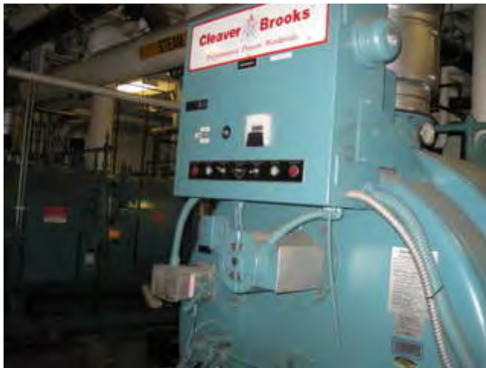
Gas fired boiler
