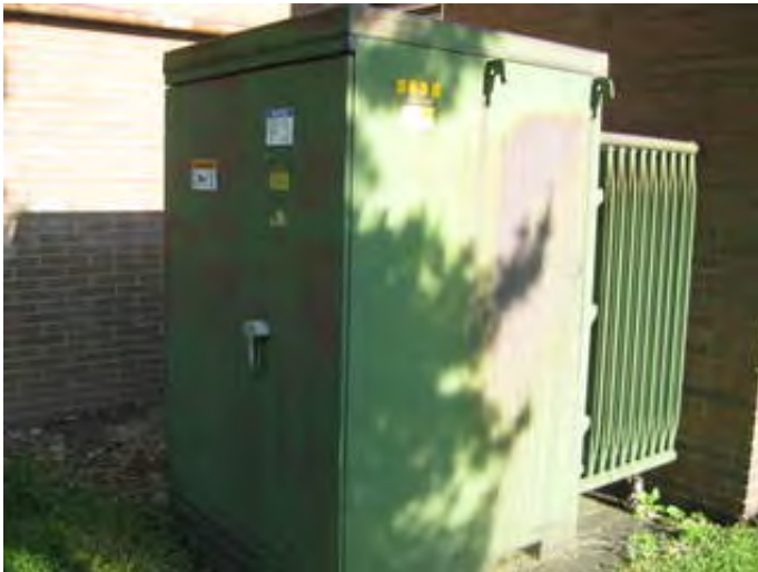
Pad mounted transformer
