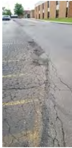
Asphalt pavement in poor condition
