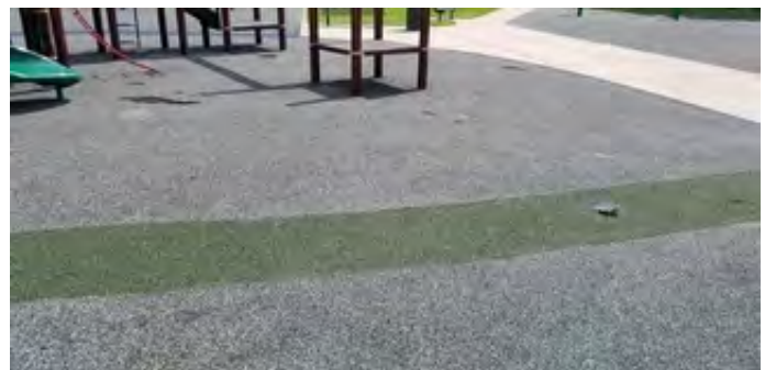
Damaged rubberized soft surfacing at playground
