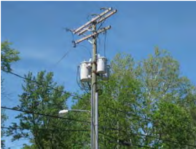
Pole mounted transformers
