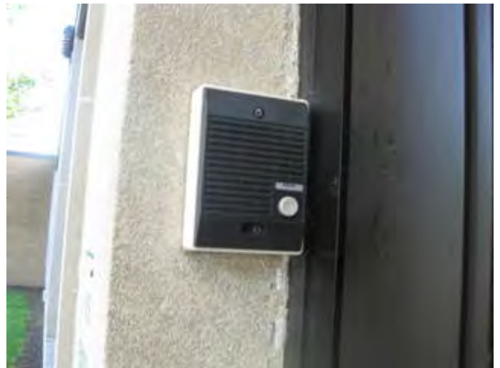
Remote door buzzer intercom and electric door strike
