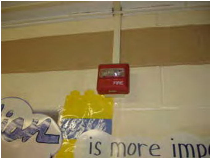
Wall mounted horn/strobe device
