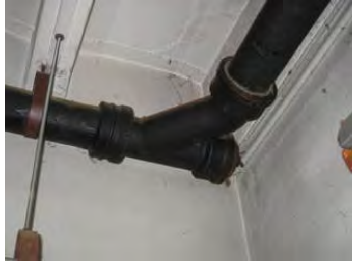
Cast-iron sanitary sewer piping
