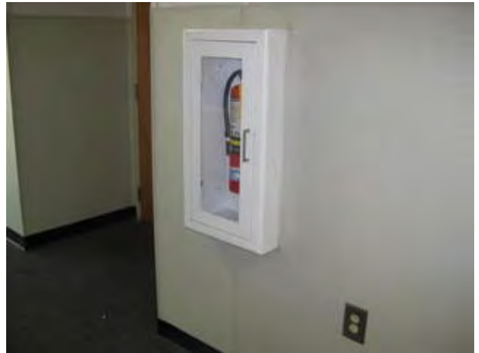
Fire extinguisher cabinet in 2002 addition
