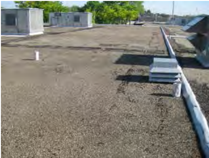
Built-up asphalt roofing
