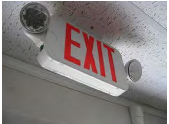
Combination exit and emergency lighting fixture in 2002 addition
