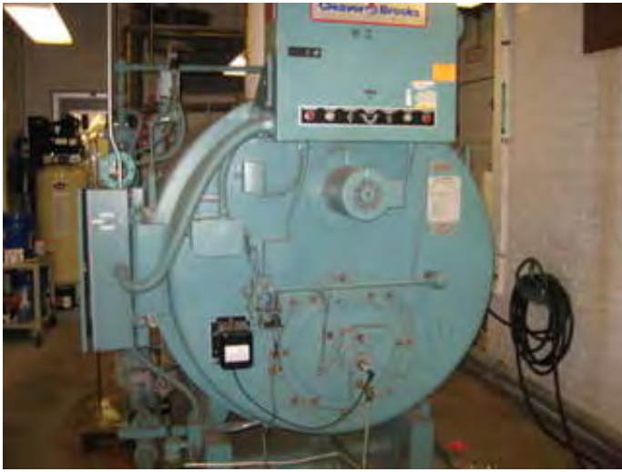
Gas fired boiler
