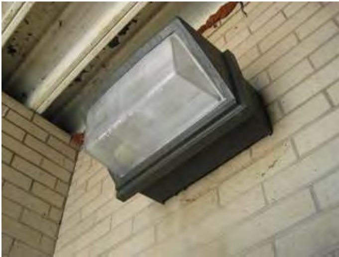
Wall mounted exterior lighting fixture
