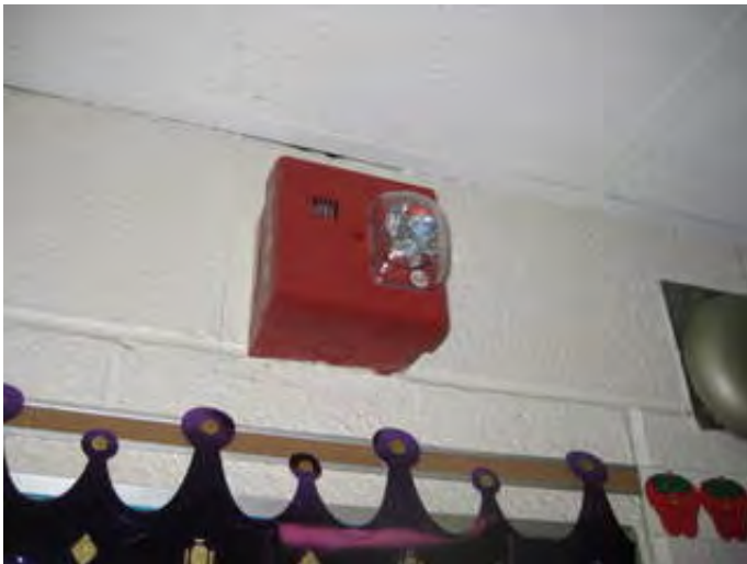
Wall mounted horn strobe device
