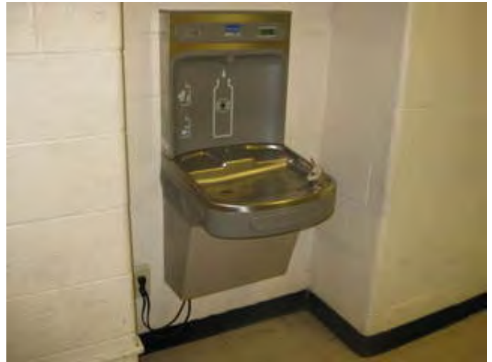
ADA compliant electric water cooler
