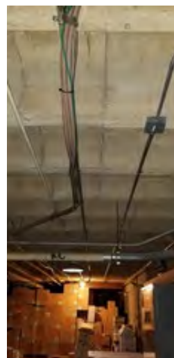
Cast in place concrete floor from mechanical space
