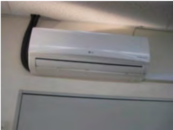
Self contained air-conditioning unit with remote condensing unit
