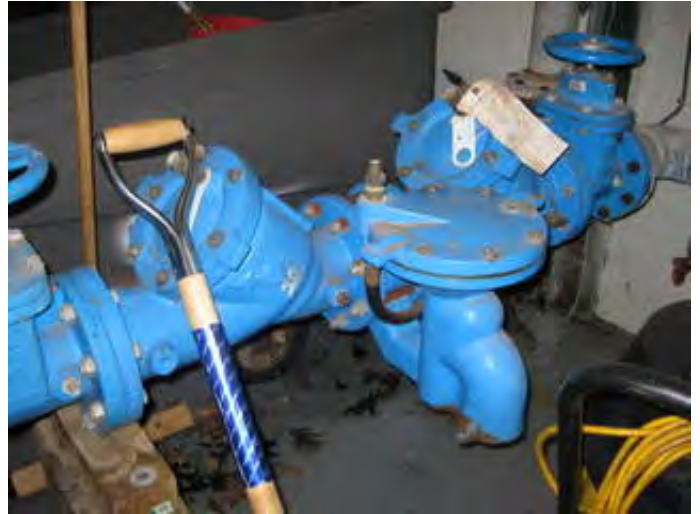
Water service back-flow preventer
