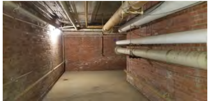
Brick and poured foundation at original construction
