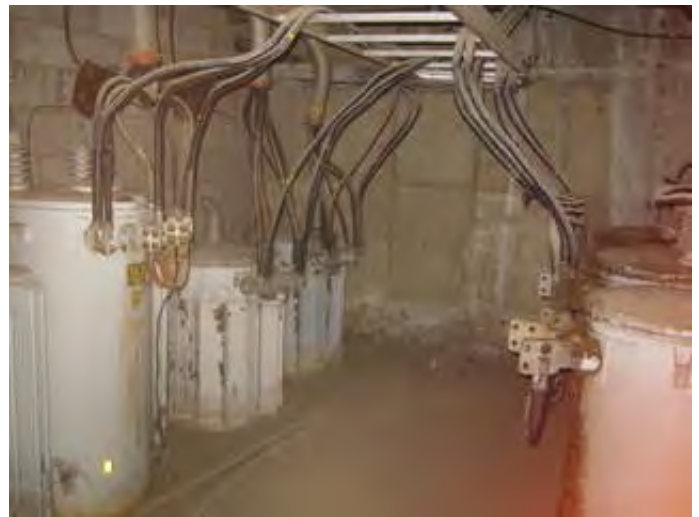
Pad mounted transformers in electrical vault
