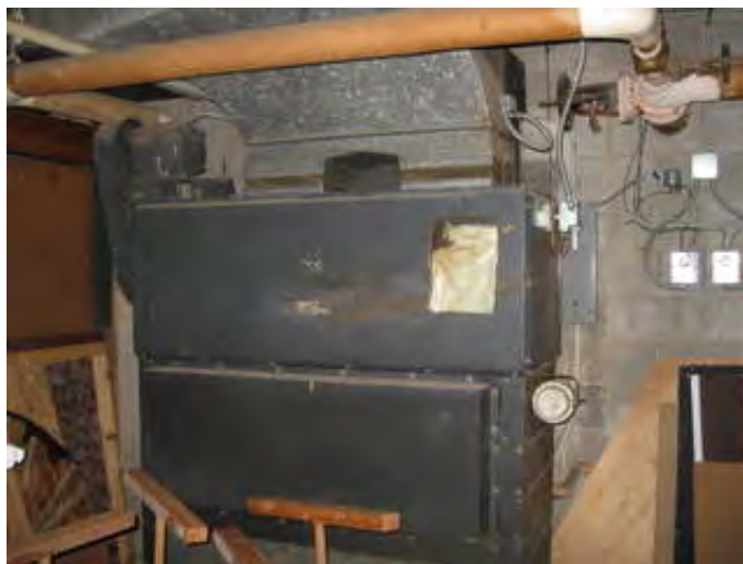
Lower level mechanical room air handling unit
