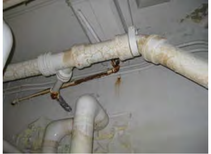
Cast-iron sanitary piping
