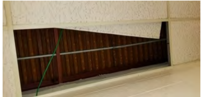
Metal form deck at 1965 addition
