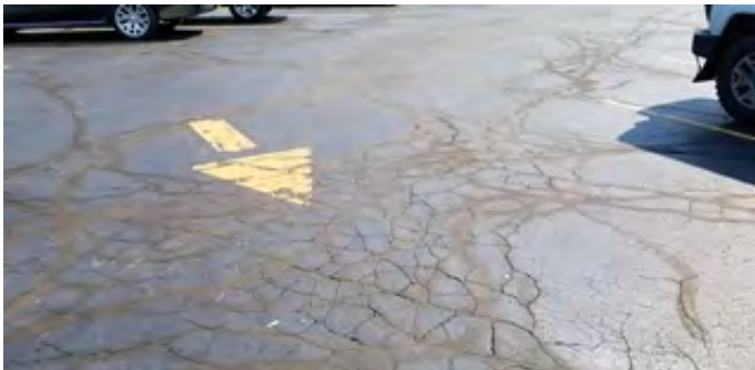
Asphalt pavement in poor condition
