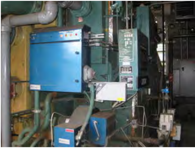
1958 mechanical building absorption chiller
