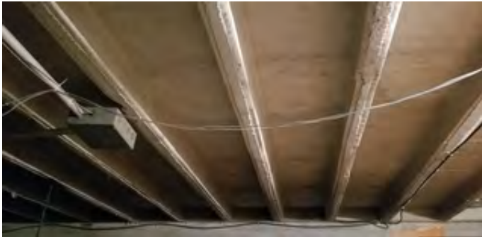
Cast in place concrete at mechanical room
