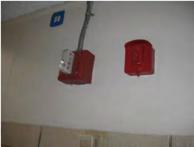
Corridor mounted horn strobe device
