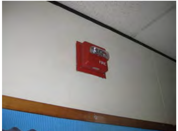
Fire alarm strobe device
