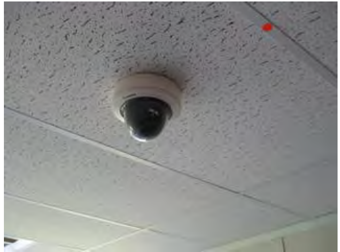
Ceiling mounted security camera
