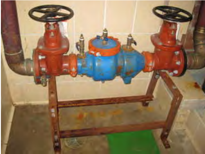
Water service back-flow preventer
