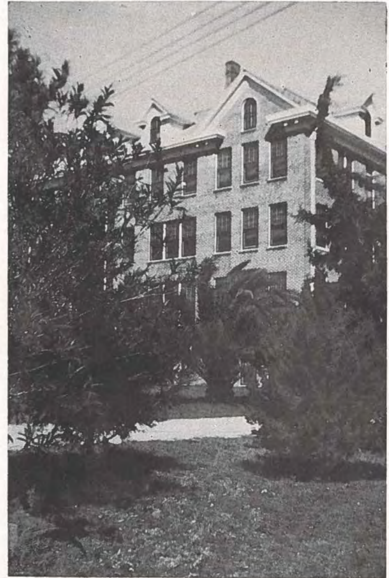
MAIN BUILDING FROM THE SOUTHEAST
