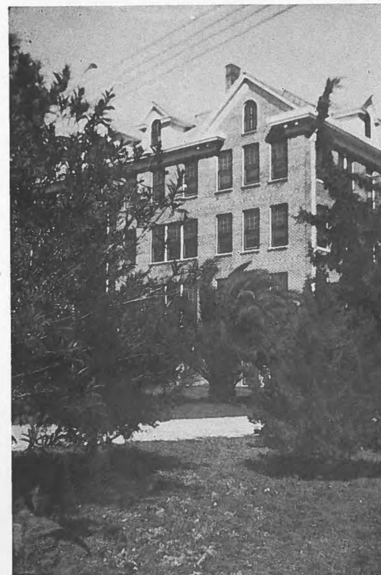
Main Building from the Southeast
