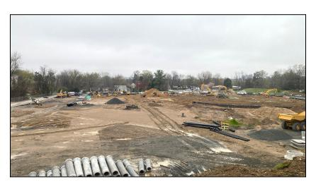
Demolition of the old school structure has been completed, with retaining wall foundations and walls now in place. Additionally, the curb, gutter, and sidewalk along the eastern property line have been installed, while site grading for the future parking area is currently underway.
