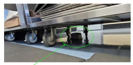
REMOVE FLOOR OUTLETS AND ADD CEILING OUTLET
