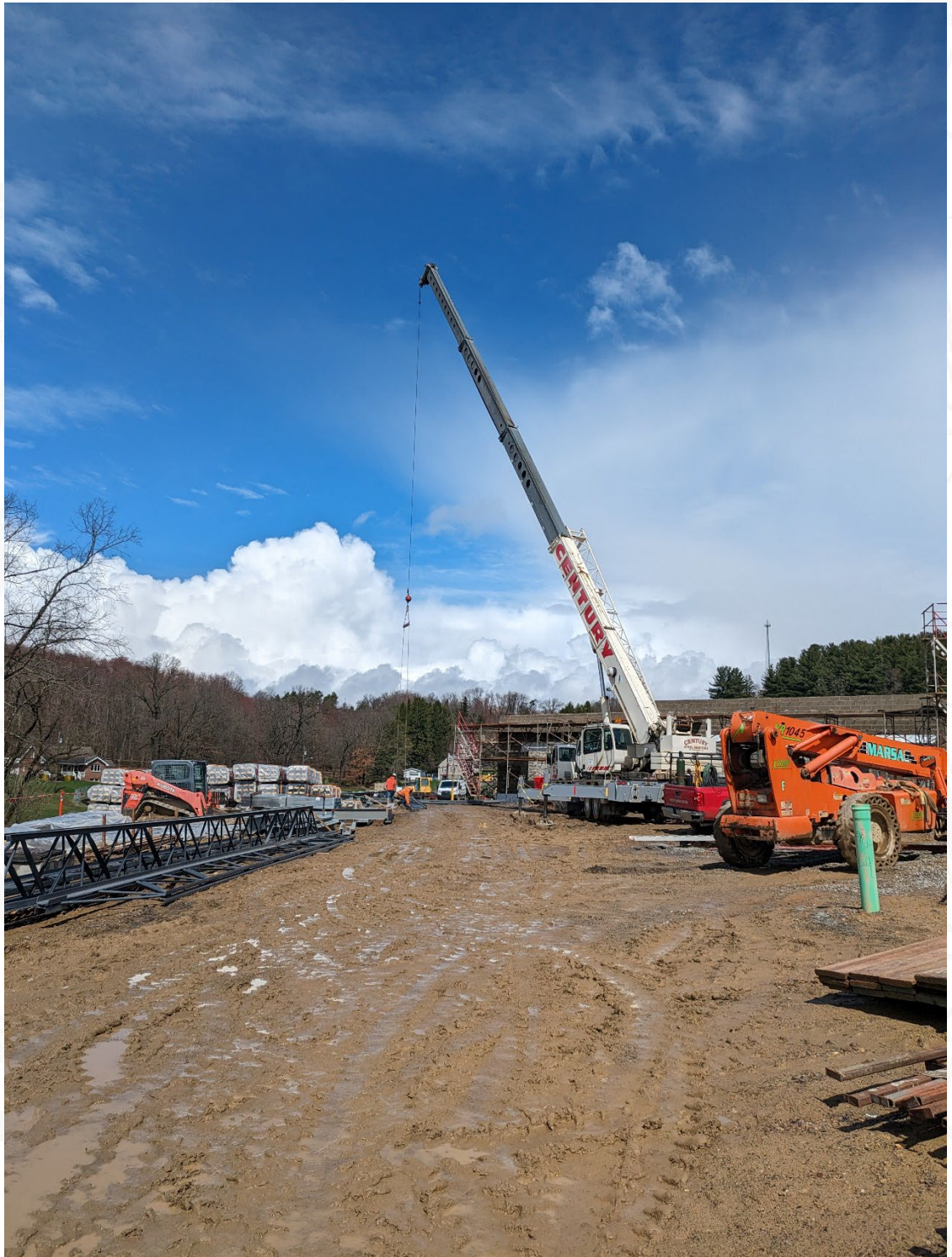
Roof joists being lifted
