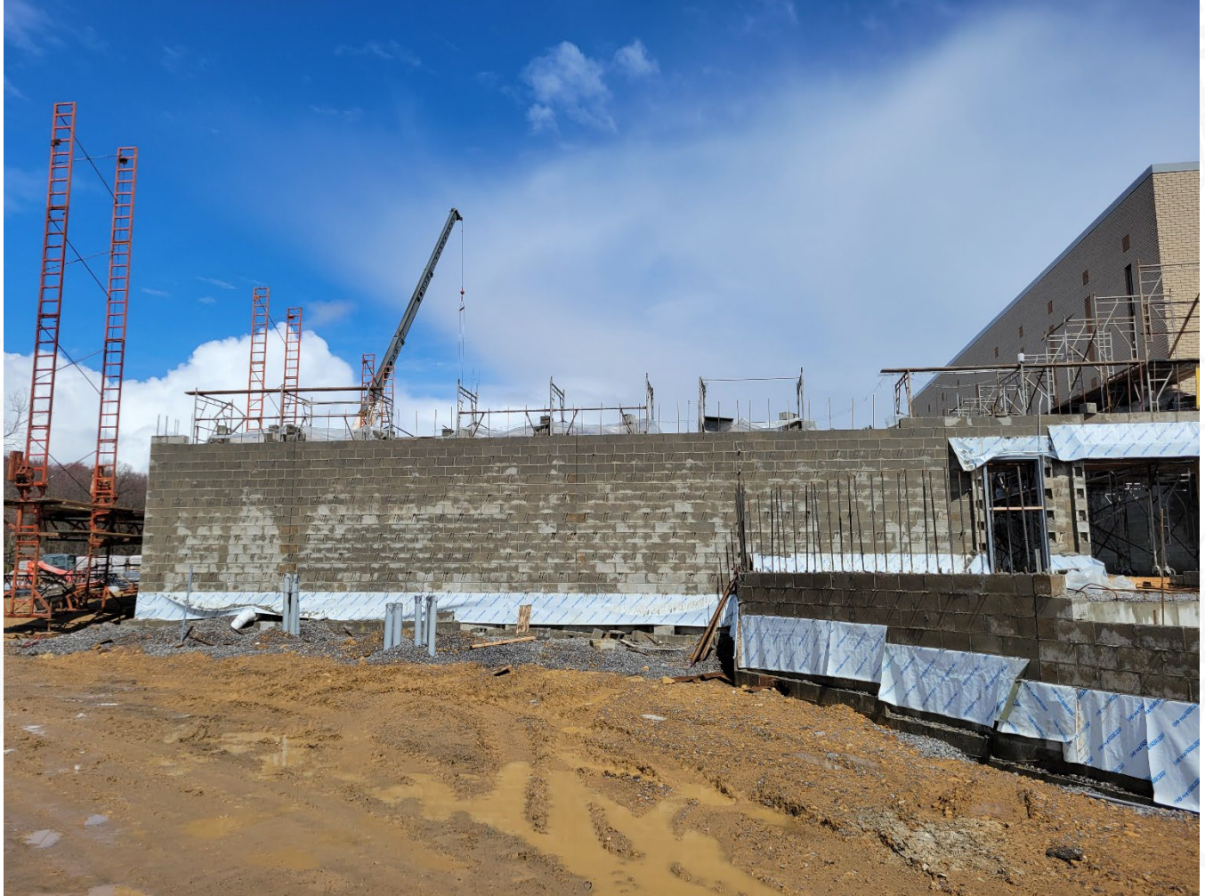
South wall of kitchen/and loading dock. Conduits for new transformer and generator pad are visible in foreground
