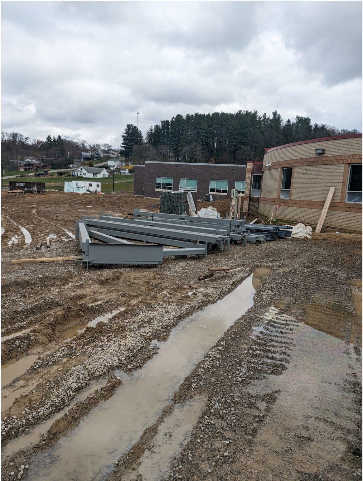
Structural steel for entrance corridor staged for installation
