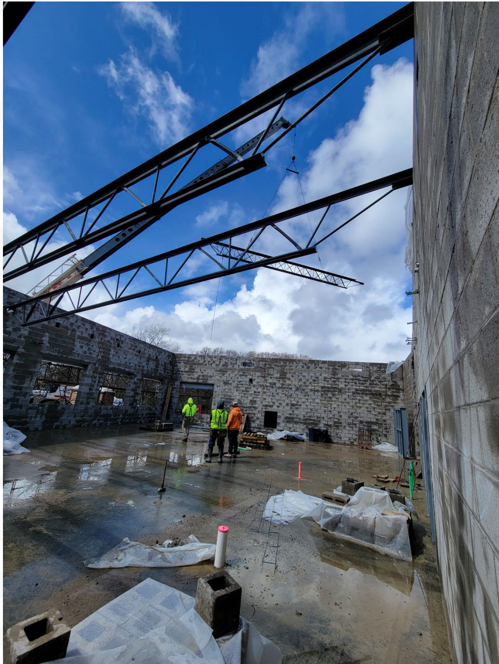
Roof joists being lowered into place
