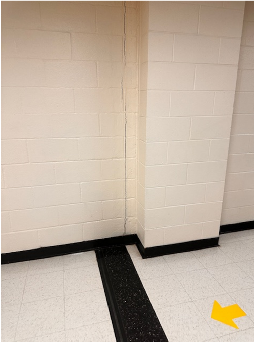
Figure 1 - expansion joint in the floor is covered with vinyl strip while the naturally formed expansion joint in the wall is off-set and formed through CMU block and joints. The abutting pilaster remains in serviceable condition.
