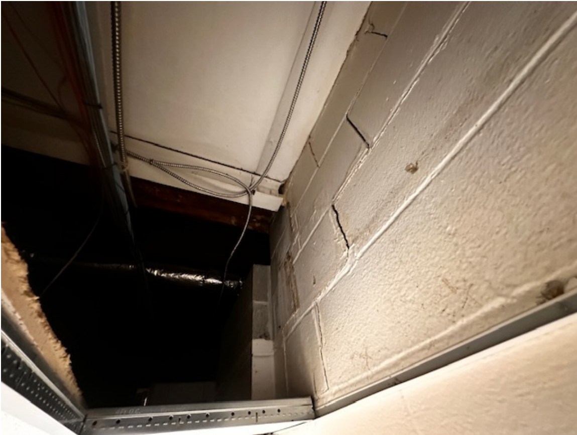
Figure 5 - different angle on Figure 4 where we observed fine hairline cracks around the beam pocket which is consistent with the response of CMU block under seismic loads.
