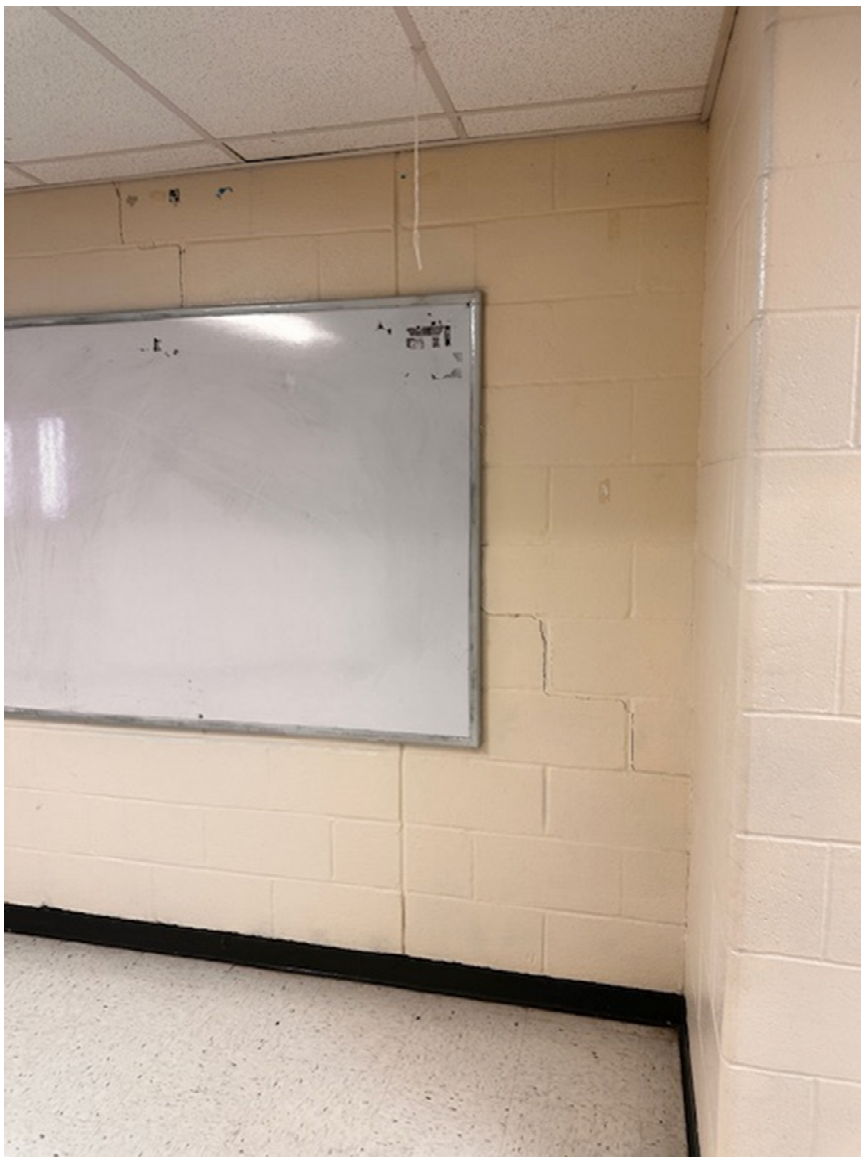
Figure 2 - stepped cracking typical of differential settlement. Note the expansion joint in the wall is not aligned with one in the floor and is not functioning.
