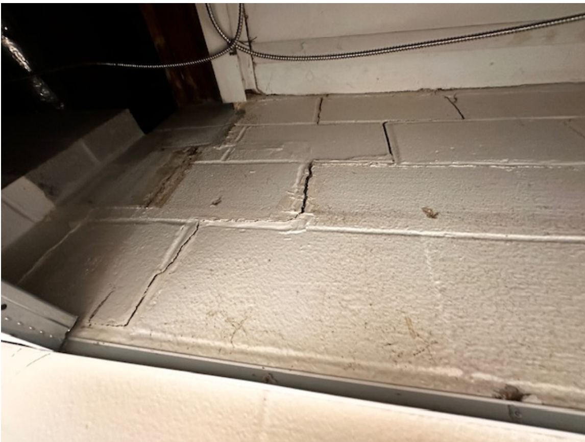
Figure 4 - Uncontrolled cracking above the ceiling in the area of the expansion joint of the sallyport.
