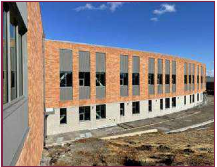
West's new T-Wing, mid-construction.
