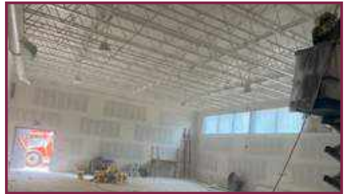
Houck's multi-purpose fitness room being painted.
