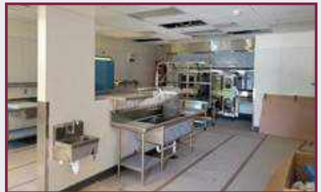
Keizer's kitchen equipment being installed.
