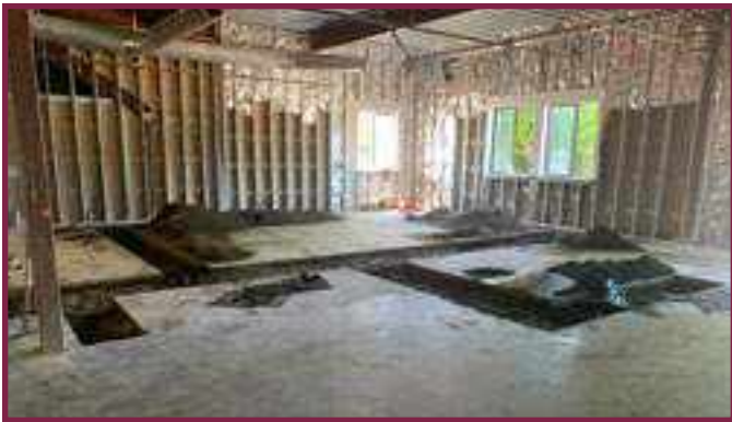
Crossler's new science room renovation.
