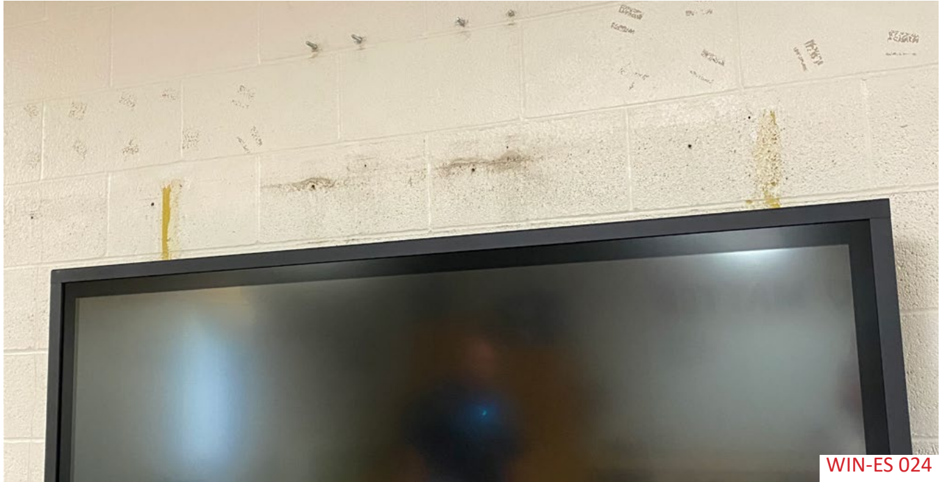
In Room 147C, the CMU paint has patches and could use some.
