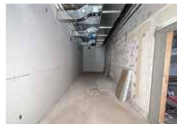
Sheetrock in the gym area has begun.
