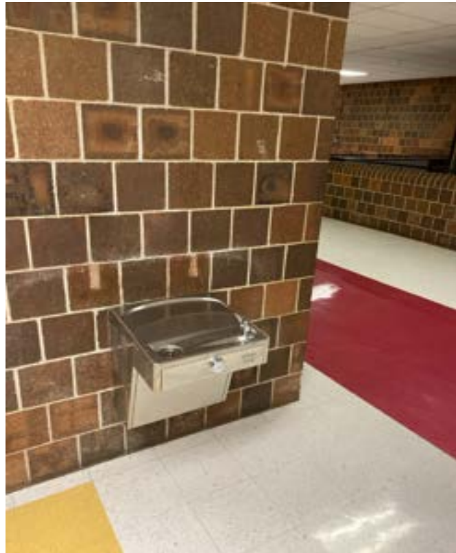
12/22/2023 - 5815-1 - Winnetonka High School - Outside Men's Restroom-Right
