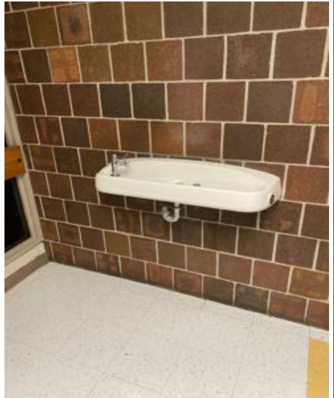
12/22/2023 - 5815-2 - Winnetonka High School - Outside Men's Restroom-Left
