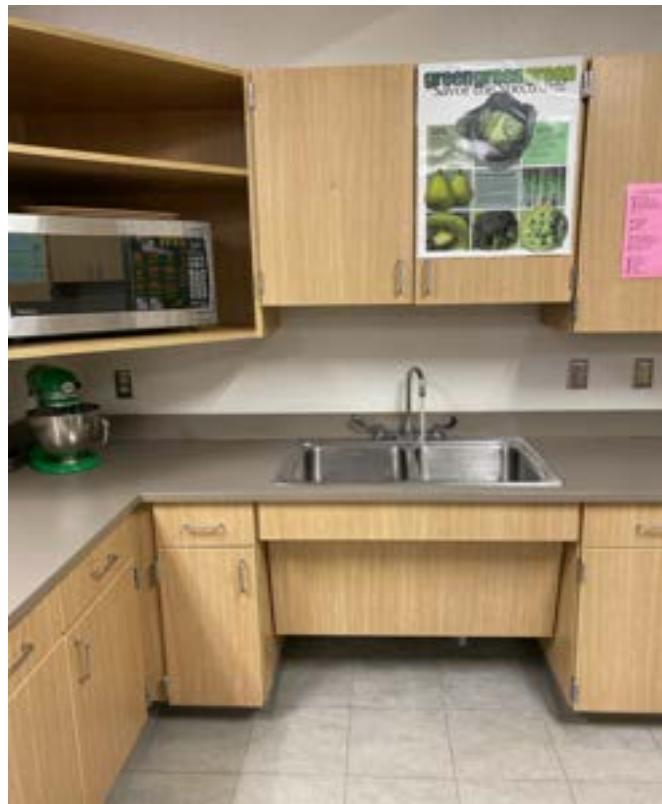
12/22/2023 - 5815-45 - Winnetonka High School - E4-North Wall-West Sink
