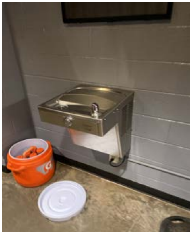
12/22/2023 - 5815-31 - Winnetonka High School - Varsity Locker Room Lower Level
