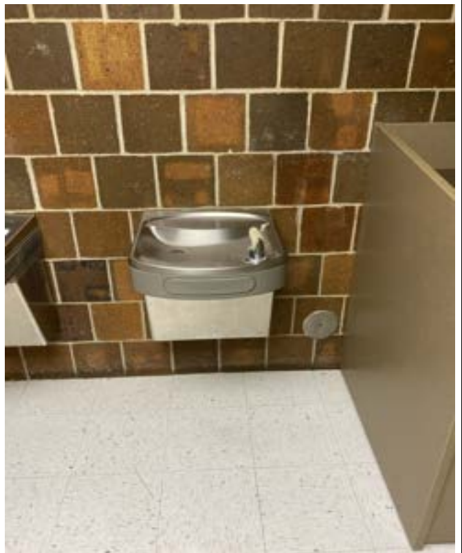
12/22/2023 - 5815-56 - Winnetonka High School - Outside Cafeteria-Right
