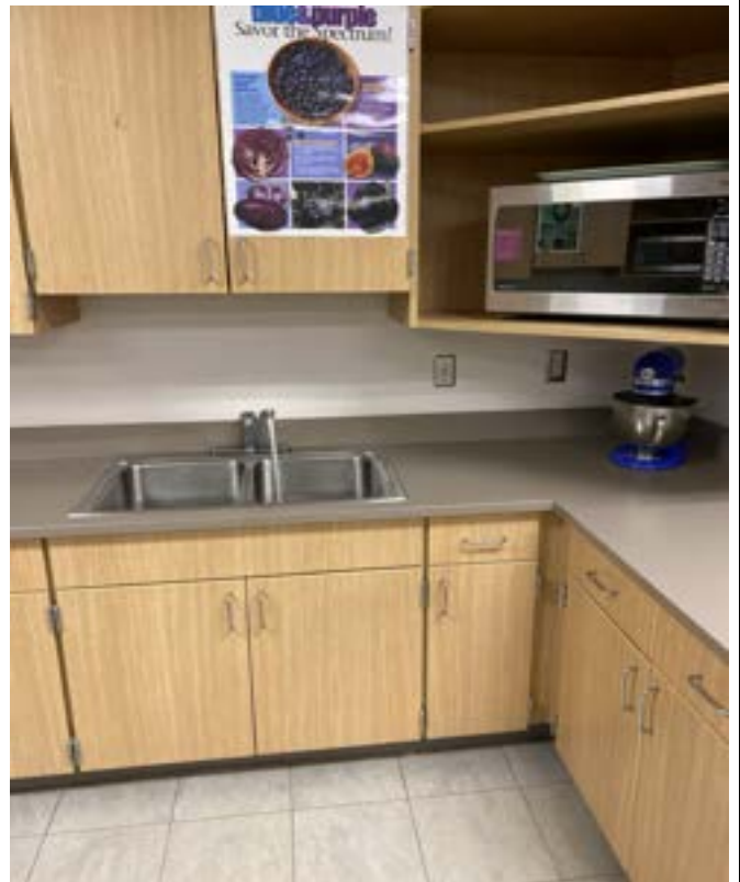
12/22/2023 - 5815-46 - Winnetonka High School - E4-East Wall-North Sink
