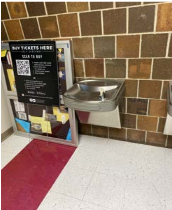
12/22/2023 - 5815-55 - Winnetonka High School - Outside Cafeteria
