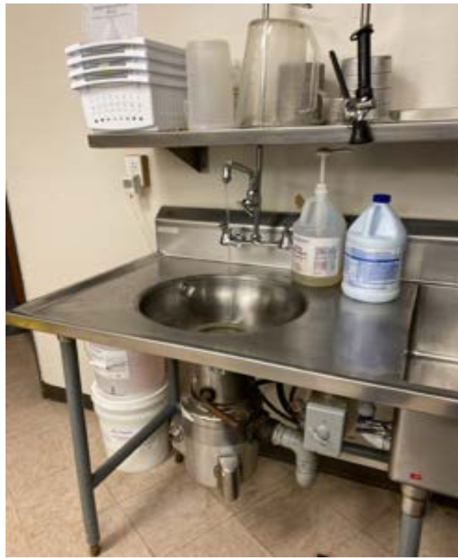
1/15/2024 - 1506-33 - West Englewood Elementary - Kitchen-Northwest Sink
