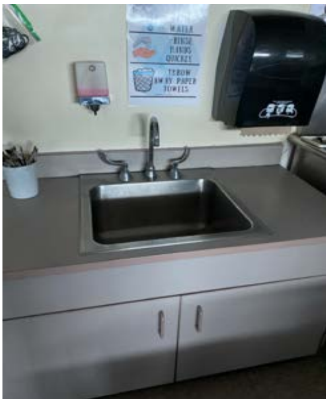
1/15/2024 - 1506-23 - West Englewood Elementary - Room 32-Left
