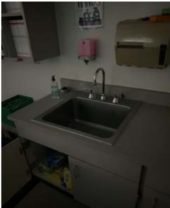
1/15/2024 - 1506-39 - West Englewood Elementary - Room 12
