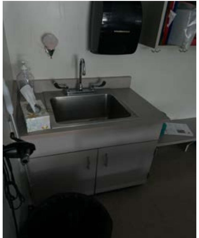
1/15/2024 - 1506-18 - West Englewood Elementary - Room 42
