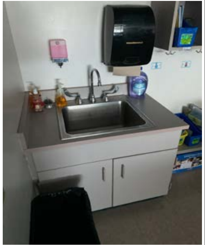
1/15/2024 - 1506-14 - West Englewood Elementary - Room 41
