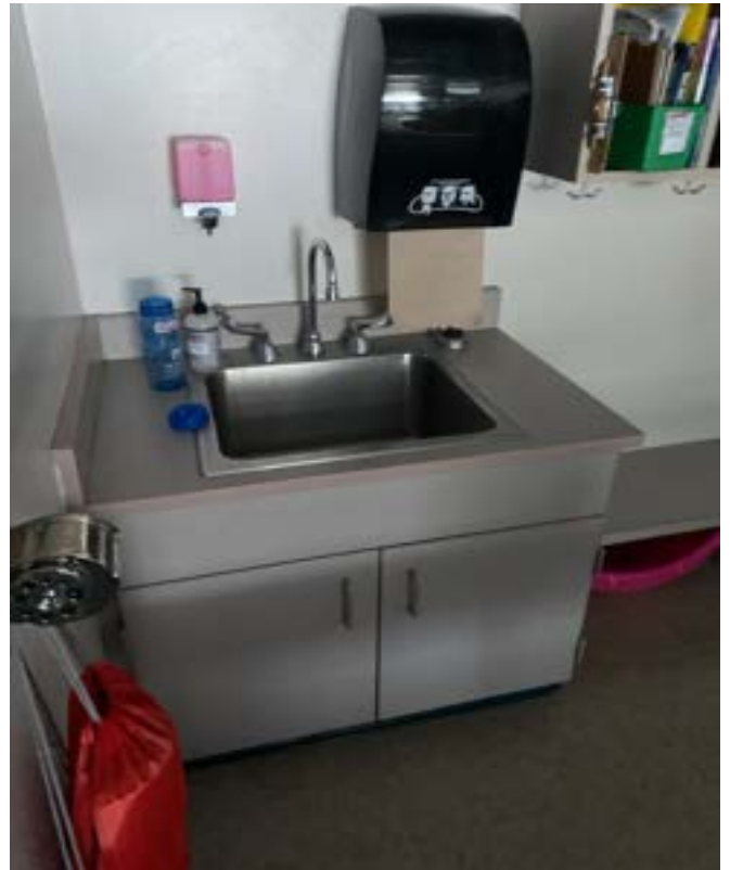
1/15/2024 - 1506-22 - West Englewood Elementary - Room 34
