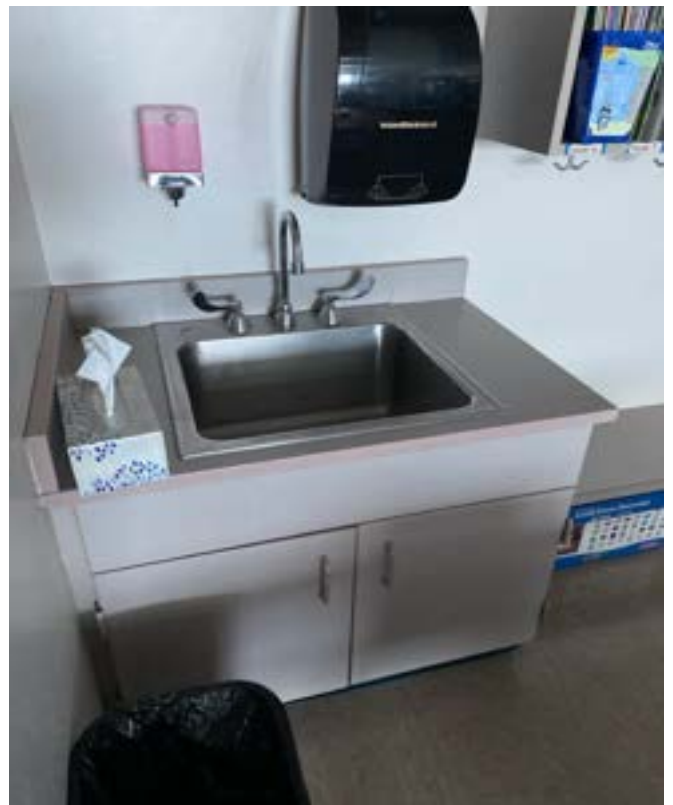
1/15/2024 - 1506-12 - West Englewood Elementary - Room 37
