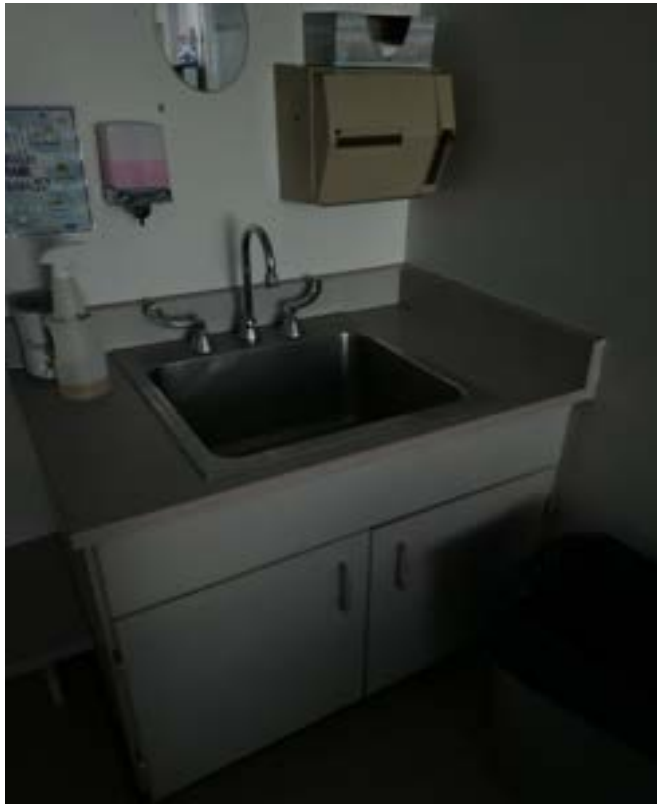
1/15/2024 - 1506-13 - West Englewood Elementary - Room 39
