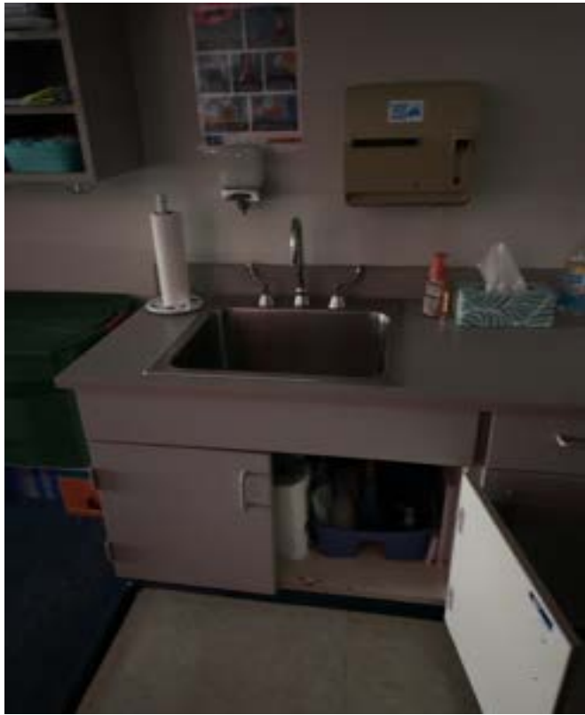
1/15/2024 - 1506-5 - West Englewood Elementary - Room 24
