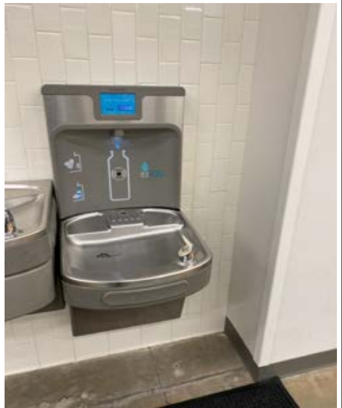
1/8/2024 - 7301-32 - Rising Hill Elementary - Cafeteria-Right
