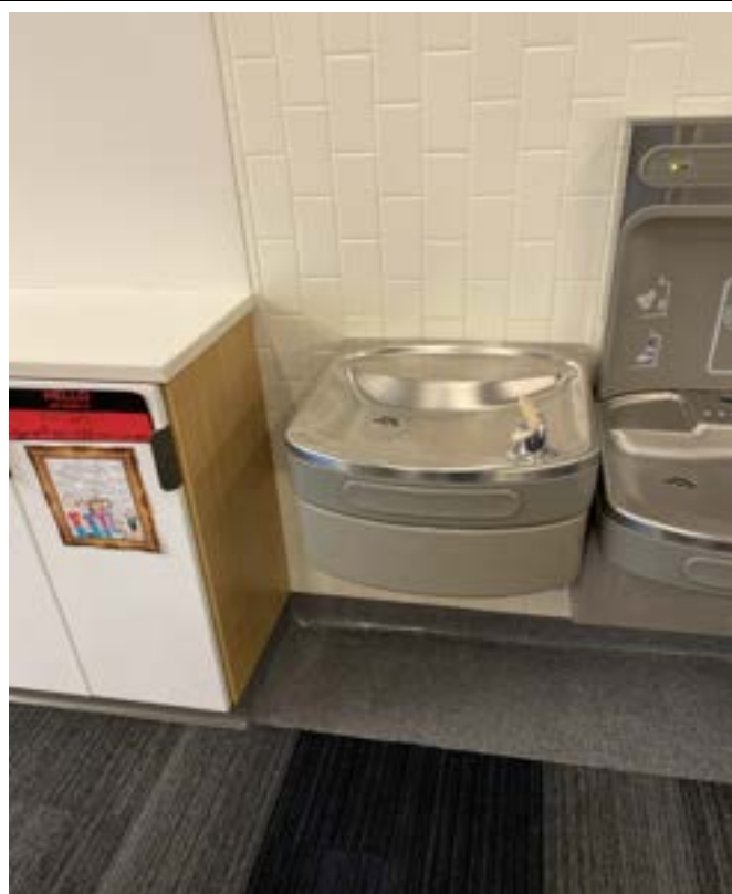
1/8/2024 - 7301-27 - Rising Hill Elementary - Outside 231-Left
