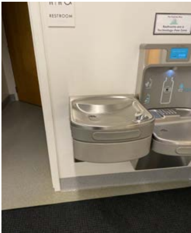
1/8/2024 - 7301-19 - Rising Hill Elementary - Outside 210-Left
