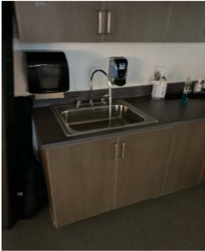
1/8/2024 - 7301-17 - Rising Hill Elementary - Room 201
