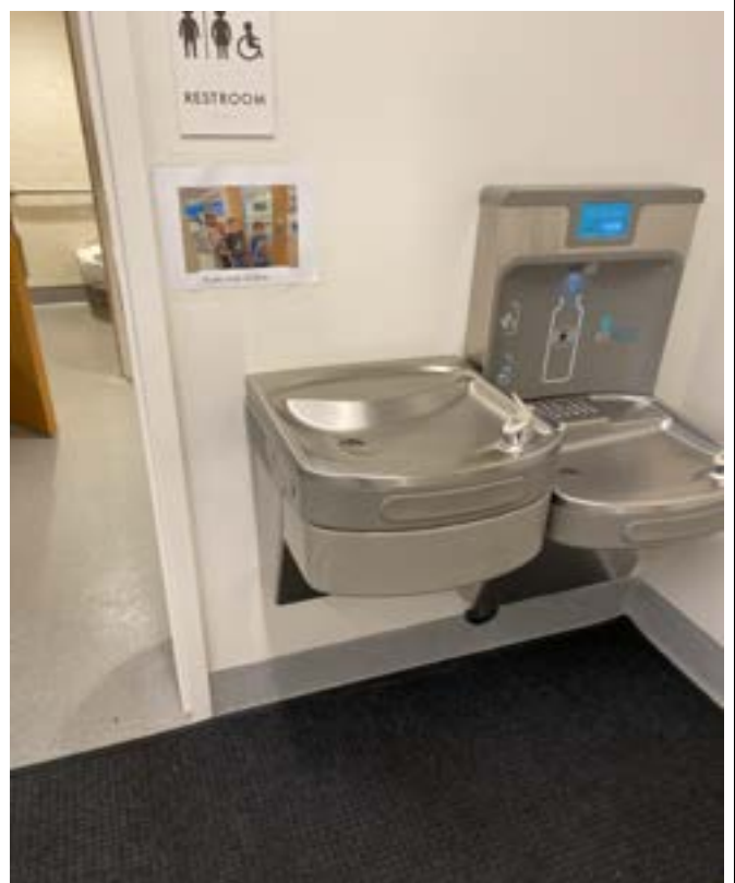
1/8/2024 - 7301-14 - Rising Hill Elementary - Outside 149-Left
