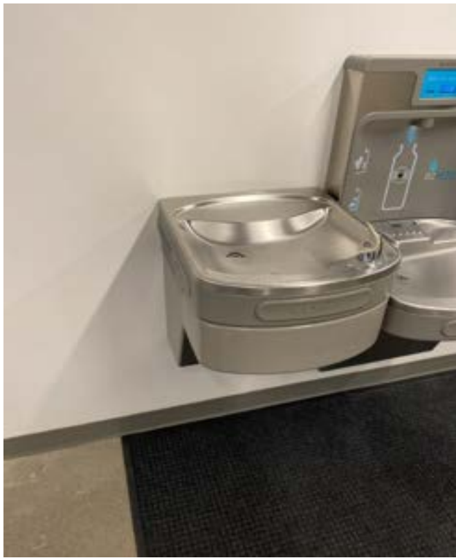
1/8/2024 - 7301-29 - Rising Hill Elementary - Outside 125-Left
