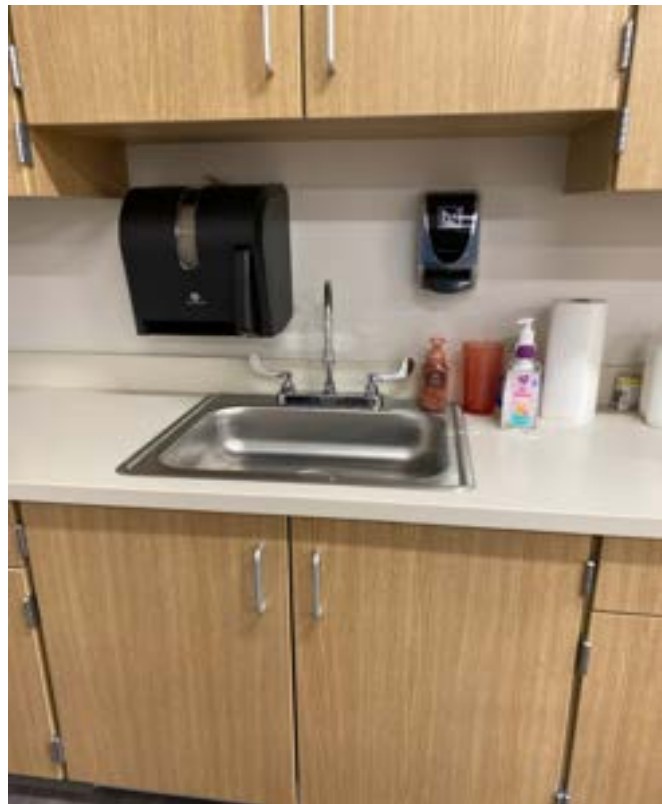
1/8/2024 - 7301-5 - Rising Hill Elementary - Room 171
