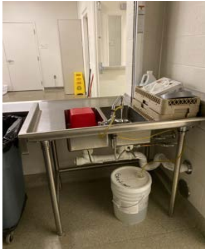
1/8/2024 - 7301-33 - Rising Hill Elementary - Kitchen-Closest to Cafe
