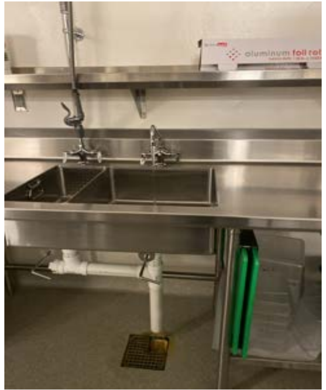
1/8/2024 - 7301-38 - Rising Hill Elementary - Kitchen-East Wall Sink
