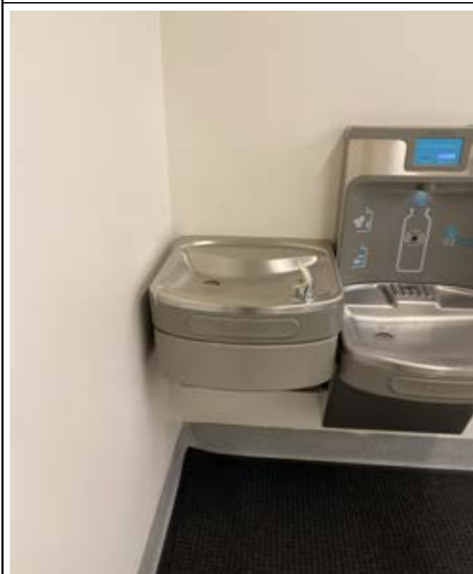
1/8/2024 - 7301-11 - Rising Hill Elementary - Outside 153-Left
