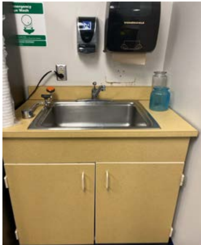
1/15/2024 - 515-1 - New Mark Middle School - Room 100
