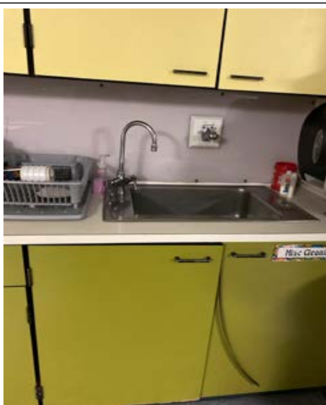
1/15/2024 - 515-14 - New Mark Middle School - Room 504
