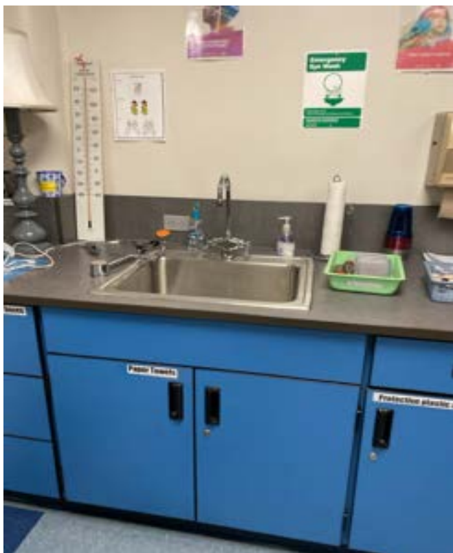
1/15/2024 - 515-39 - New Mark Middle School - Room 511-Furthest from Door
