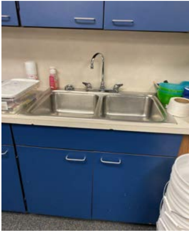
1/15/2024 - 515-29 - New Mark Middle School - Room 500
