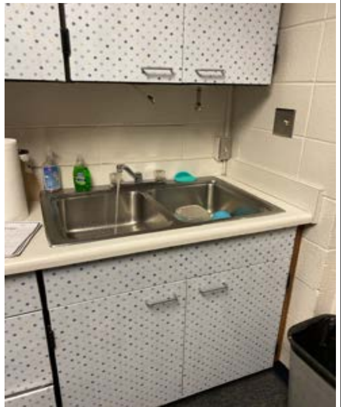
1/15/2024 - 515-32 - New Mark Middle School - Room 508
