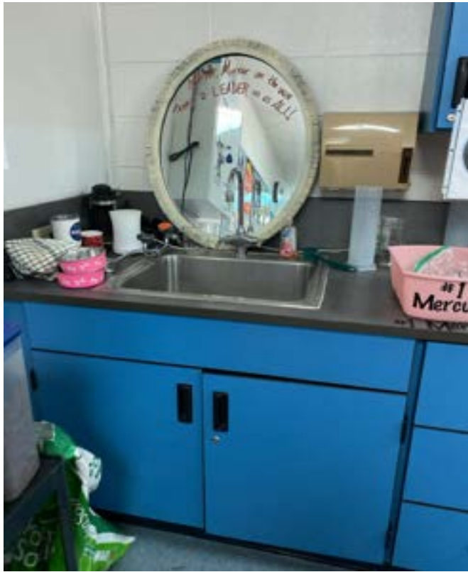
1/15/2024 - 515-45 - New Mark Middle School - Room 514
