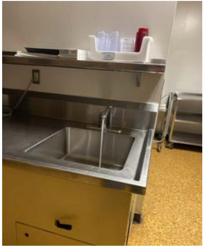
1/15/2024 - 515-54 - New Mark Middle School - Kitchen-By Ice Machine
