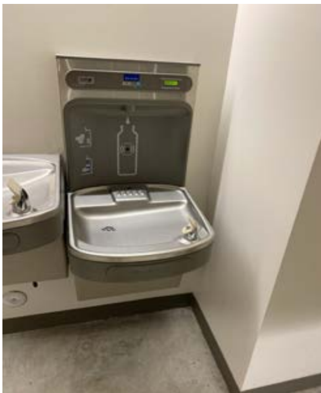
12/21/2023 - 620-15 - NKC High School - Restrooms by A304- Right
