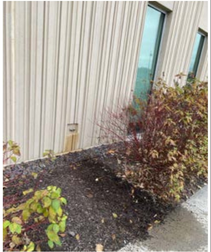
12/21/2023 - 620-87 - NKC High School - North of Exit Door 18
