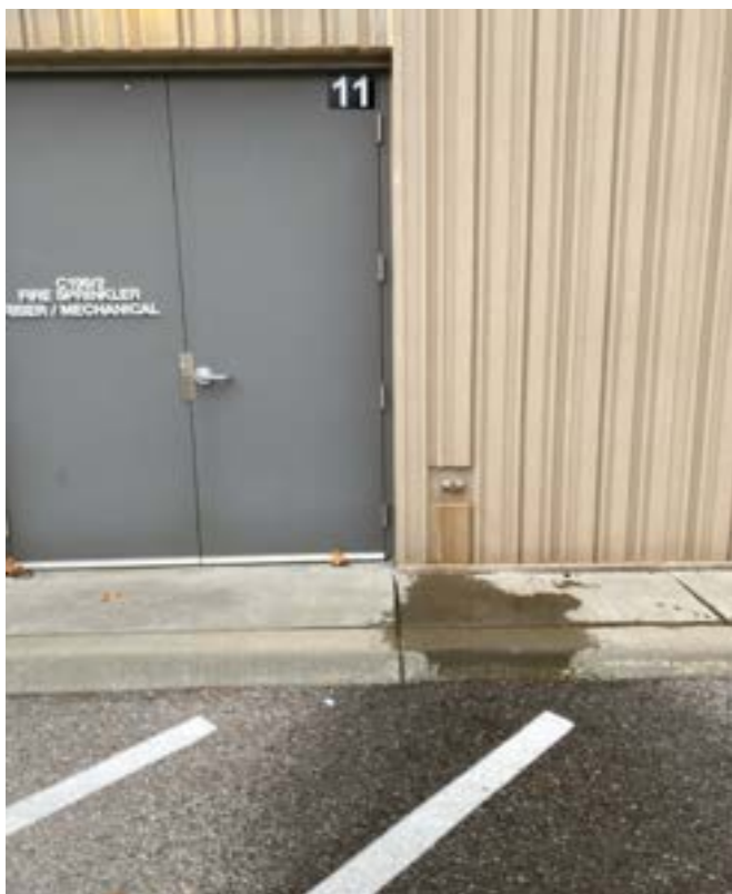
12/21/2023 - 620-84 - NKC High School - By Exit Door 11
