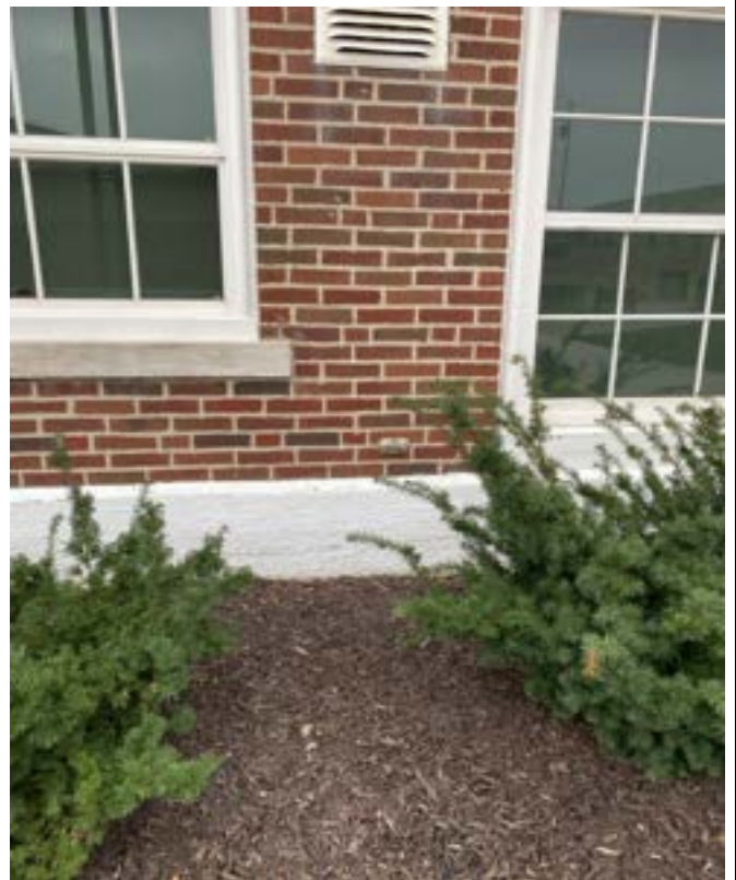
12/21/2023 - 620-89 - NKC High School - West of Exit Door 20
