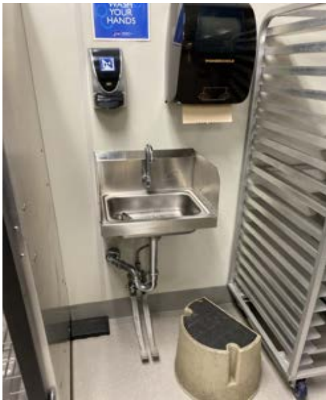
12/21/2023 - 620-67 - NKC High School - Kitchen- Northwest Sink
