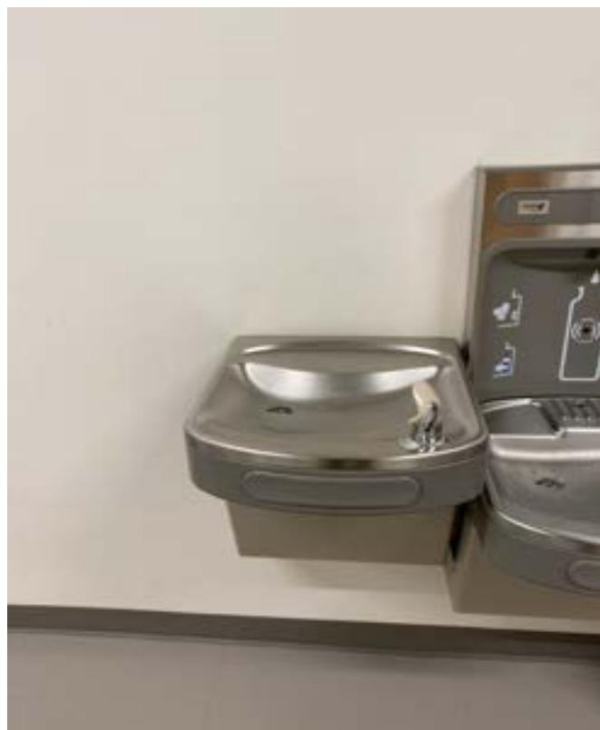
12/21/2023 - 620-27 - NKC High School - Outside M239-Left
