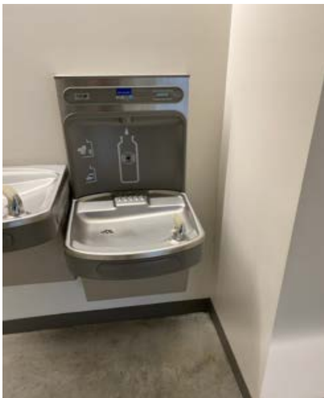
12/21/2023 - 620-47 - NKC High School - Restrooms Outside A102-Right
