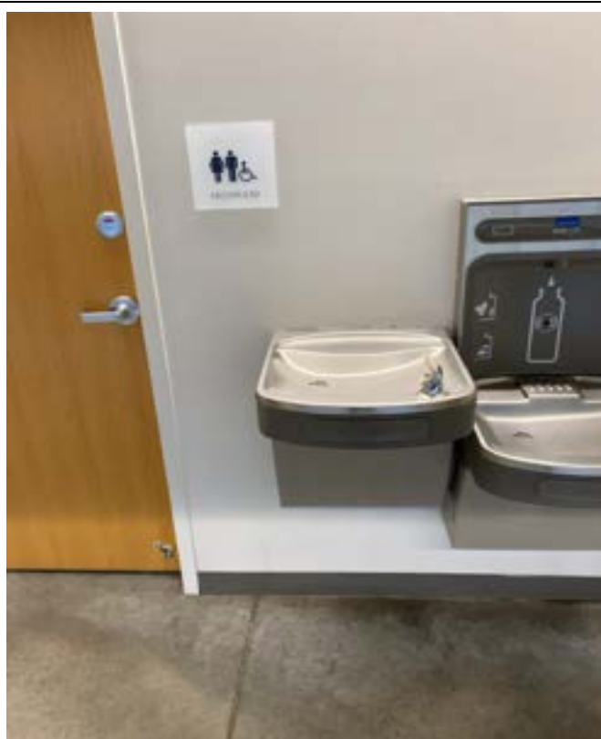
12/21/2023 - 620-60 - NKC High School - Restrooms by Cafe-Left
