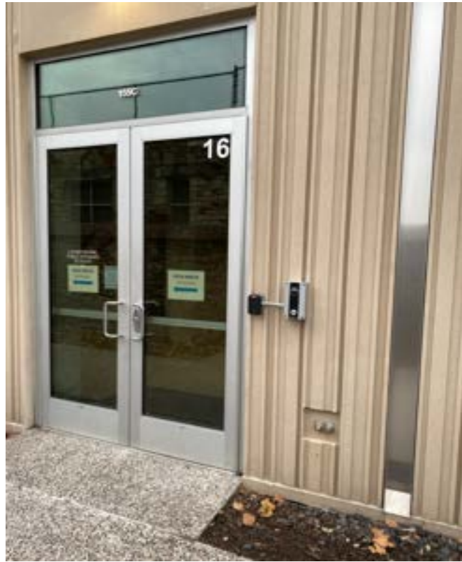
12/21/2023 - 620-86 - NKC High School - Outside Exit Door 16
