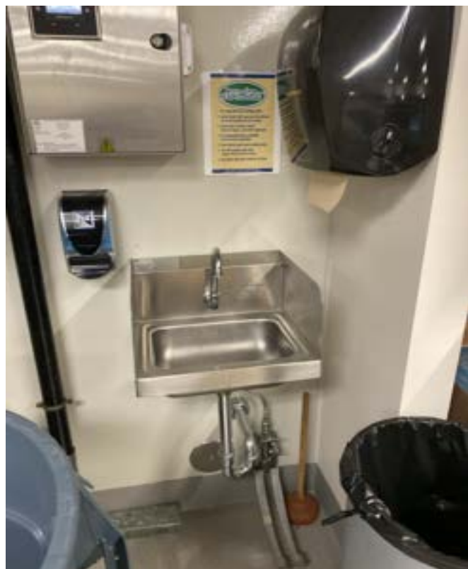
12/21/2023 - 620-71 - NKC High School - Kitchen- Northeast Handwashing Sink
