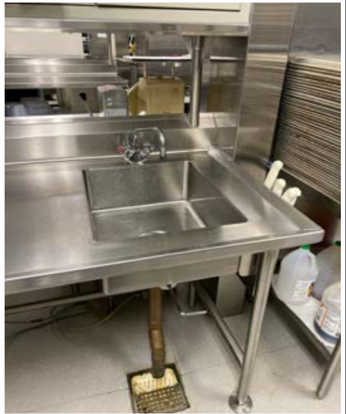
12/21/2023 - 620-66 - NKC High School - Kitchen- West Sink
