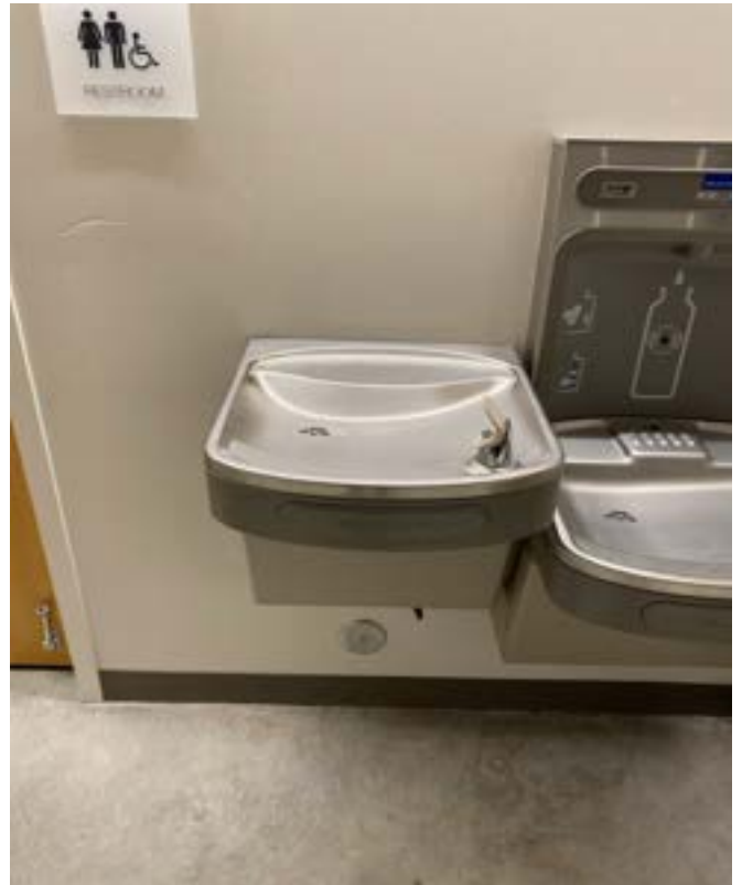
12/21/2023 - 620-14 - NKC High School - Restrooms by A304- Left
