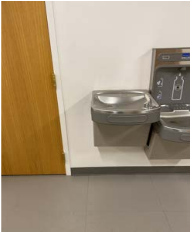
12/21/2023 - 620-29 - NKC High School - Outside M112-Left
