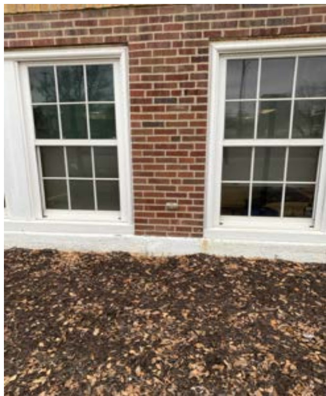
12/21/2023 - 620-90 - NKC High School - North of Exit Door 21
