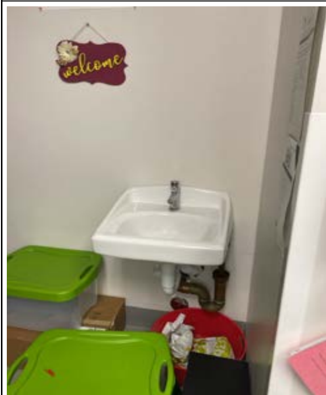
12/21/2023 - 620-59 - NKC High School - B145- North Sink
