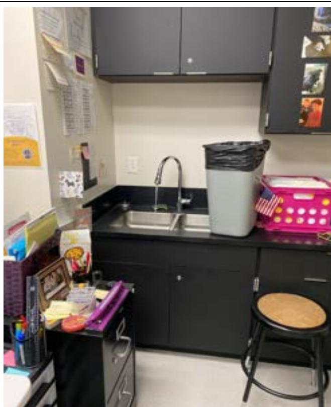
12/21/2023 - 620-58 - NKC High School - B145- Northwest Sink
