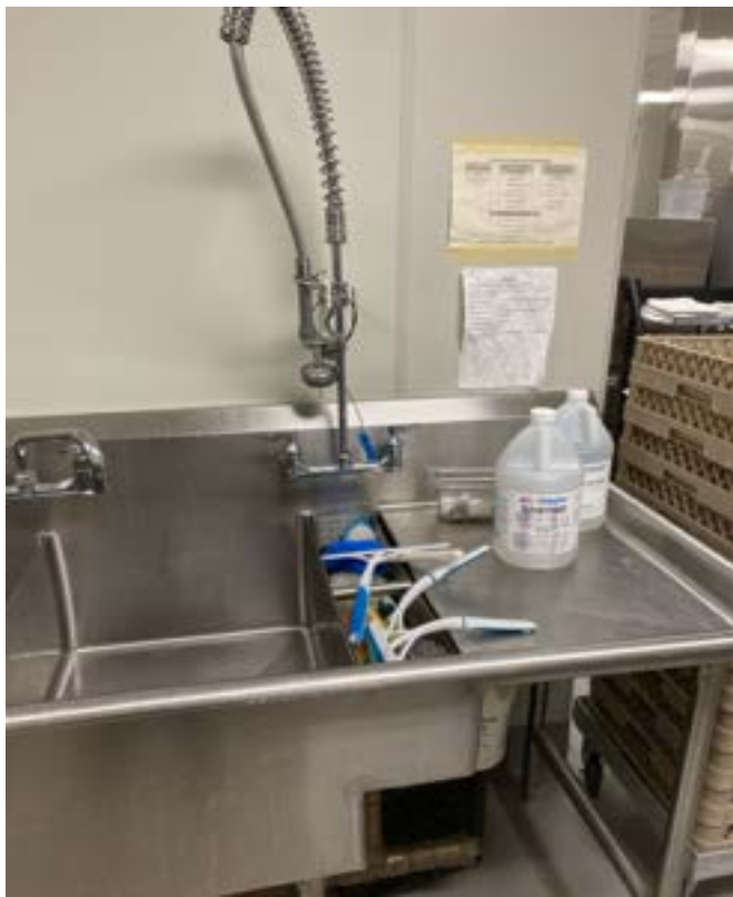
12/21/2023 - 620-63 - NKC High School - Kitchen- Three Bay Sink Right
