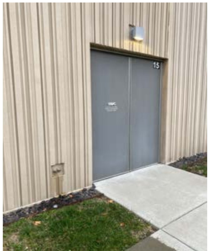
12/21/2023 - 620-85 - NKC High School - By Exit Door 15
