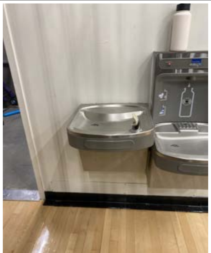
01/02/2024 - 620-93 - NKC High School - Gym-West-Left
