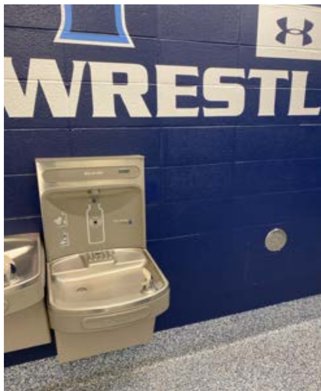
12/26/2023 - 825-71 - Oak Park High School - Men's Locker Room by Main Gym-Right
