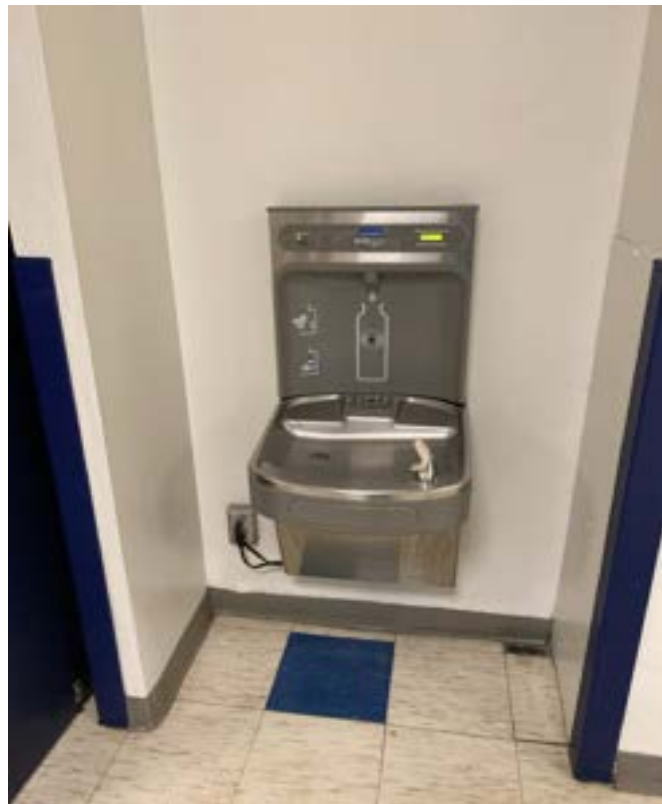
12/26/2023 - 825-45 - Oak Park High School - Outside Training Room-Left
