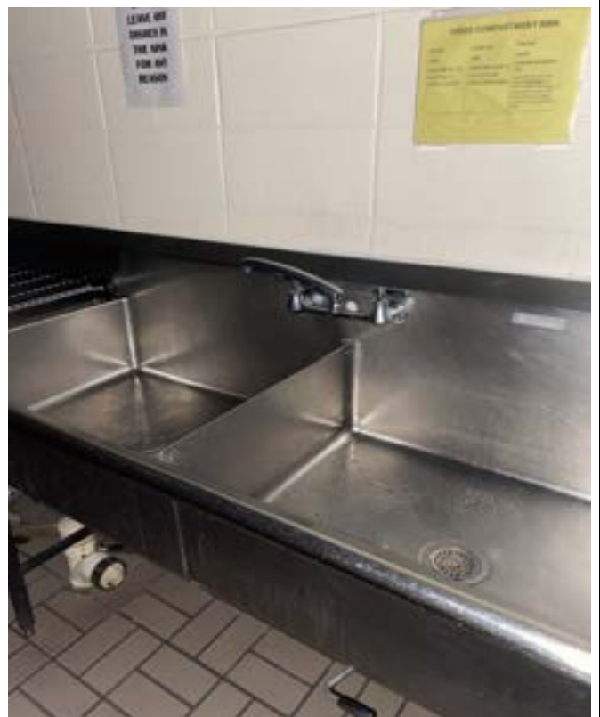
12/26/2023 - 825-56 - Oak Park High School - Kitchen-Northwest Wall-Left Middle
