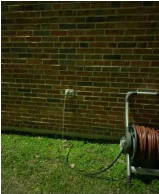
12/26/2023 - 825-77 - Oak Park High School - By Exit Door 21
