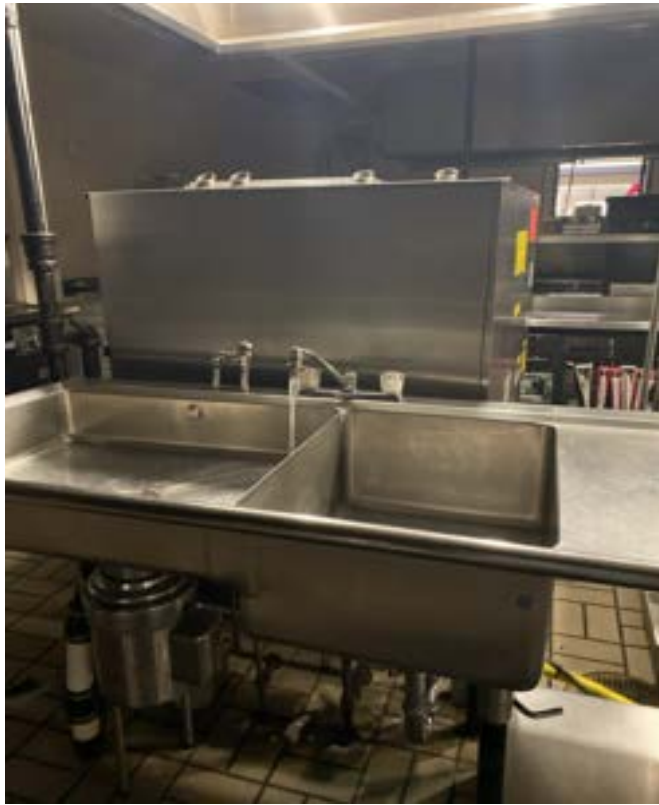
12/26/2023 - 825-53 - Oak Park High School - Kitchen-North Middle Sink
