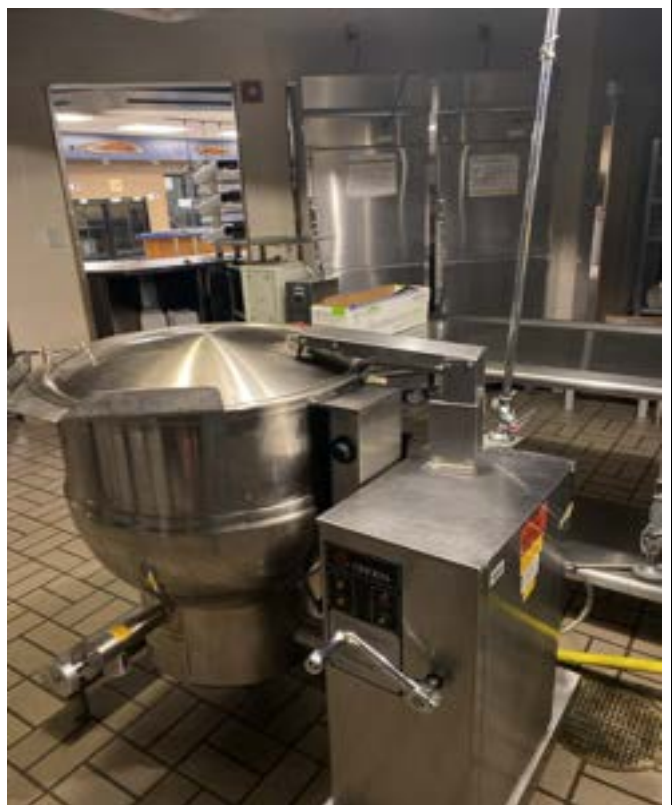
12/26/2023 - 825-52 - Oak Park High School - Kitchen
