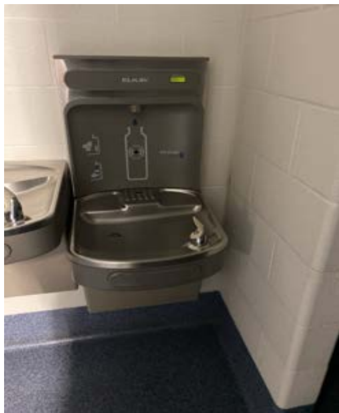
12/26/2023 - 825-69 - Oak Park High School - Men's Locker Room by Main Gym-Right (Restrooms)
