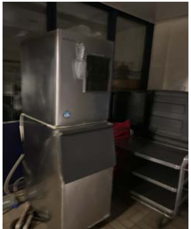
12/26/2023 - 825-60 - Oak Park High School - Kitchen
