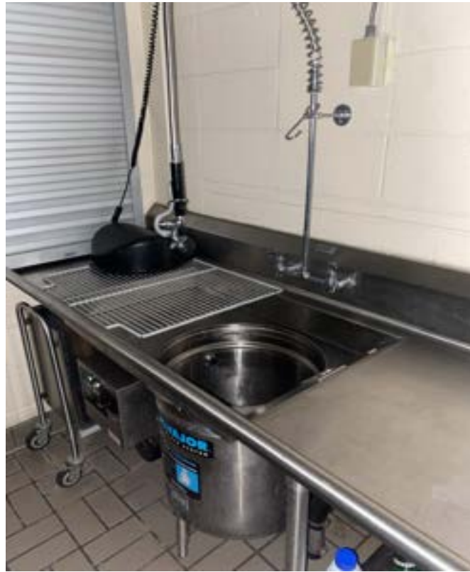
12/26/2023 - 825-57 - Oak Park High School - Kitchen-Northwest Wall-Far Left
