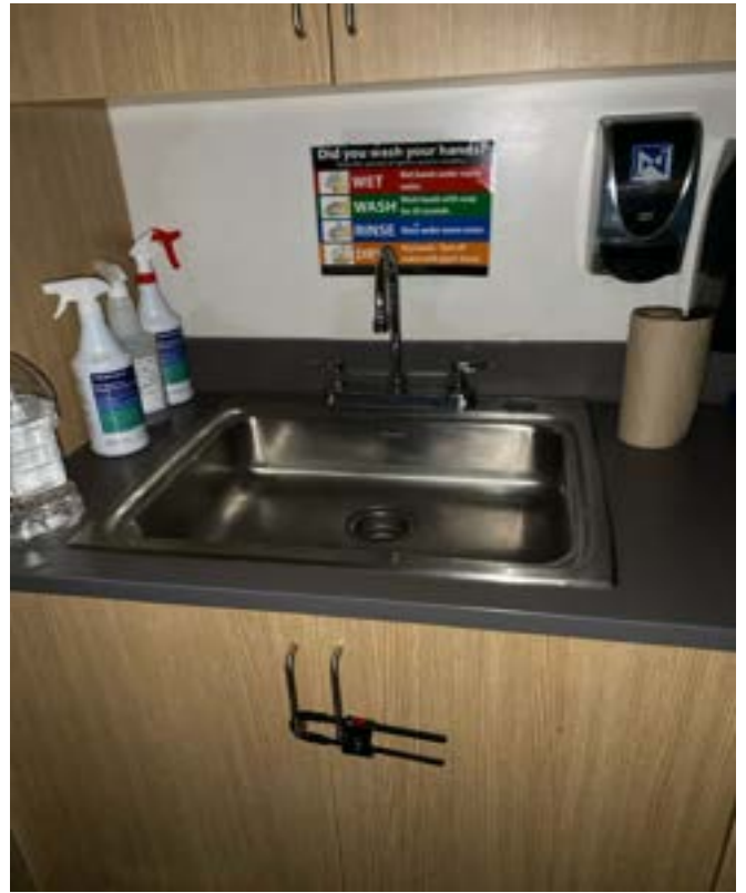
1/16/2024 - 3901-6 - Northview Elementary - Room 163-Left
