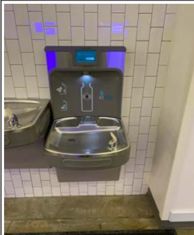
1/16/2024 - 3901-35 - Northview Elementary - Cafeteria-Right
