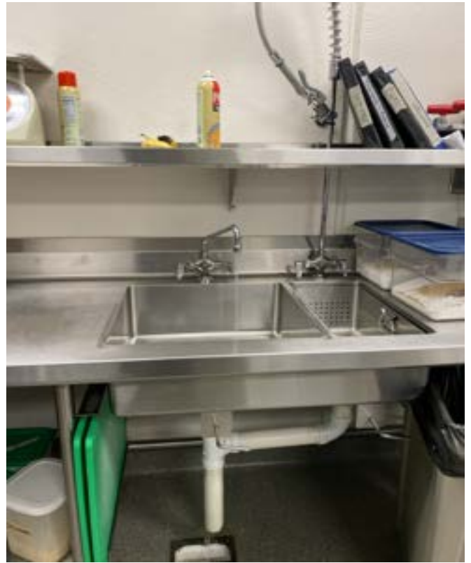
1/16/2024 - 3901-30 - Northview Elementary - Kitchen-South Wall
