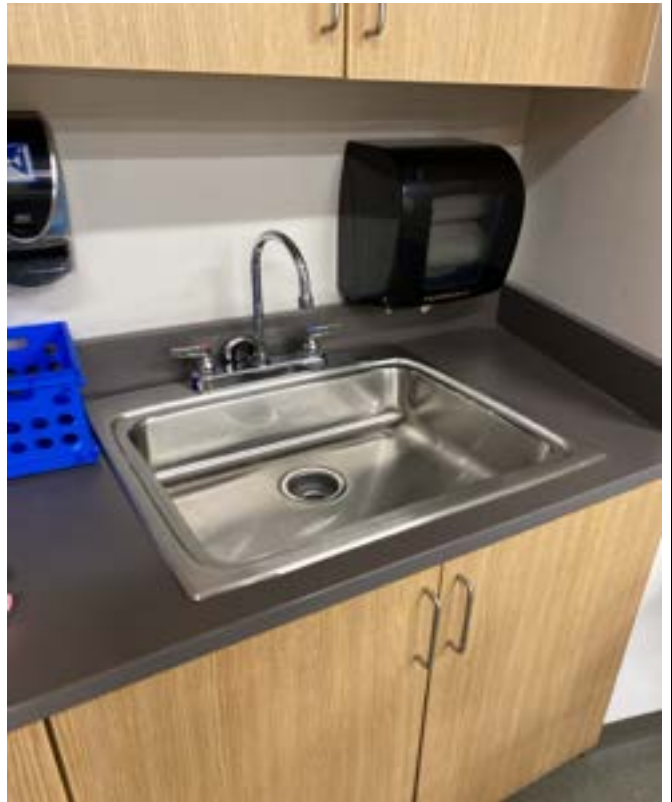
1/16/2024 - 3901-14 - Northview Elementary - Room 201
