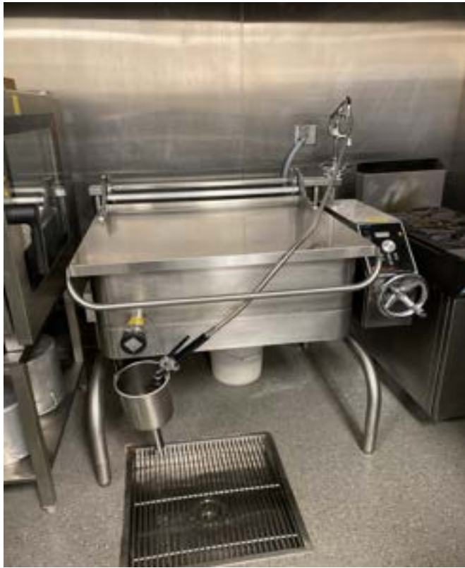
1/16/2024 - 3901-29 - Northview Elementary - Kitchen
