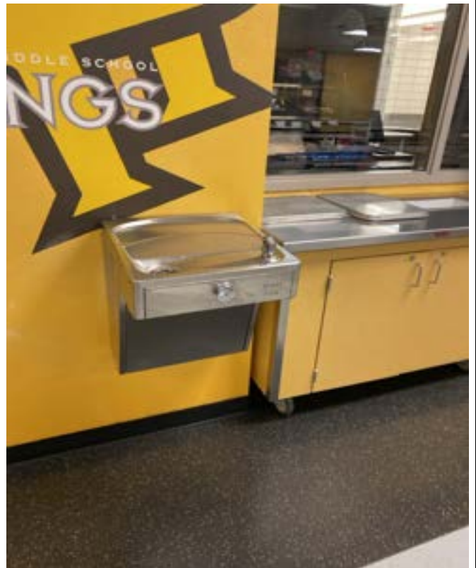
1/17/2024 - 5300-10 - Maple Park Middle School - Cafeteria-Left
