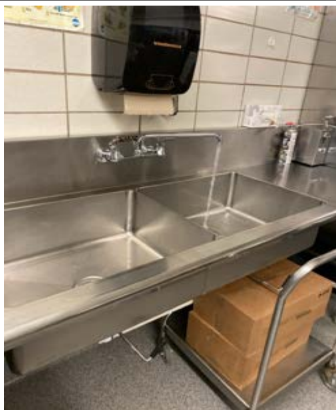
1/17/2024 - 5300-15 - Maple Park Middle School - Kitchen-East Wall Sink
