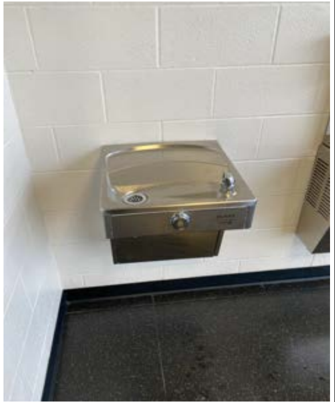
1/17/2024 - 5300-2 - Maple Park Middle School - Outside Room 119
