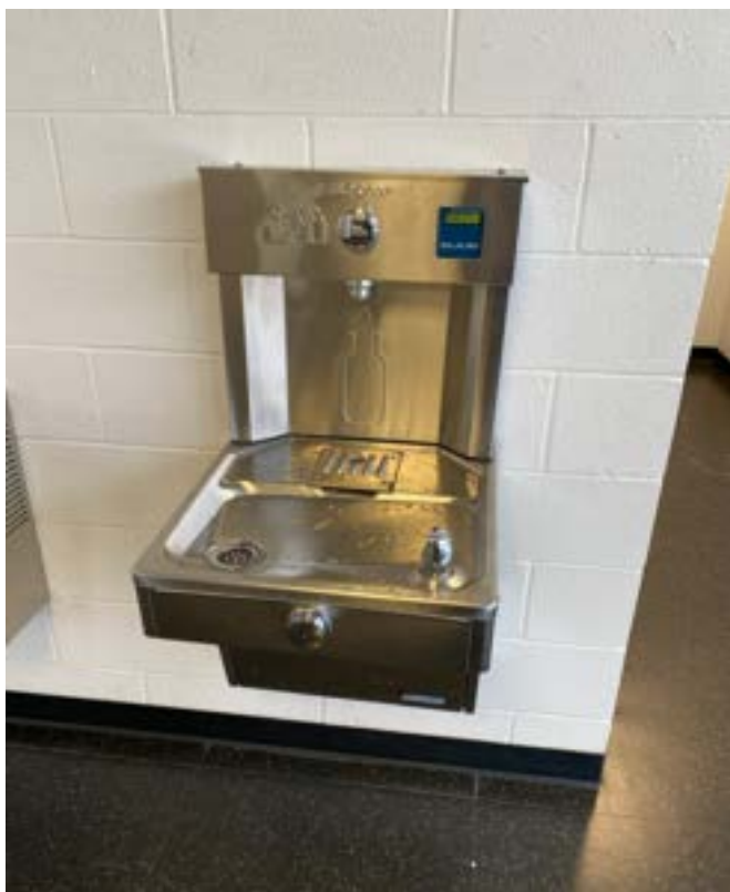
1/17/2024 - 5300-3 - Maple Park Middle School - Outside Room 119
