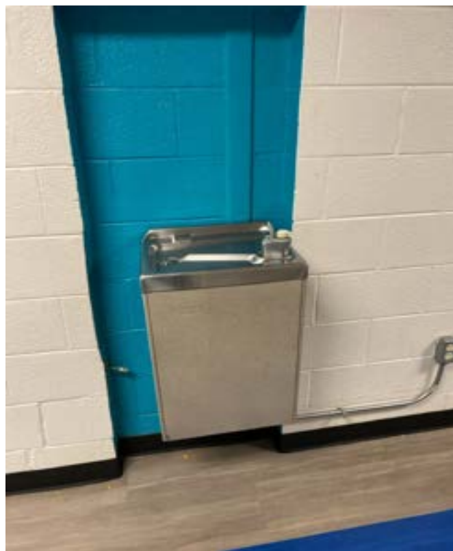
1/11/2024 - 7333-35 - Linden West Elementary - Outside Room 18
