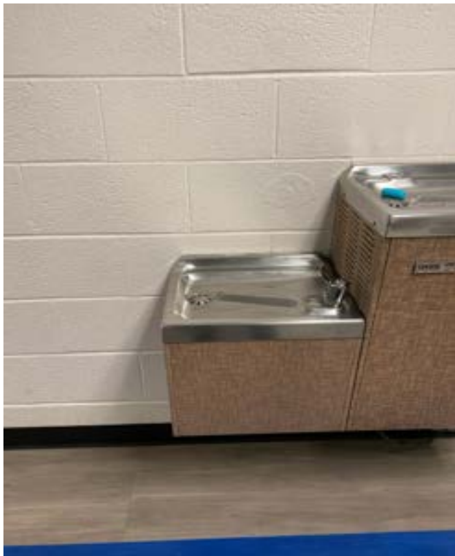
1/11/2024 - 7333-57 - Linden West Elementary - Outside Room 7-Left
