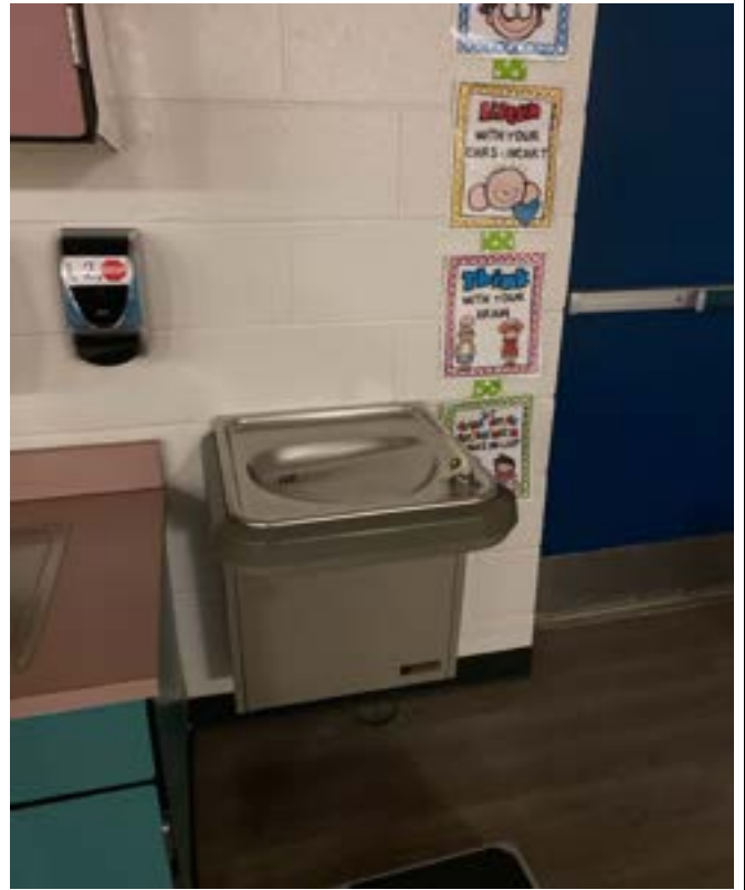
1/11/2024 - 7333-66 - Linden West Elementary - Room 1
