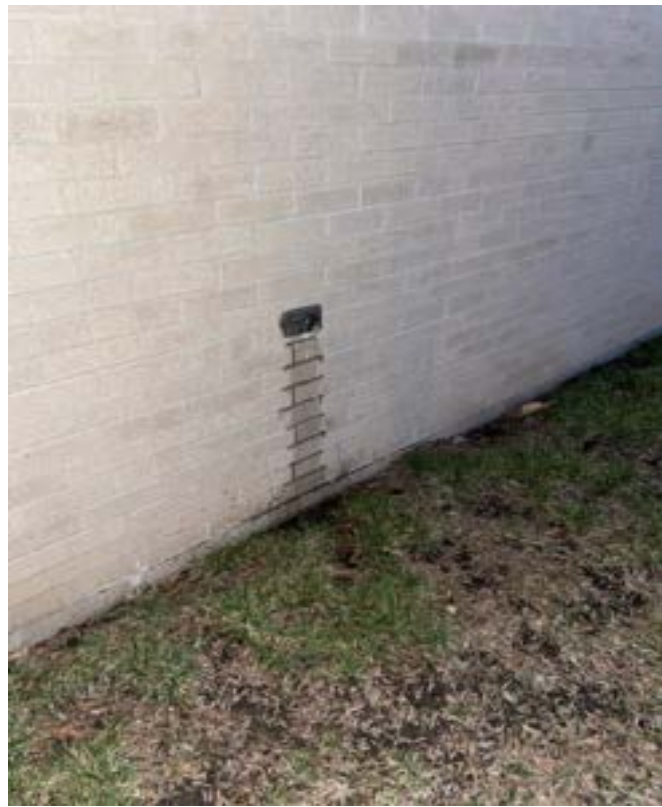
1/5/2024 - 5125-73 - Gracemor Elementary - South of Exit Door 1
