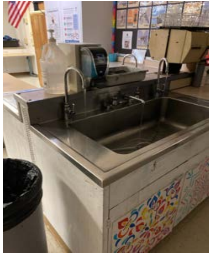
12/29/2023 - 4700-26 - Eastgate - Room 226- West-Left
