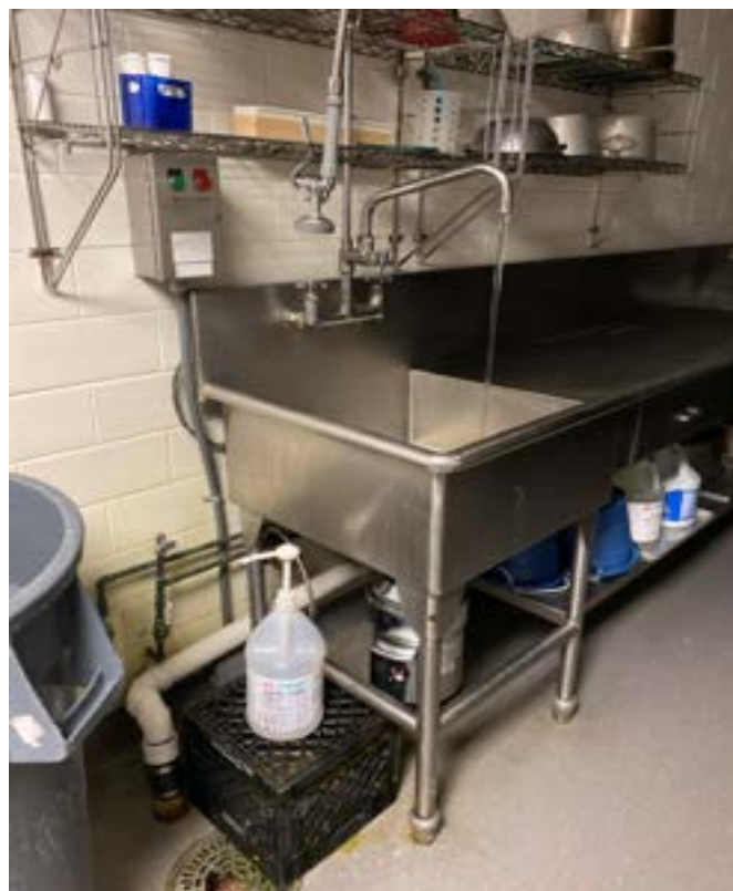
12/29/2023 - 4700-47 - Eastgate - Kitchen-East Wall-Far Left
