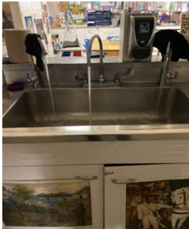
12/29/2023 - 4700-17 - Eastgate - Room 223- West-Left
