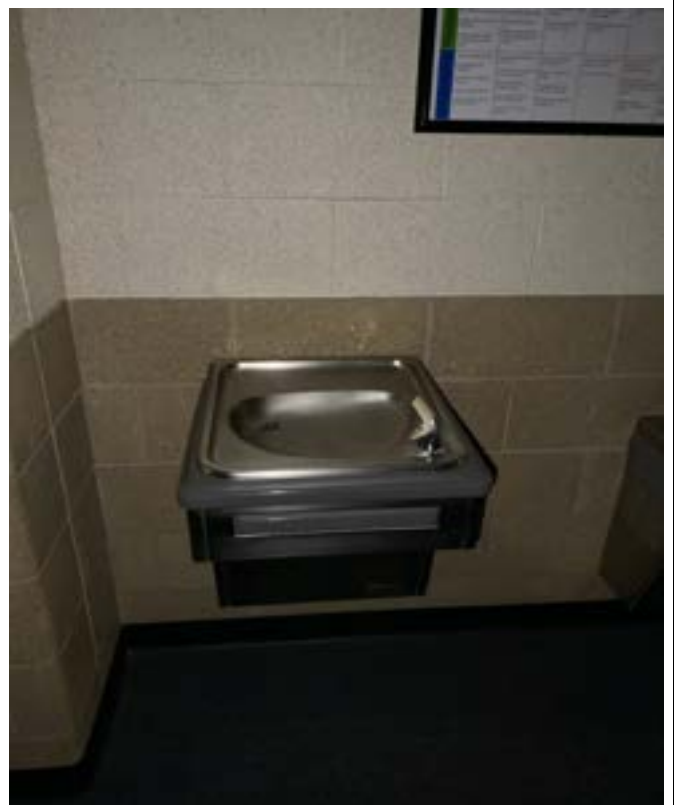
1/16/2024 - 9201-68 - Gateway Middle School - Outside 800 Hallway-Left
