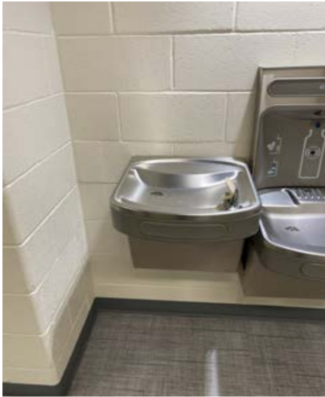
1/16/2024 - 9201-73 - Gateway Middle School - Outside Jumbo Gym-Far Left
